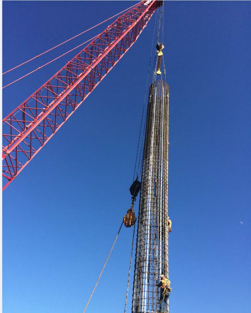
Aviation Century Aerial Structure – CIDH Rebar Cage.
