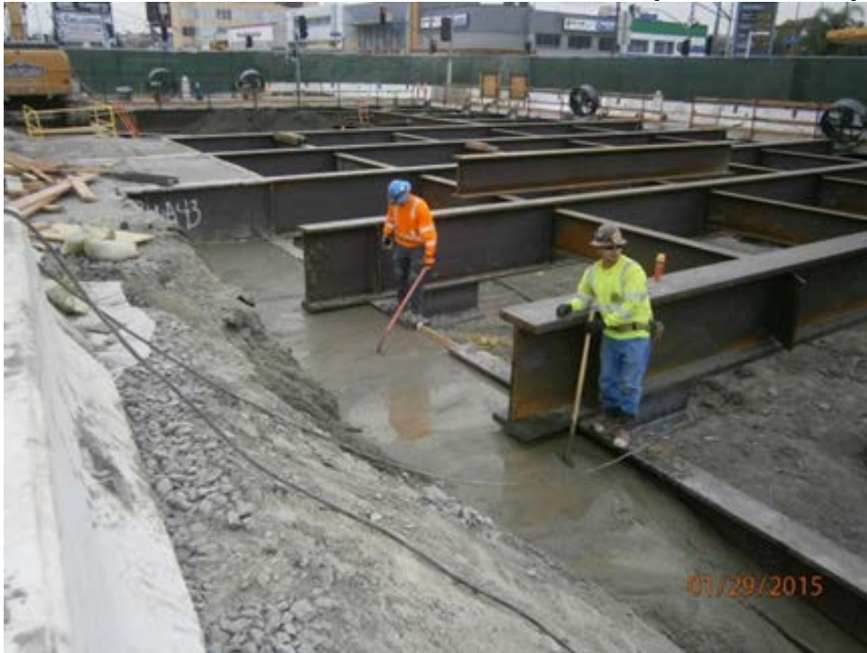
Slurry backfill behind lagging N/E end of Expo Station.
