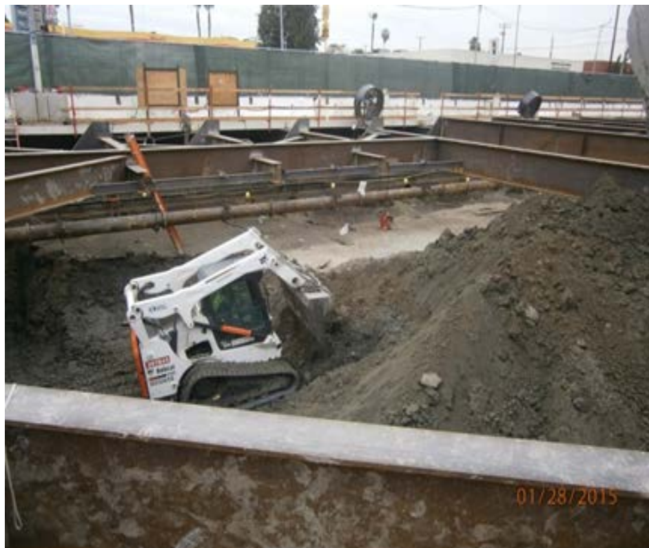
Moving soil in muck shaft.
