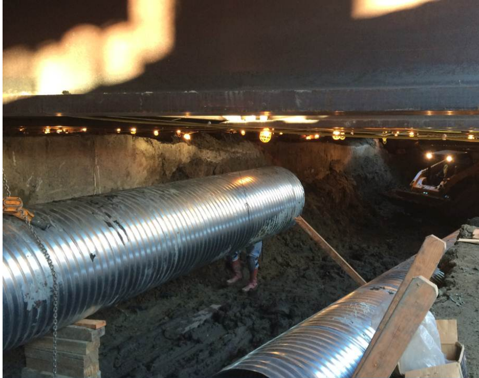
Expo Station Decking – Temporary Storm Drain.
