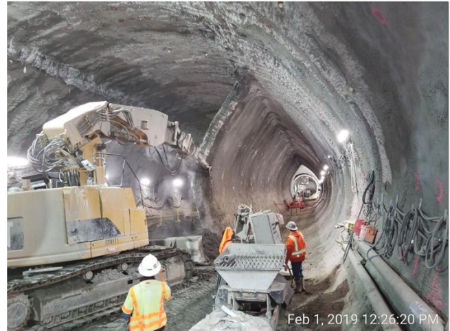
Right center wall demolition of SEM Cavern
