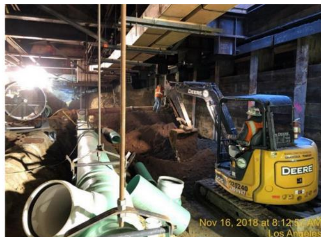
Preparations for sewer bypass under Flower St
