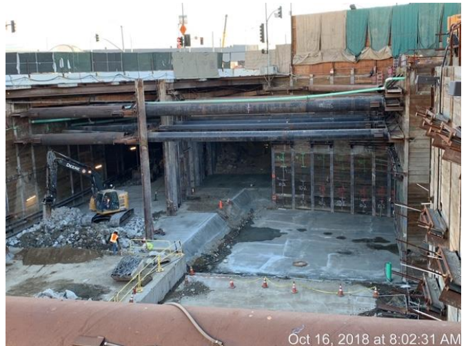
Installation of mud slab at track level in the future Little Tokyo/Arts District Station
