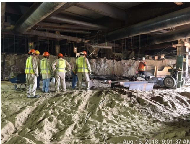
DWP onsite to patch duct bank at Wye and 1 st Street
