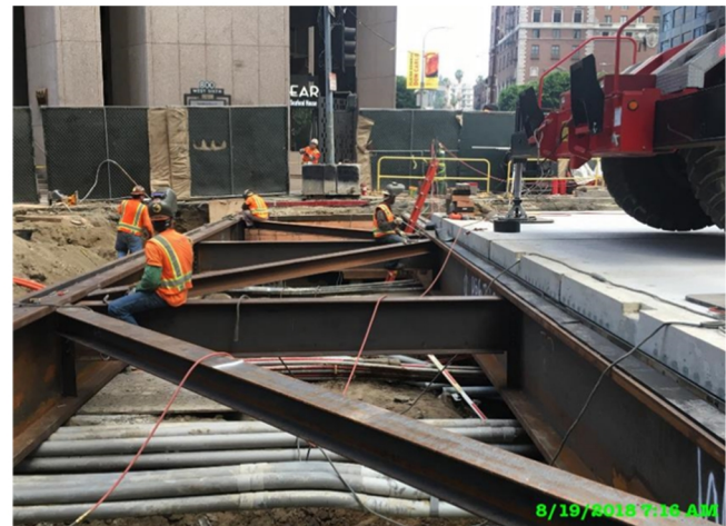
Welding deck beams on Flower St
