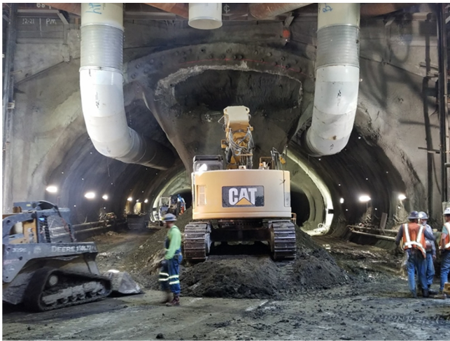
Excavation of SEM Cavern upper center drift
