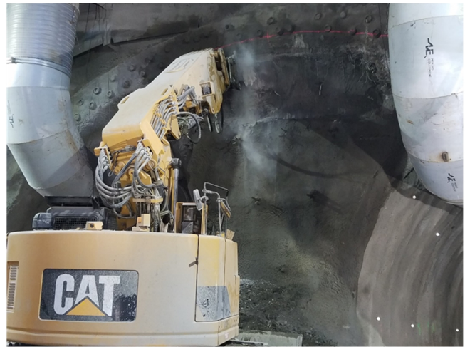
Excavation of SEM Cavern upper center drift
