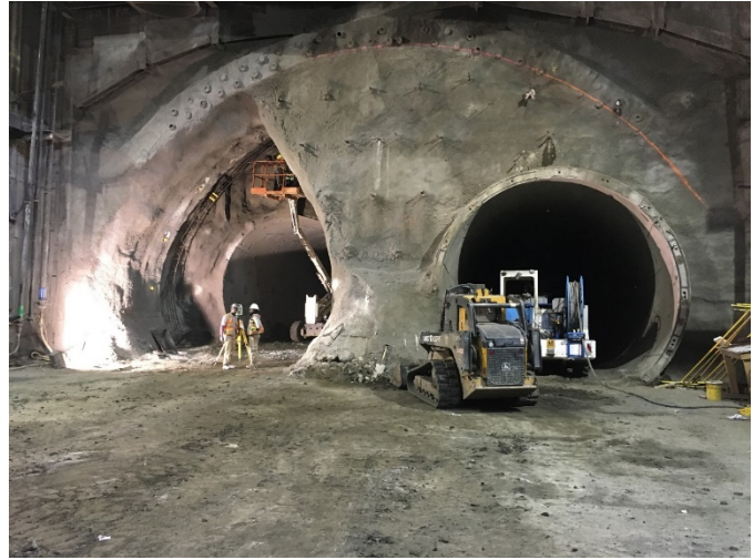
SEM mining for crossover cavern at Historic Broadway Station
