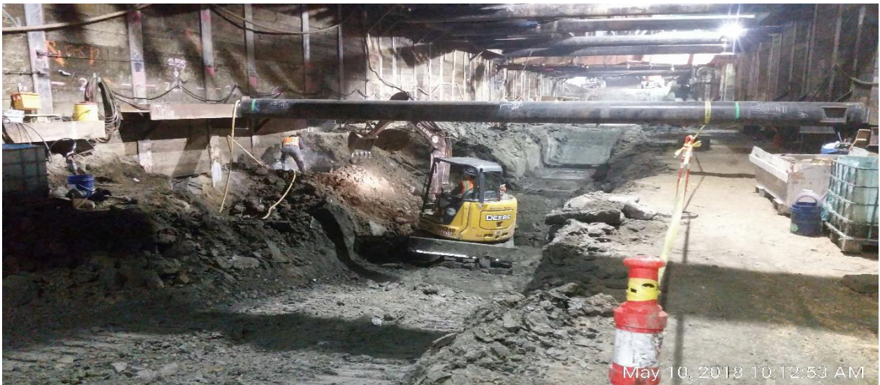
Excavation and lagging under Flower Street
