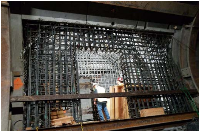
Cross Passage construction underway
