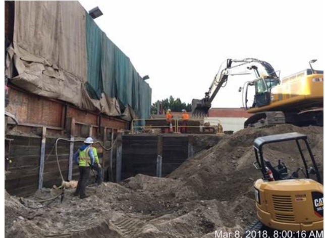
Excavation for Central Station and Wye
