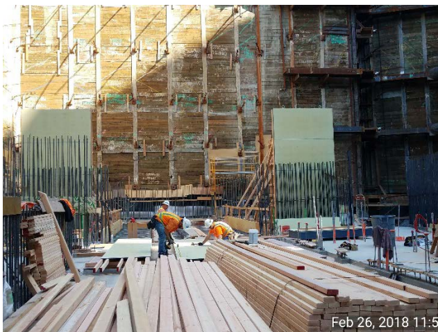
Grand Av Arts/Bunker Hill Station elevator shaft wall forms
