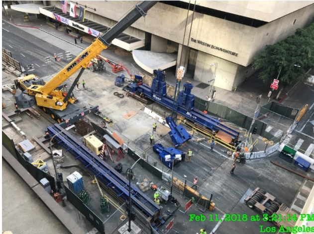
Gantry Crane demobilization
