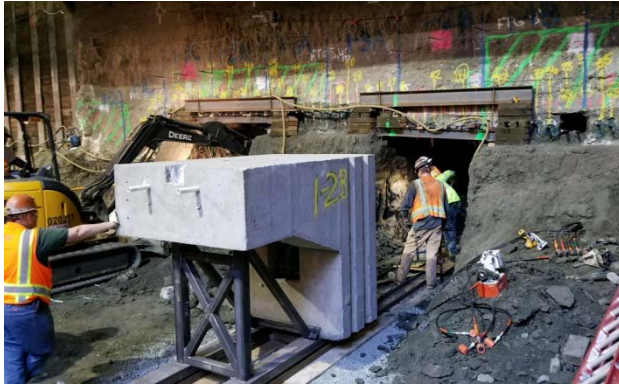
Underpinning activities underway
