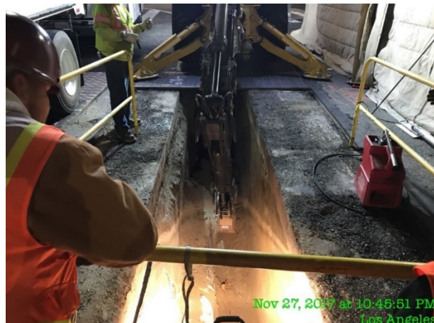
Excavation for Mainline B
