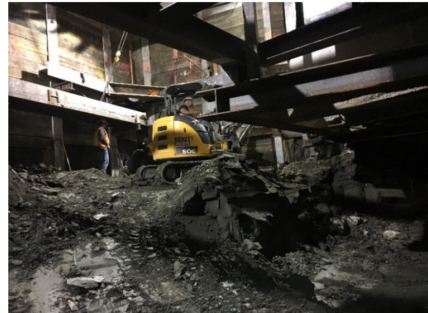
Excavation under Flower Street
