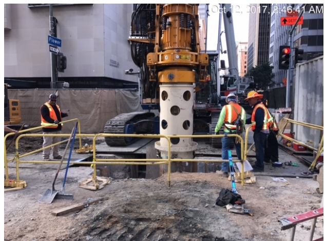
Pile installation on east side at 6th/Flower
