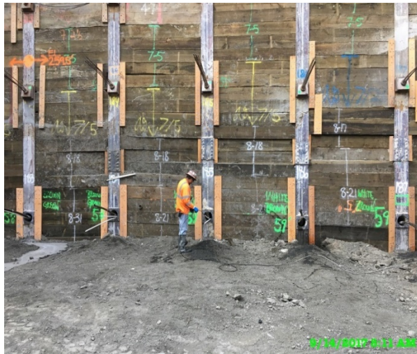
Grouting tie-backs at Level 3 Wall F
