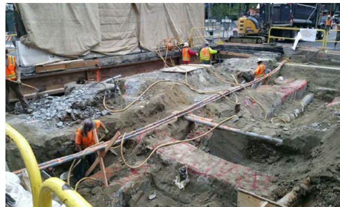
Excavation in preparation for deck beam installation
