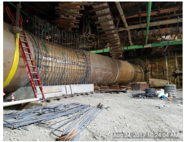
Hobas rebar cage forming at Historic Broadway
