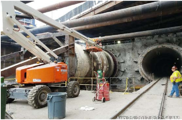
Welding TBM Shield in preparation for re-launch
