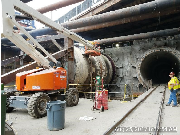
Welding TBM Shield in preparation for re-launch
