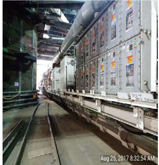
TBM trailing gear walked back to Central Station
