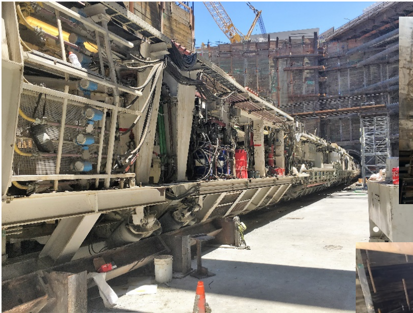
TBM in Grand Av Arts/Bunker Hill Station
