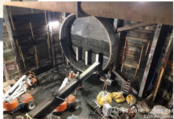
Installing fiberglass rebar at tunnel eye
