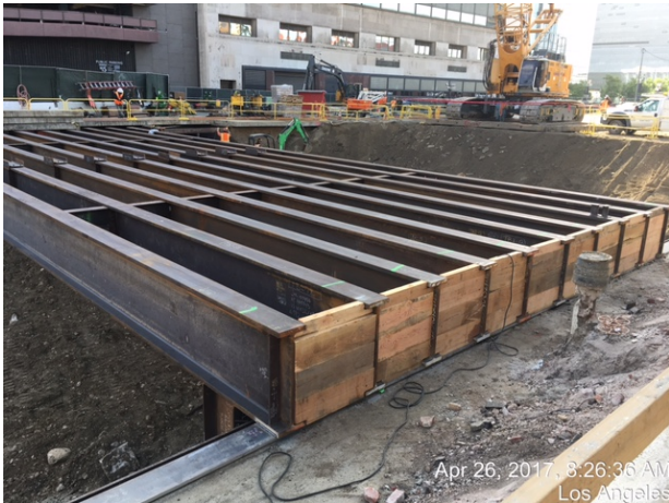
Installation of Trestle Beams at Broadway Station
