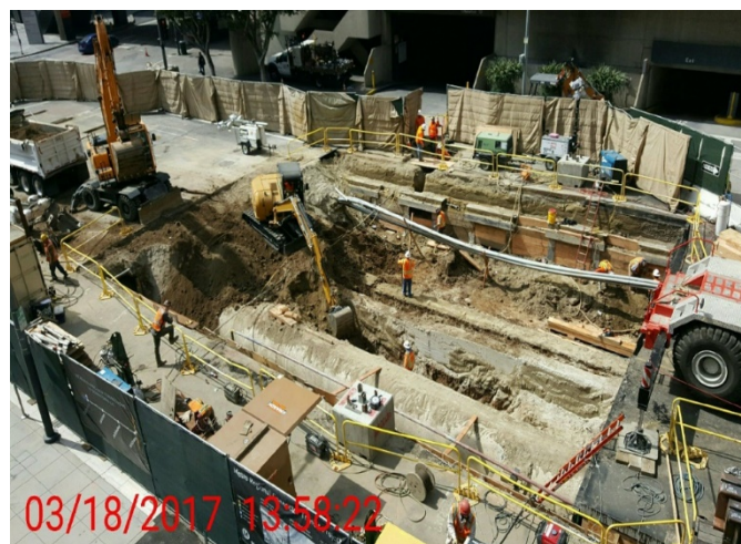
Excavation for deck beam installation over weekend closure
