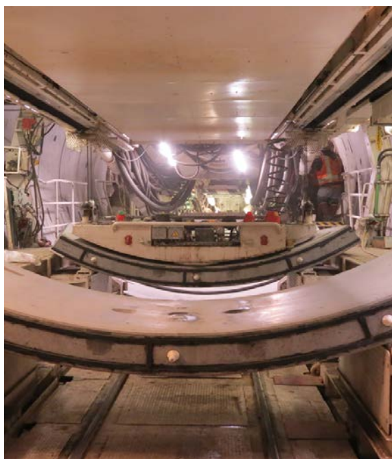
Concrete tunnel segments prepped for installation
