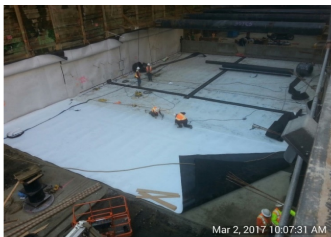
HDPE Installation at 2nd/Hope Station
