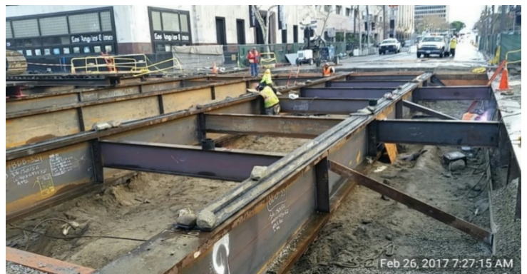
Decking at the 2nd/Spring Intersection
