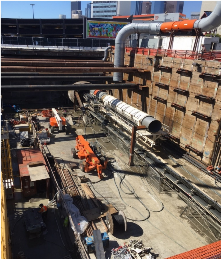
Tunneling operations underway
