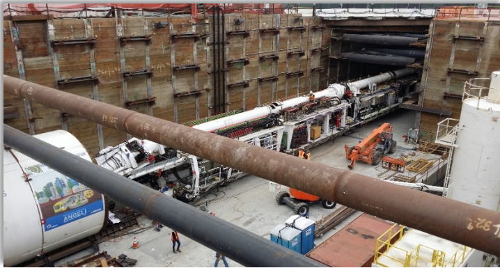
TBM assembly underway at 1st/Central Station
