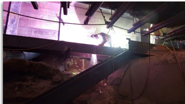
Welding of walers under Flower Street decking
