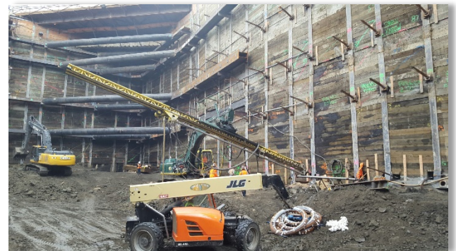
Drilling for tie-backs at 2nd/Hope Station
