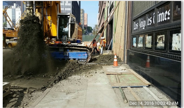
Piling on 2nd Street
