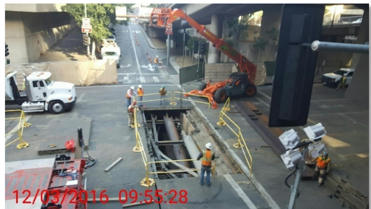
Lowering walers (support of excavation) at 4th/Flower
