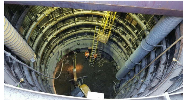
Tie-back removal shaft excavation
