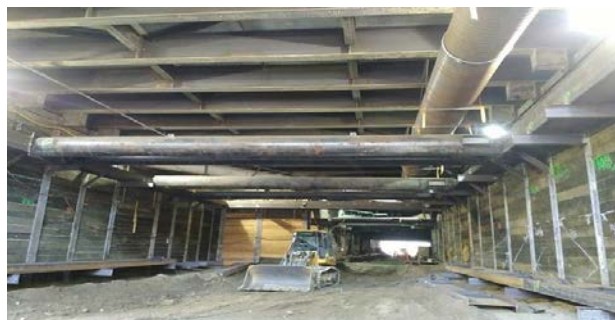
Continued excavation at Wye
