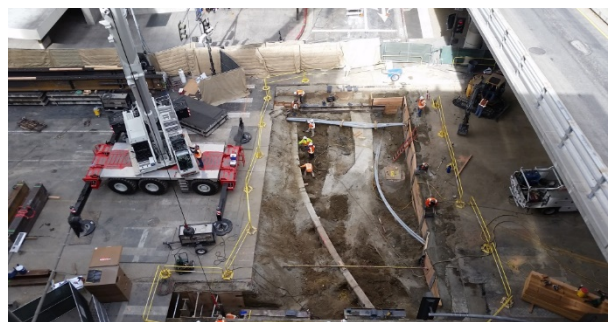
Decking preparations at 4 th /Flower Intersection
