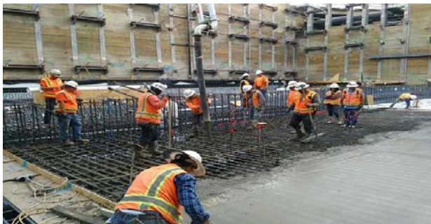
Concrete pours of invert slab
