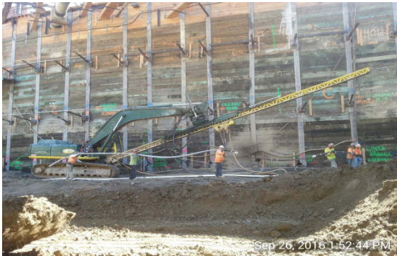
Tie-back installation at 2 nd /Hope
