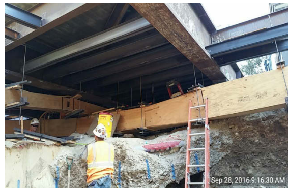
Utility hanging at 2 nd /Broadway
