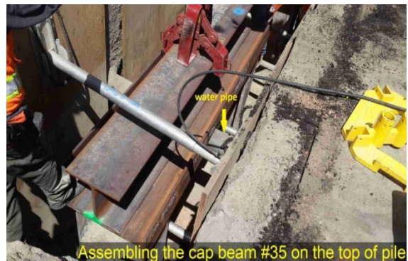
Cap beam installation on Flower Street
