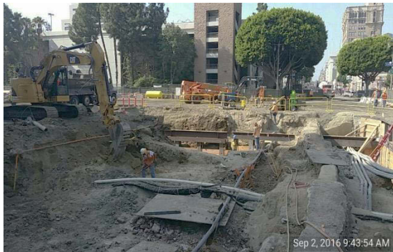
Deck beam installation at 2 nd /Broadway intersection
