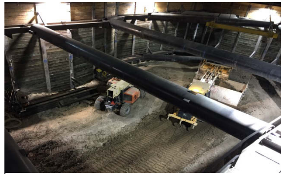
Excavation at 2 nd /Hope Station
