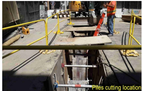
Pile related work on Flower Street
