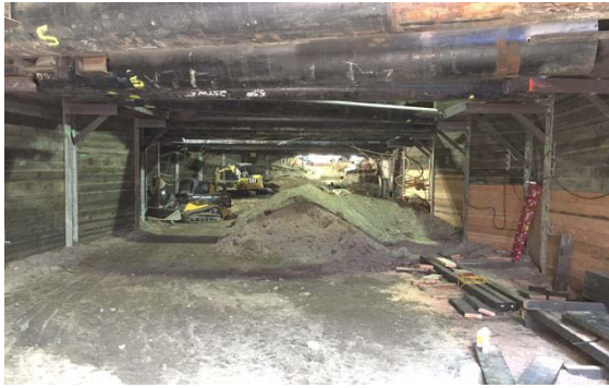
Excavation at Alameda Wye
