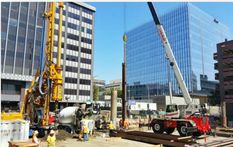
Piling at 2 nd /Broadway Intersection
