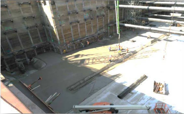
Pouring mud mat at 1 st /Central Station
