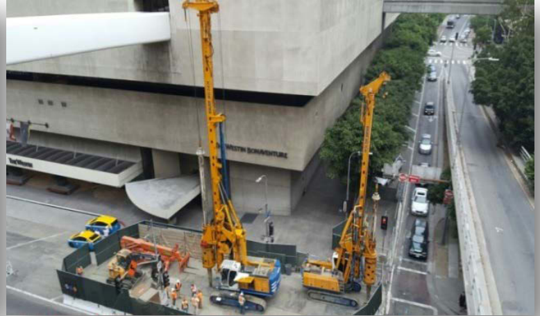
Piling setup at 4 th /Flower
