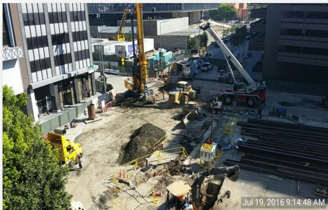
Piling at 2nd/Broadway Hammer Head
