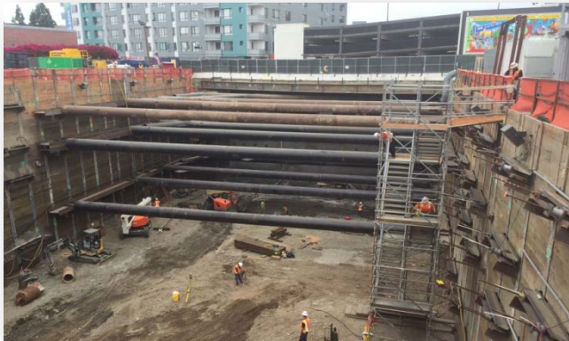
1st/Central Station Excavation
