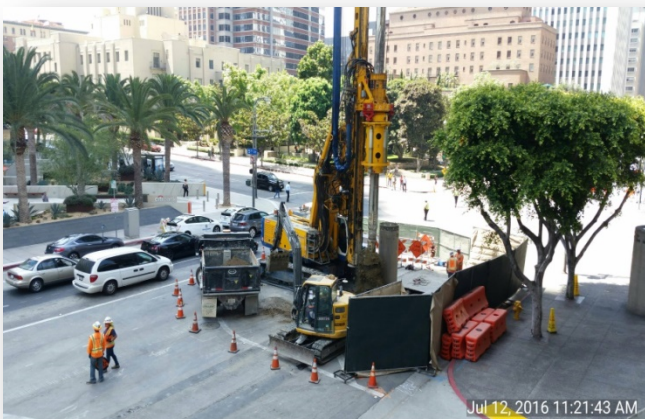
Piling on west side 5th/Flower Street
