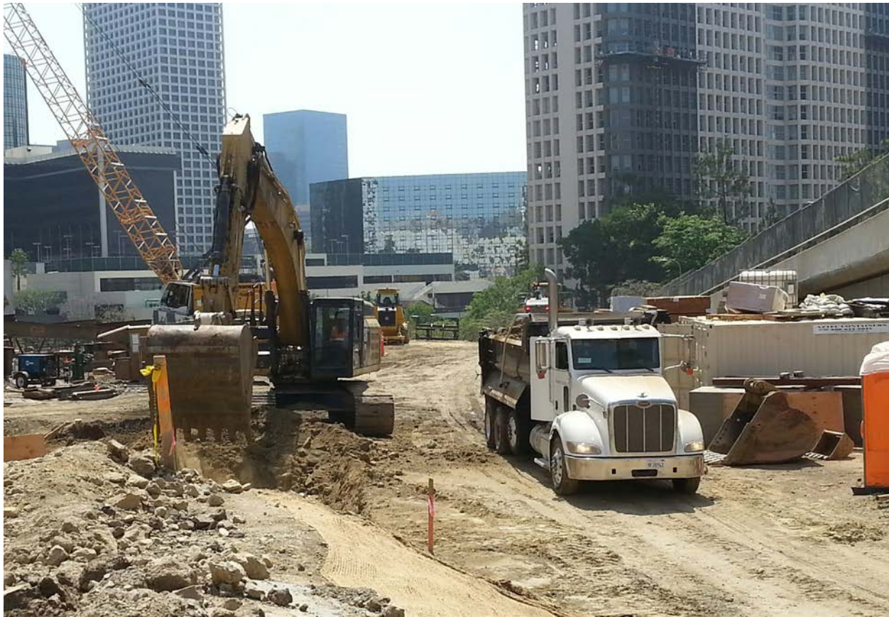
2 nd /Hope construction activities
