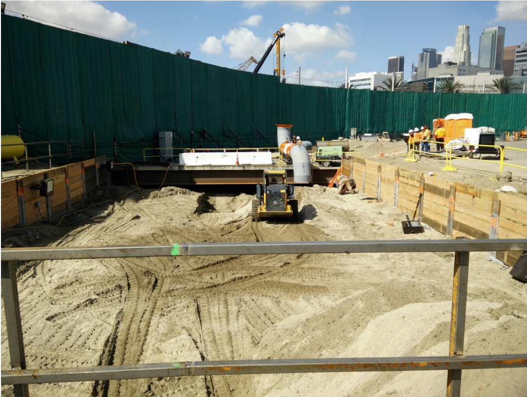
TBM Pit/Wye Excavation
