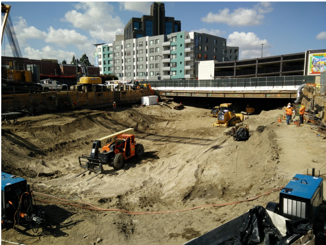
1 st /Central Station construction activities
