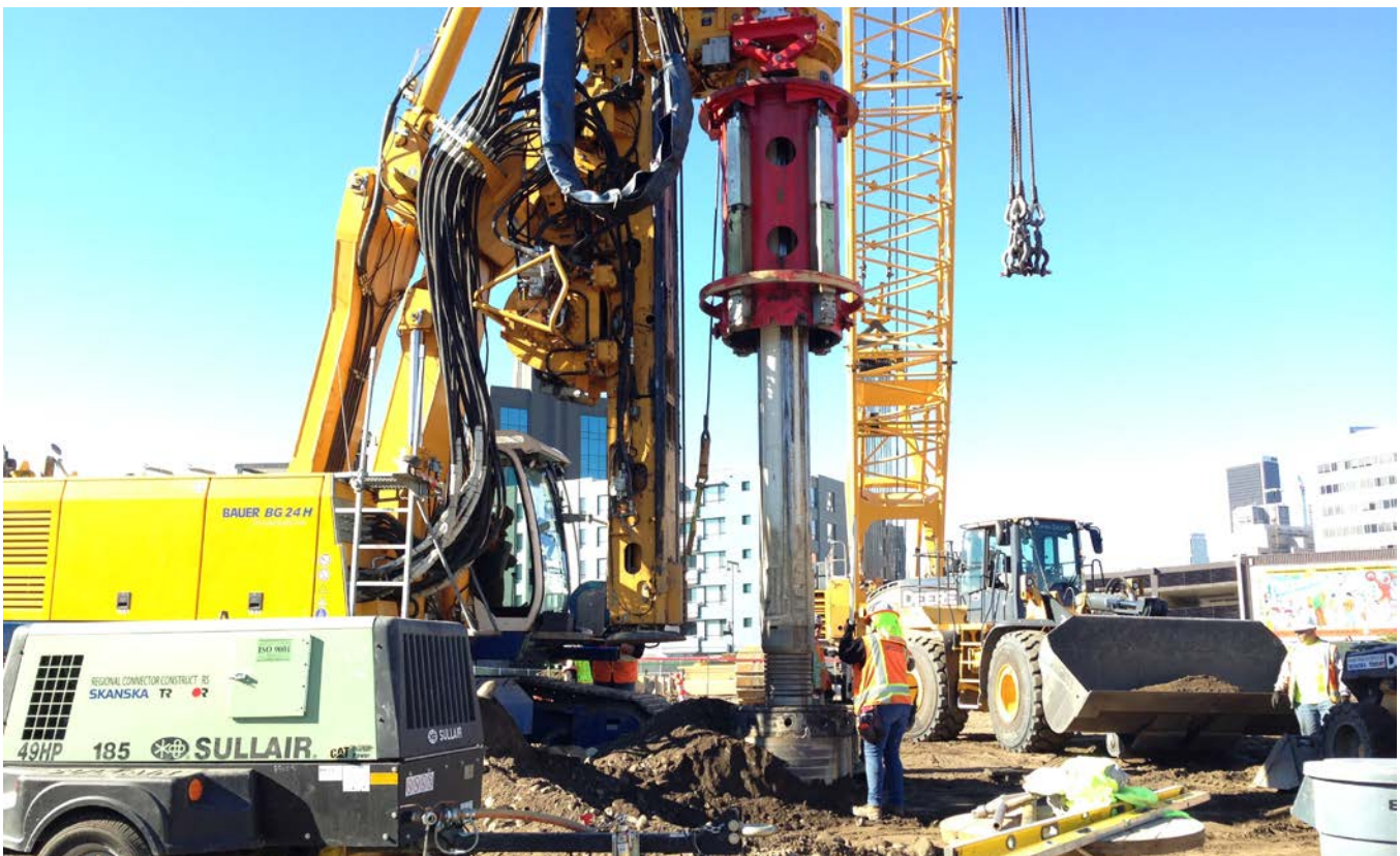
Pile installation at 1 st /Central Station
