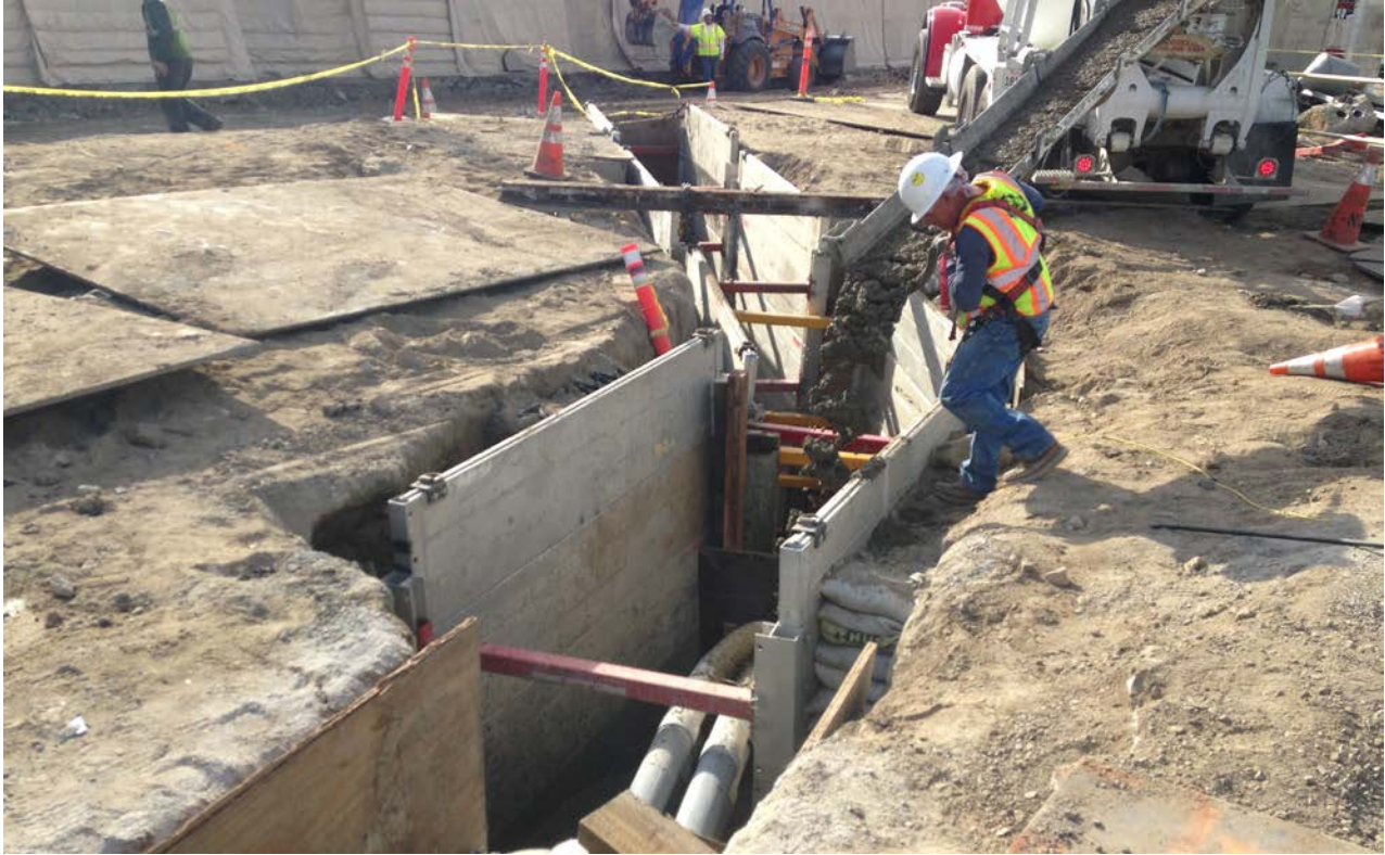
Backfill ductbank at 1 st /Hewitt
