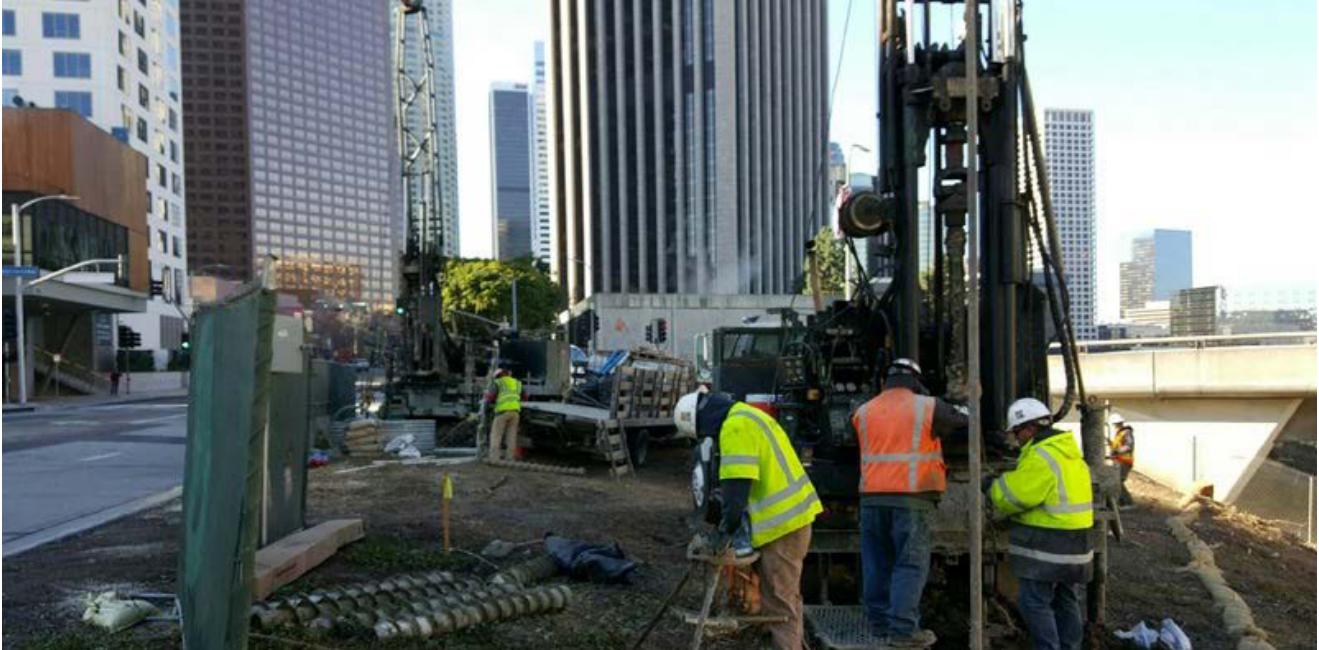
Installing Inclinometer at 2 nd /Hope
