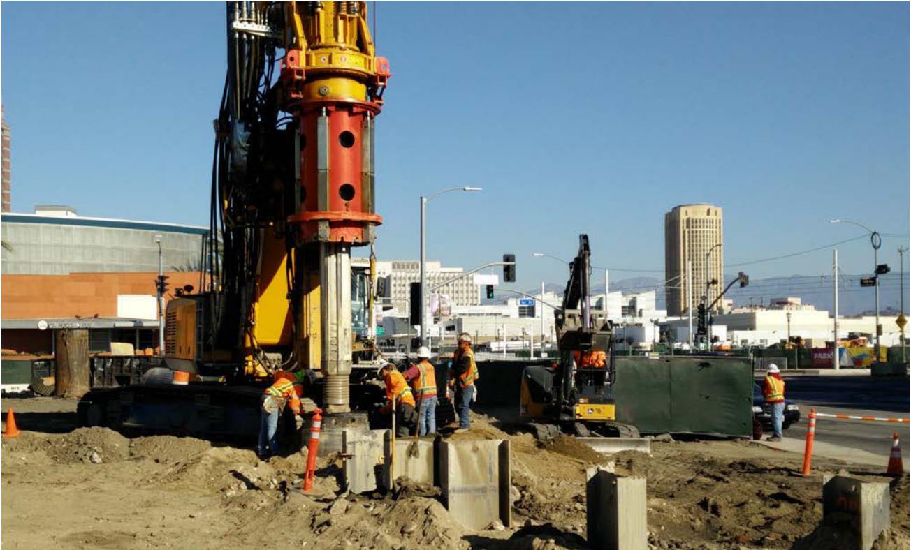
1 st /Central Pile Installation
