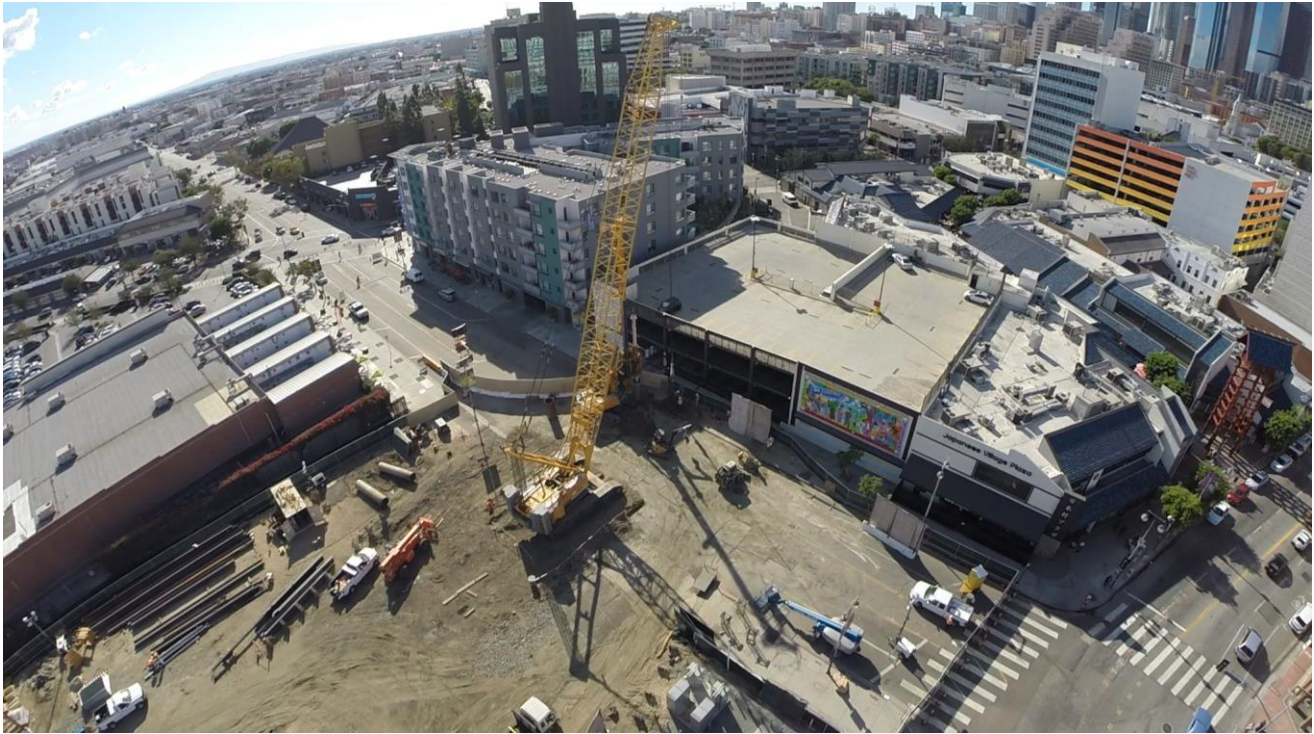
1 st /Central Construction Activities
