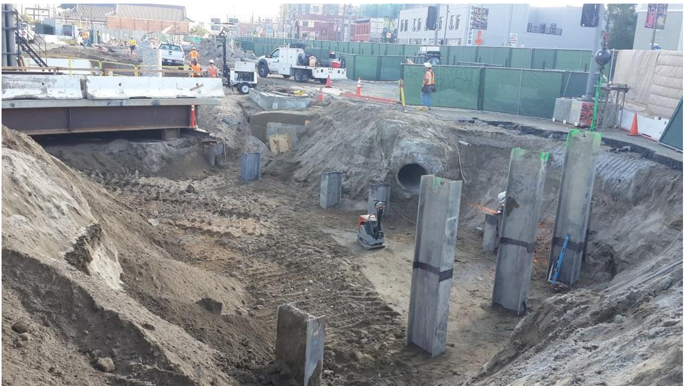
Excavation and pile installation at Mangrove Yard
