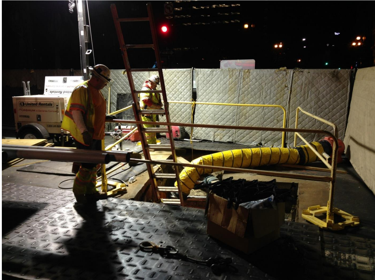
Nighttime electrical work at 2 nd /Spring
