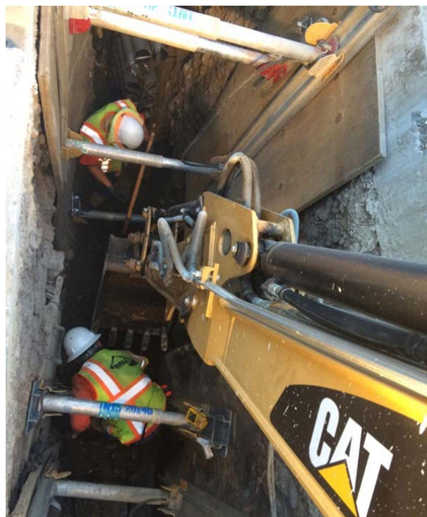
Trench Excavation at Broadway St.
