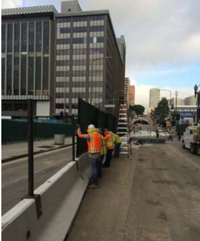
2 nd St. closure – Installing fence panels
