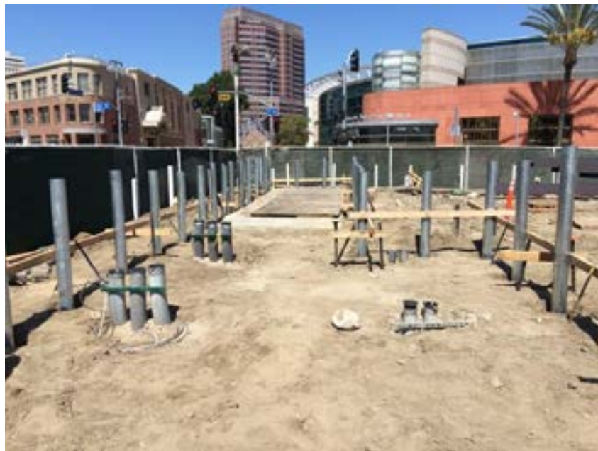
Bollards set up at 1 st and Central
