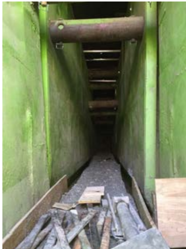
1 st /Rose – Stripping Encasement
