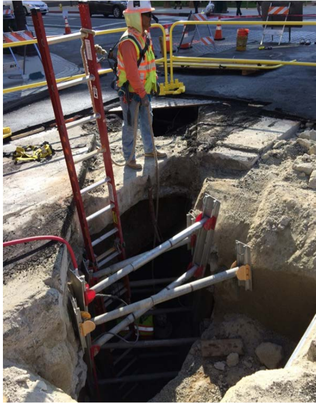
2 nd /Broadway trenching and shoring
