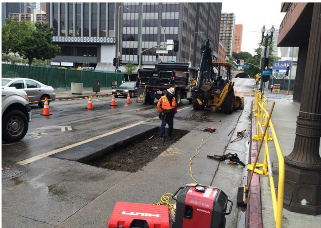
C0980 Contract – Pile Trenching on 2 nd Street
