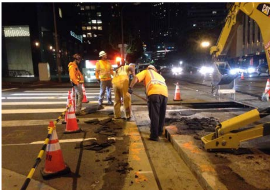
C0980 Contact – Trench/Pothole pave at Flower St.
