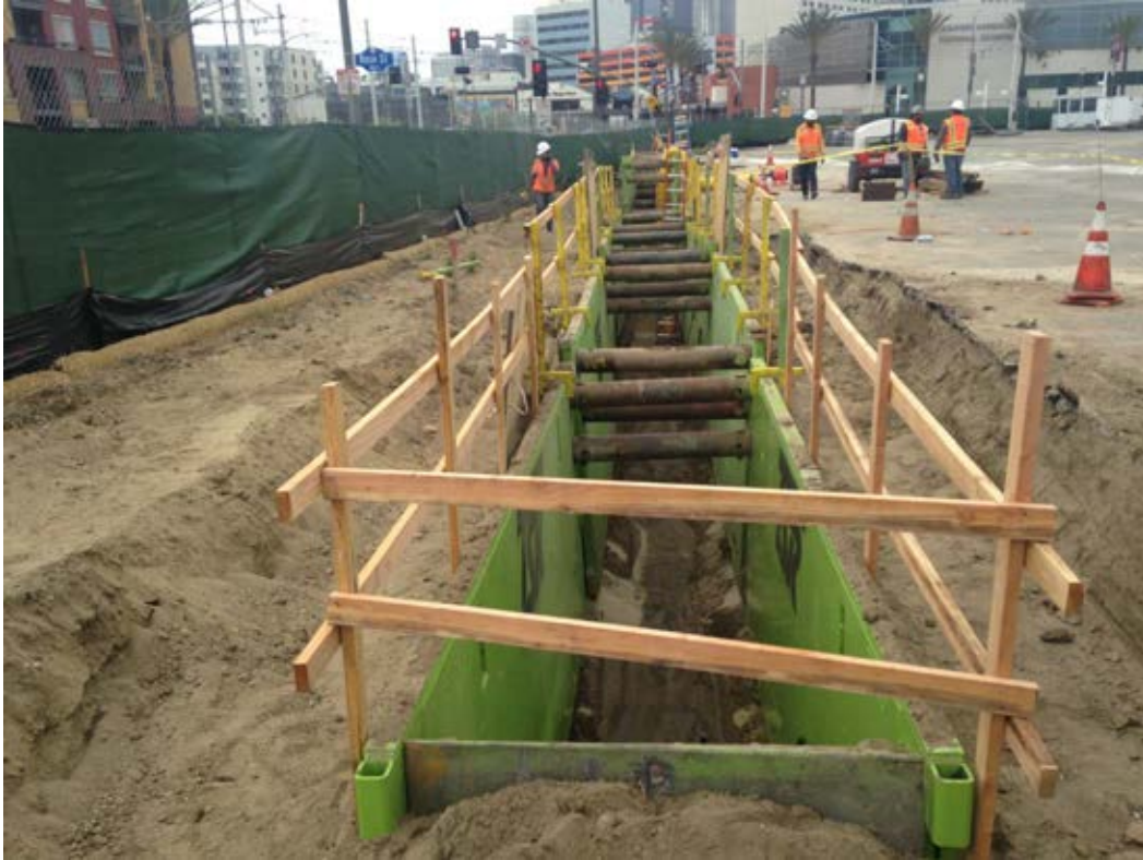
C0980 Contract – Storm Drain at Mangrove yard
