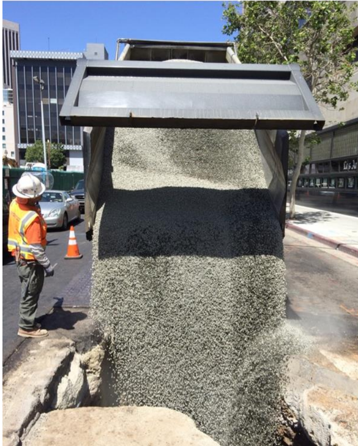
C0980 Contract - Backfilling main line at 2 nd /Spring Sts.
