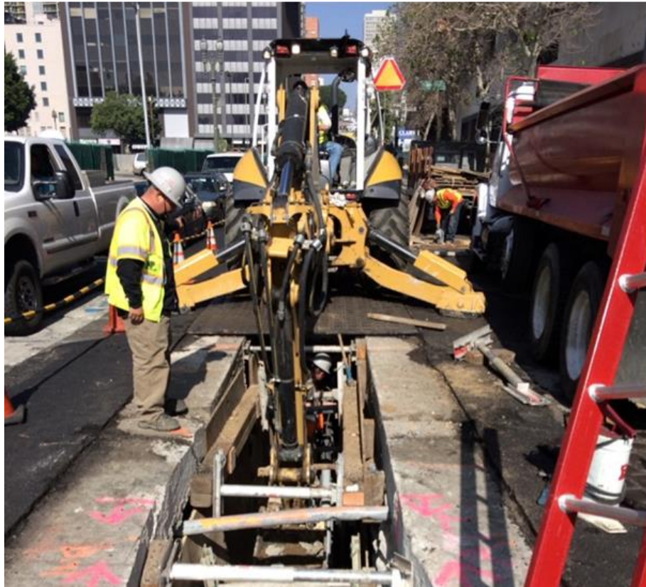
AUR C0981R – Lateral excavation at 2 nd St.
