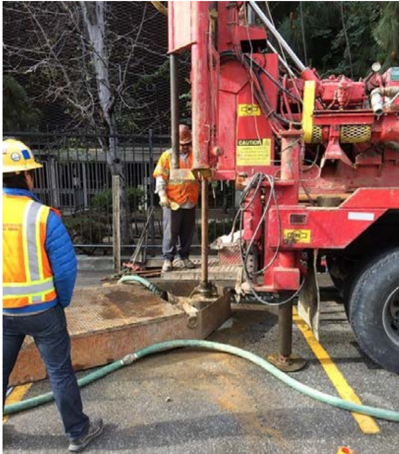
C0980 Contract – Well Shaft Construction at 2 nd /Spring Sts.
