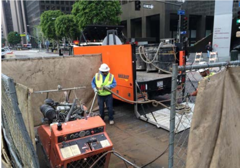
AUR C0981R – Saw cutting and potholing at 5 th and Flower Sts.
