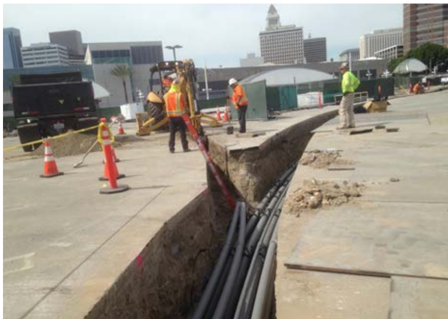
C0980 Contract – Mangrove Yard set up
