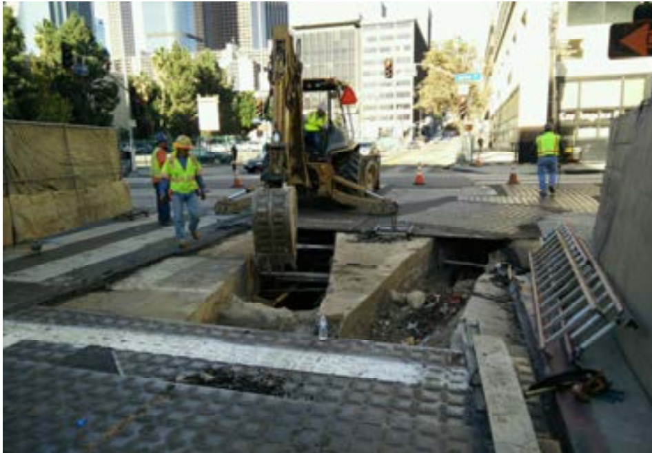
AUR C0981R - Excavation and Shoring at 2 nd and Broadway Sts.
