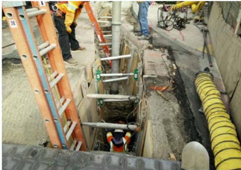
AUR C0981R – Electrical Excavation at 1 st and Alameda Sts.
