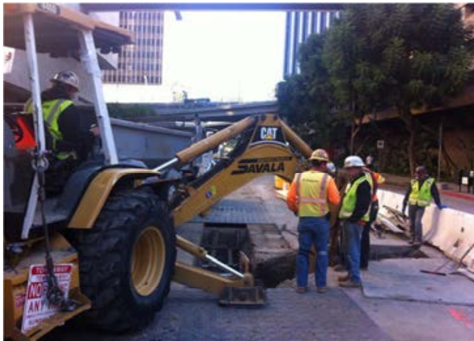
AUR C0981R – Excavation and Shoring at Flower St.
