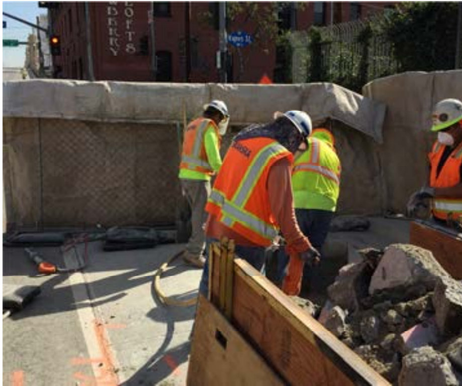
C0980 Contract – Potholing at 1 st and Vignes Sts.
