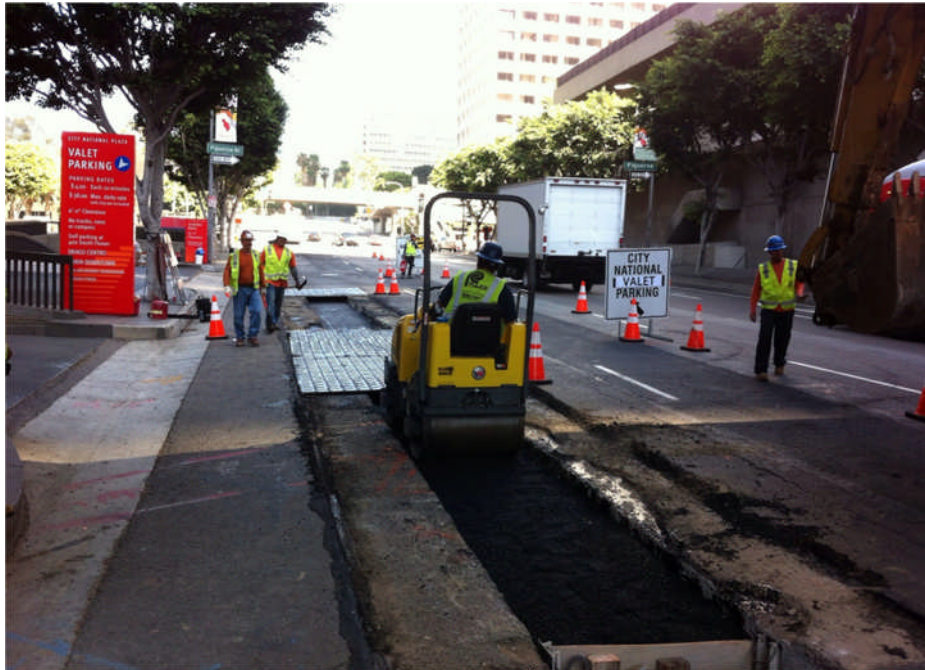
Placing asphalt base at 5 th St. west of Flower St.
