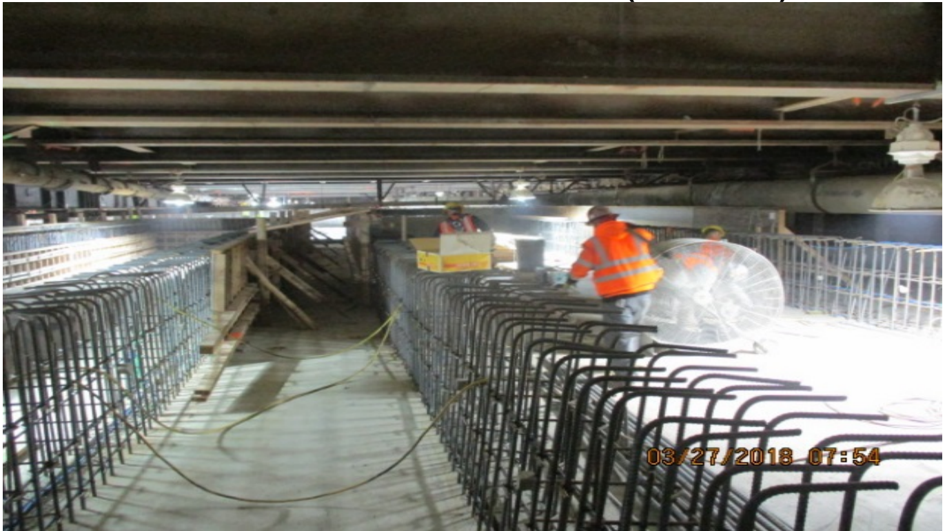
LEIMERT PARK STATION – Installation of formwork for roof plenum walls.
