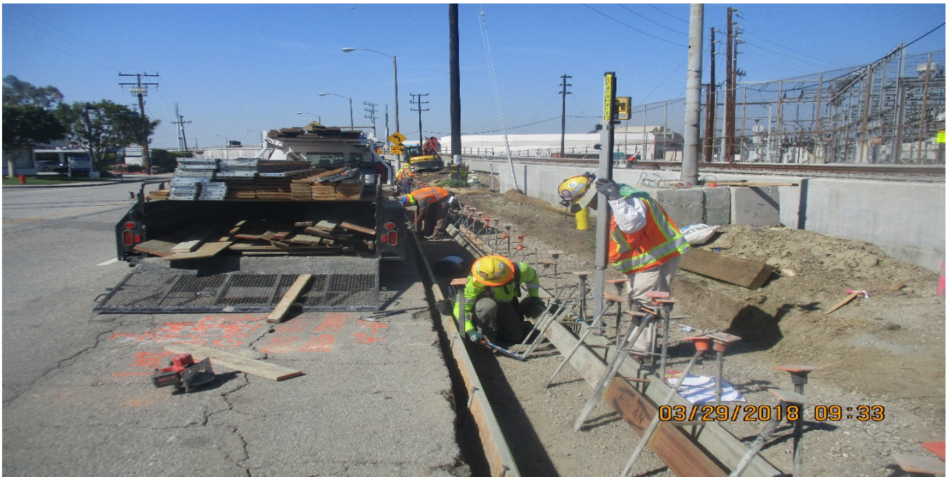
B1 GUIDEWAY - Placing curb & gutter on Florence close to Hillcrest.
