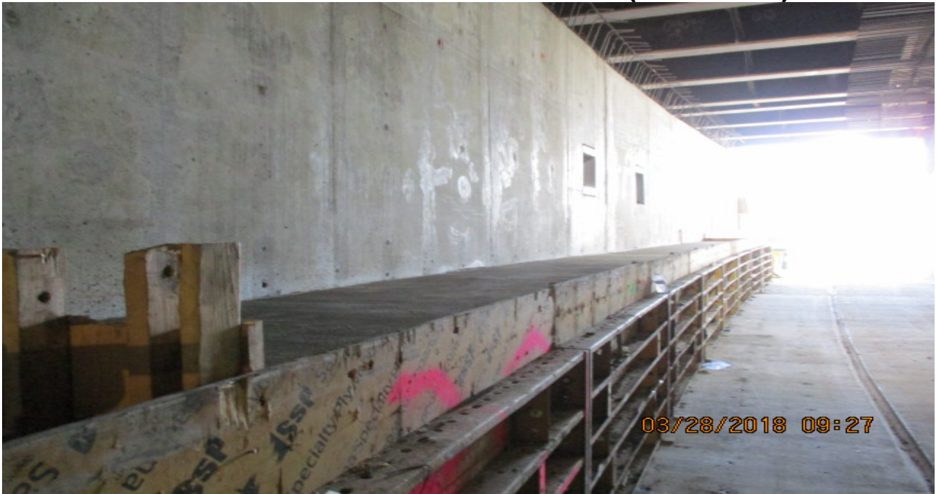
UG4 – Southbound walkway forms (pre-strip).
