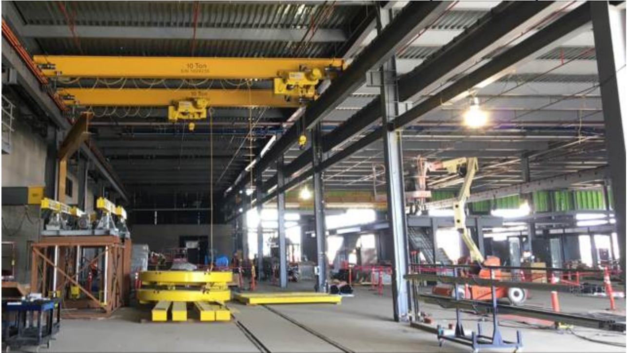
SOUTHWESTERN YARD – Main shop equipment turn tables, truck lift, 10 ton cranes.
