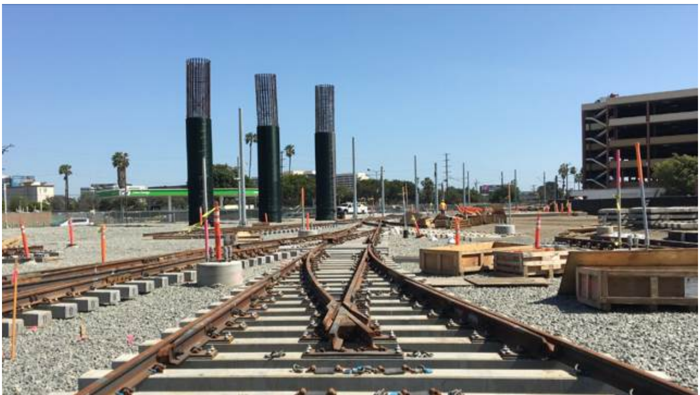
SOUTHWESTERN YARD – Looking south showing yard and automated people mover columns.
