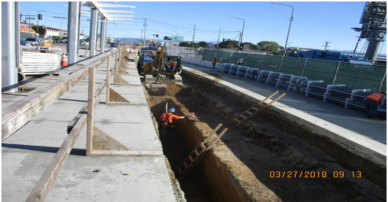
HYDE PARK STATION - Trenching for systems duct bank.
