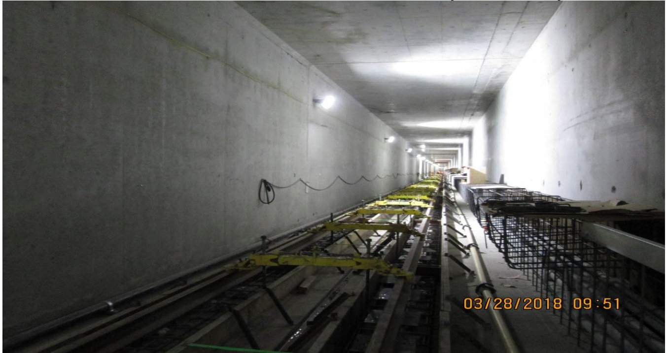
UG3 - Ironhorse direct fixation plinth construction alongside walkway reinforcement.
