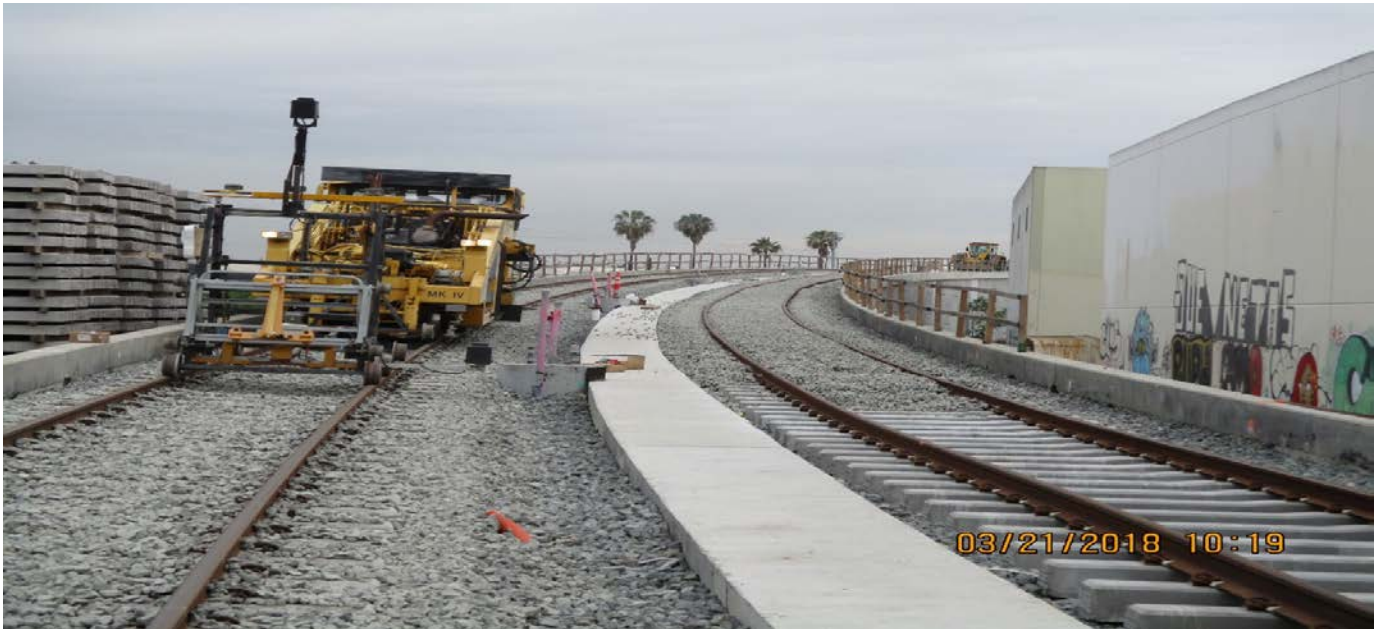
(AG-4) MANCHESTER BRIDGE – Tamping of SB track and flooding of ballast rock along NB track.
