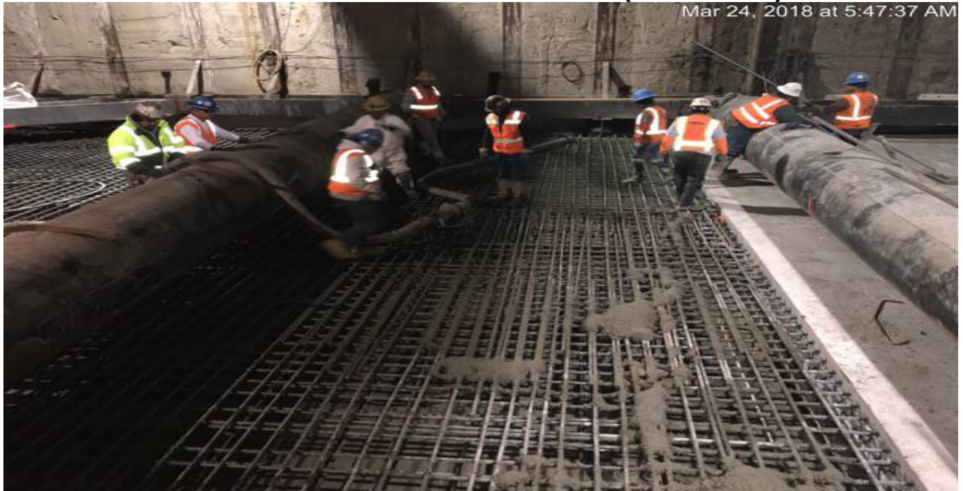
EXPOSITION/CRENSHAW STATION – Concrete placement at section F1 of Phase 4 Roof.
