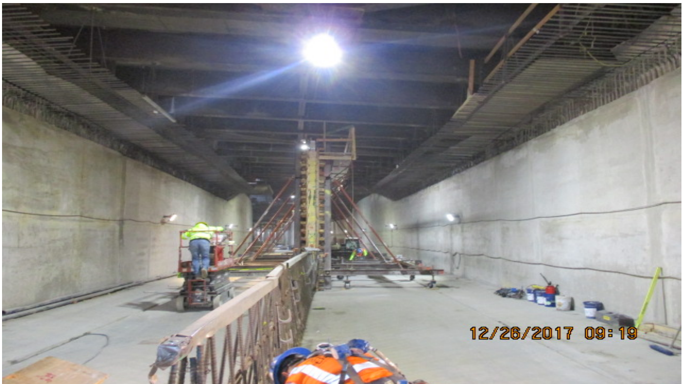
UG4 – Installation of formwork for center wall section CW-16.
