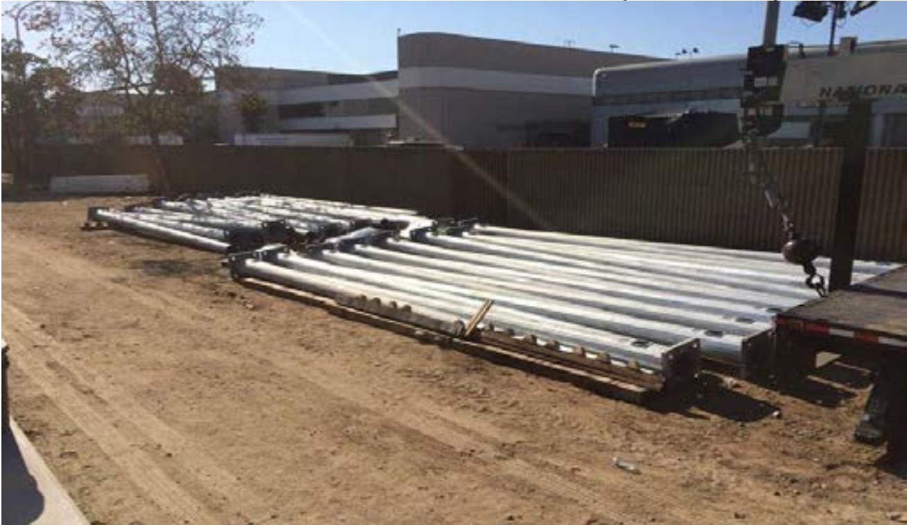
MSE 29L&R – OCS poles delivered and stock piled on the west side of the retaining wall.
