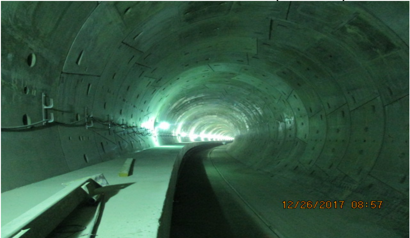
TUNNELING – NB Tunnel at Vernon portal.
