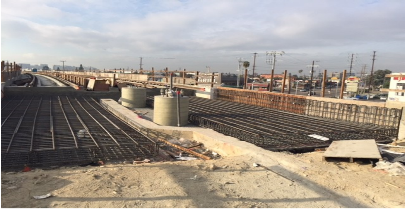
MANCHESTER BRIDGE - Abutment 3 approach slabs overview.
