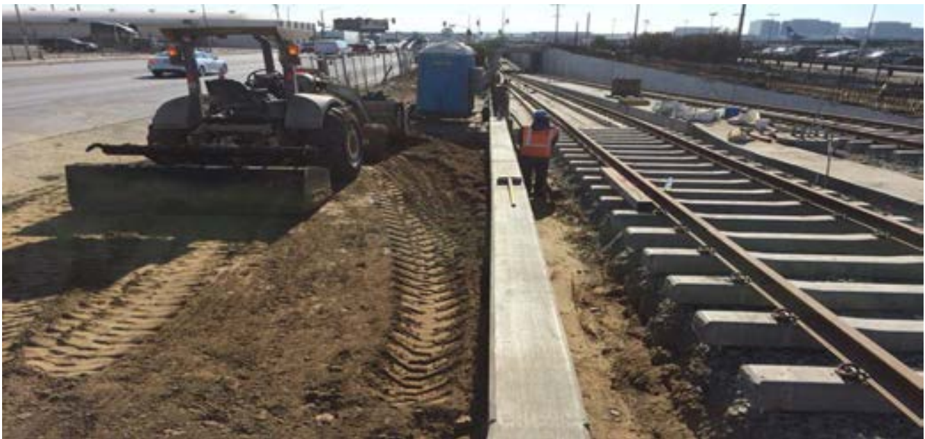
UG1 – Backfill and compaction on both sides of the retainer wall STA 59+50 to 60+00.
