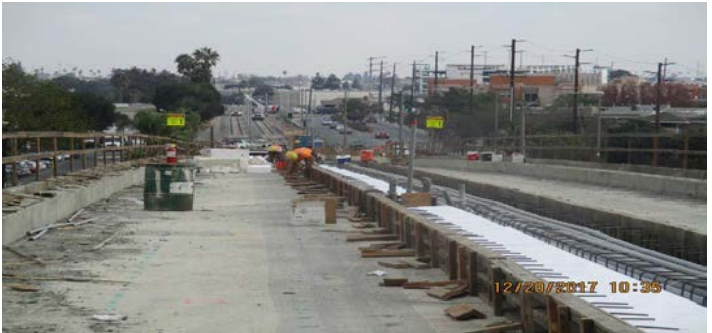
(AG-5) I-405 - Span 4 epoxied reinforcement doweling and bracing the north face of ductbank.
