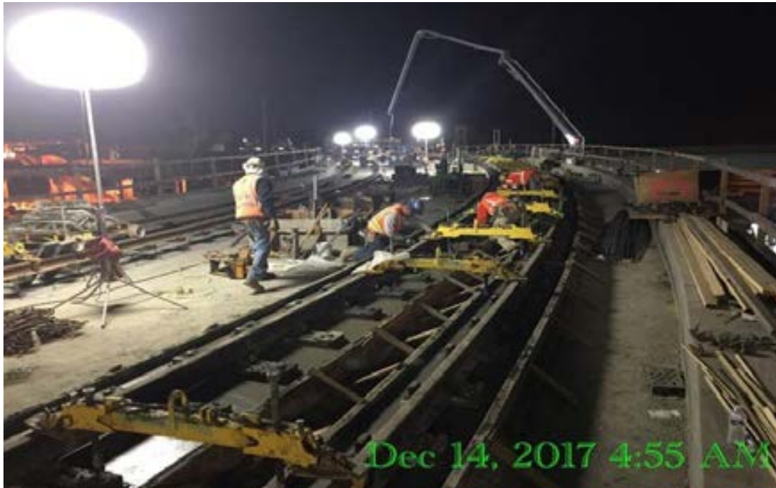
GREENLINE UNDERPASS – Crew finishing concrete plinth pour on track-3 SB.
