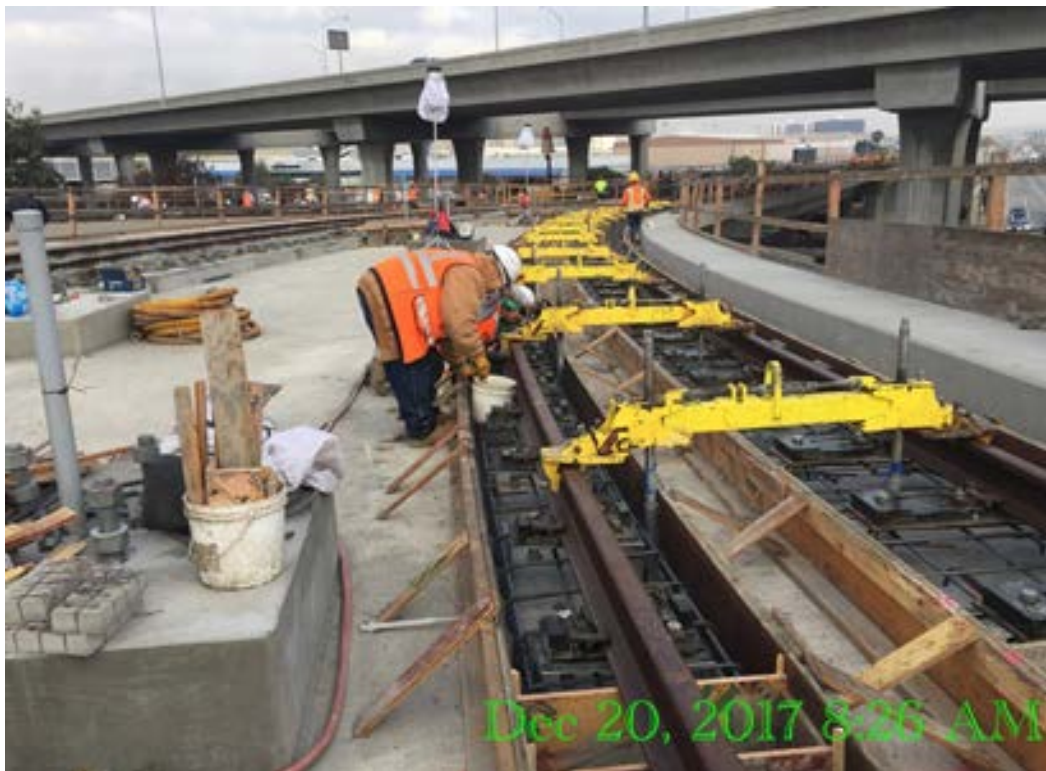
GREENLINE UNDERPASS – Crew continued installation of iron horse system and rail fasteners on track-4 NB.
