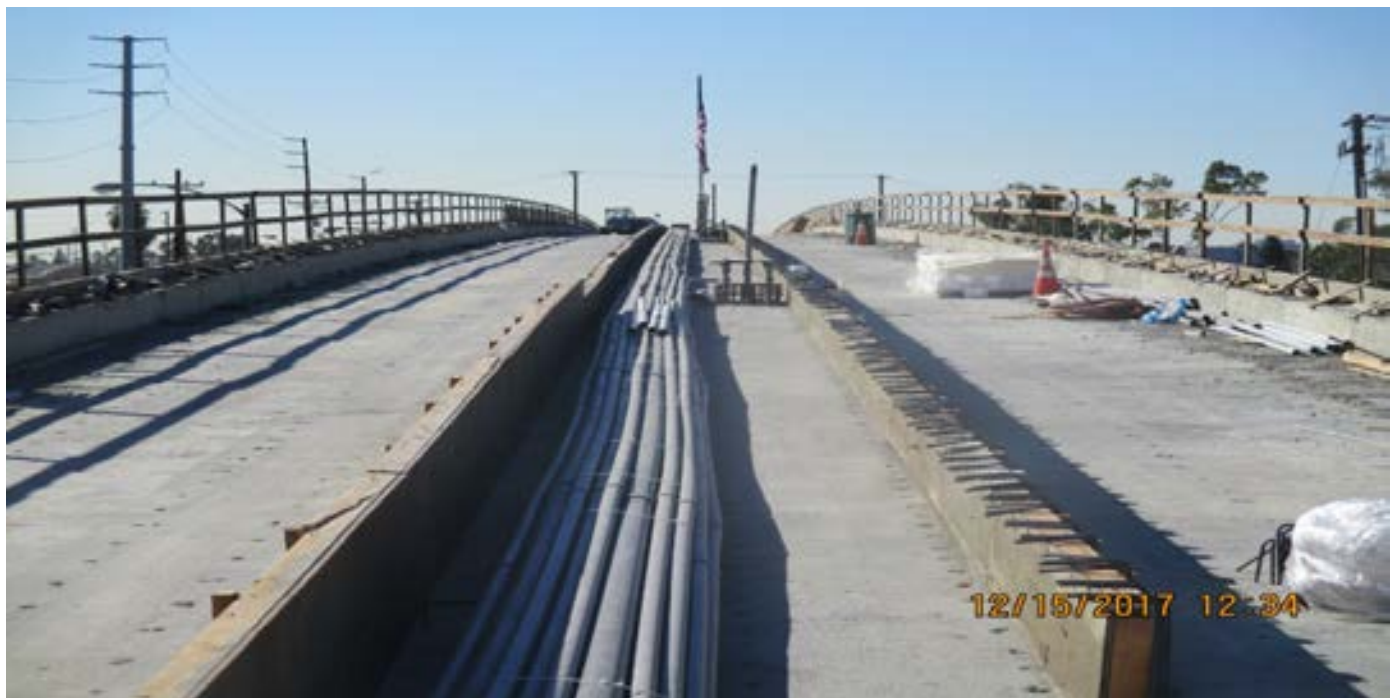
(AG-5) I-405 - Overview of electrical ductbank forming.
