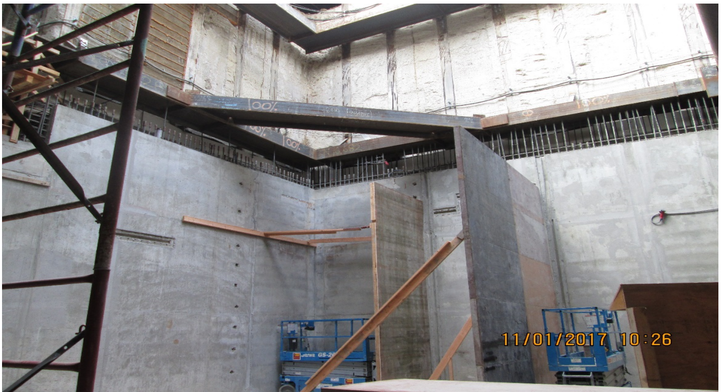
MARTIN LUTHER KING JR. STATION – Installing formwork for west interior walls.
