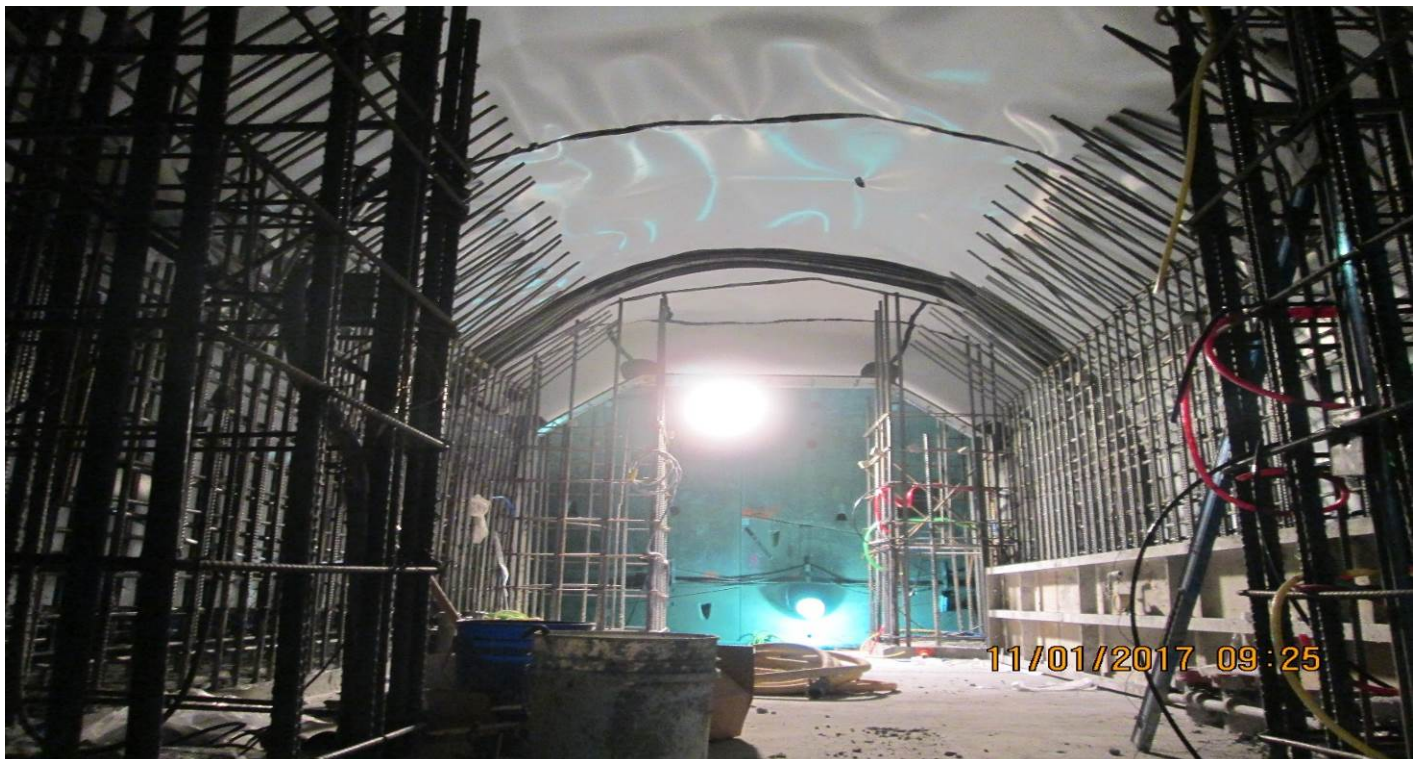
TUNNELING – Side and end wall rebar progress at CP-1.
