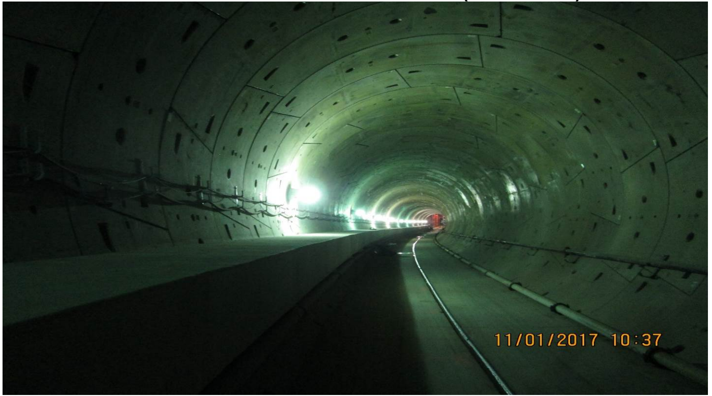
TUNNELING – NB Tunnel Walkway looking into MLK station.
