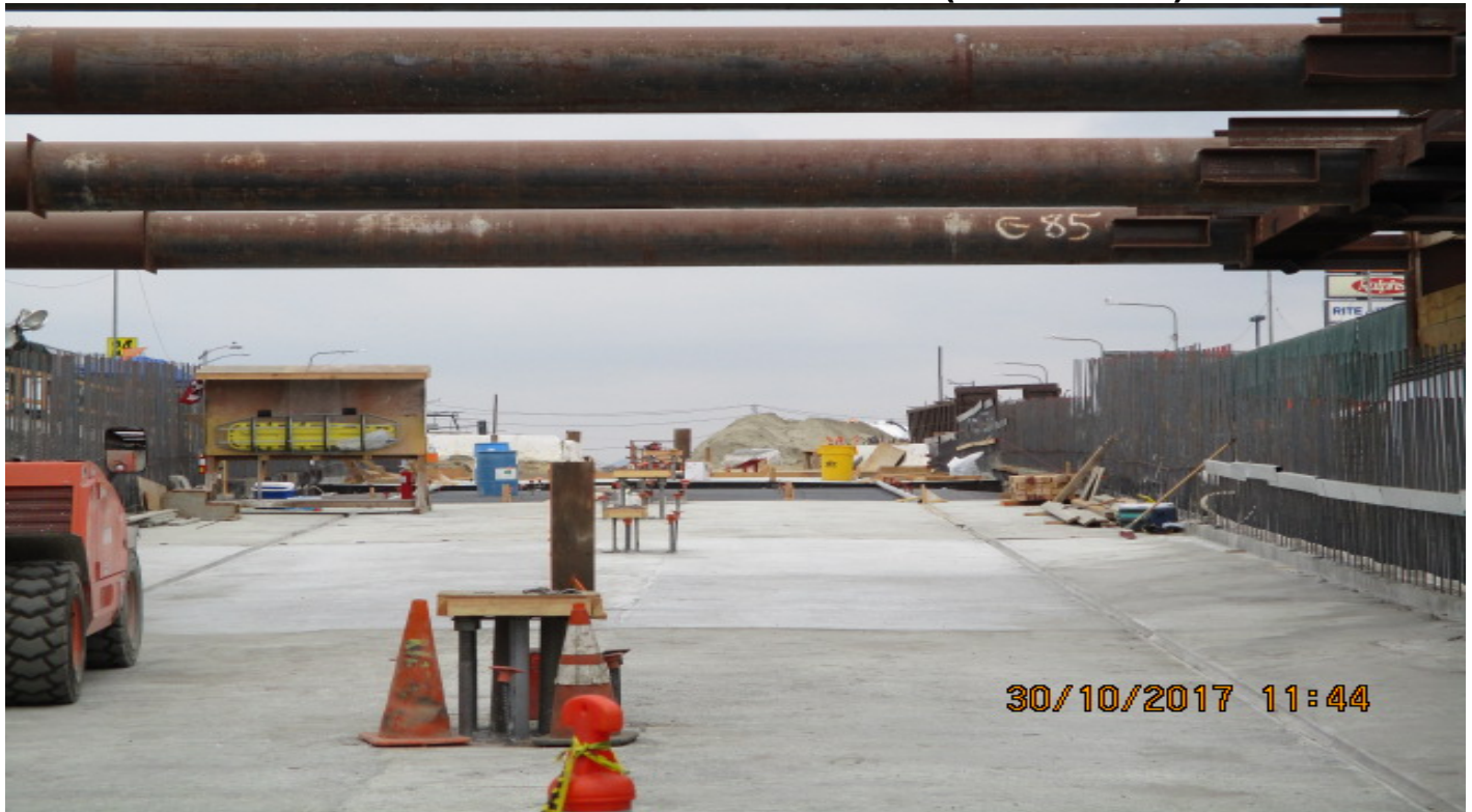
UG#3 - Approach slab at the north portal.
