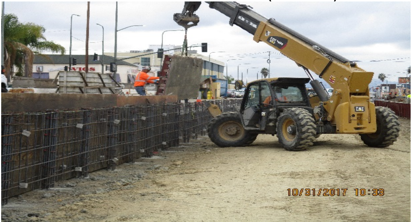
PARK MESA – Installing ballast wall formwork between 54th and 57th St.
