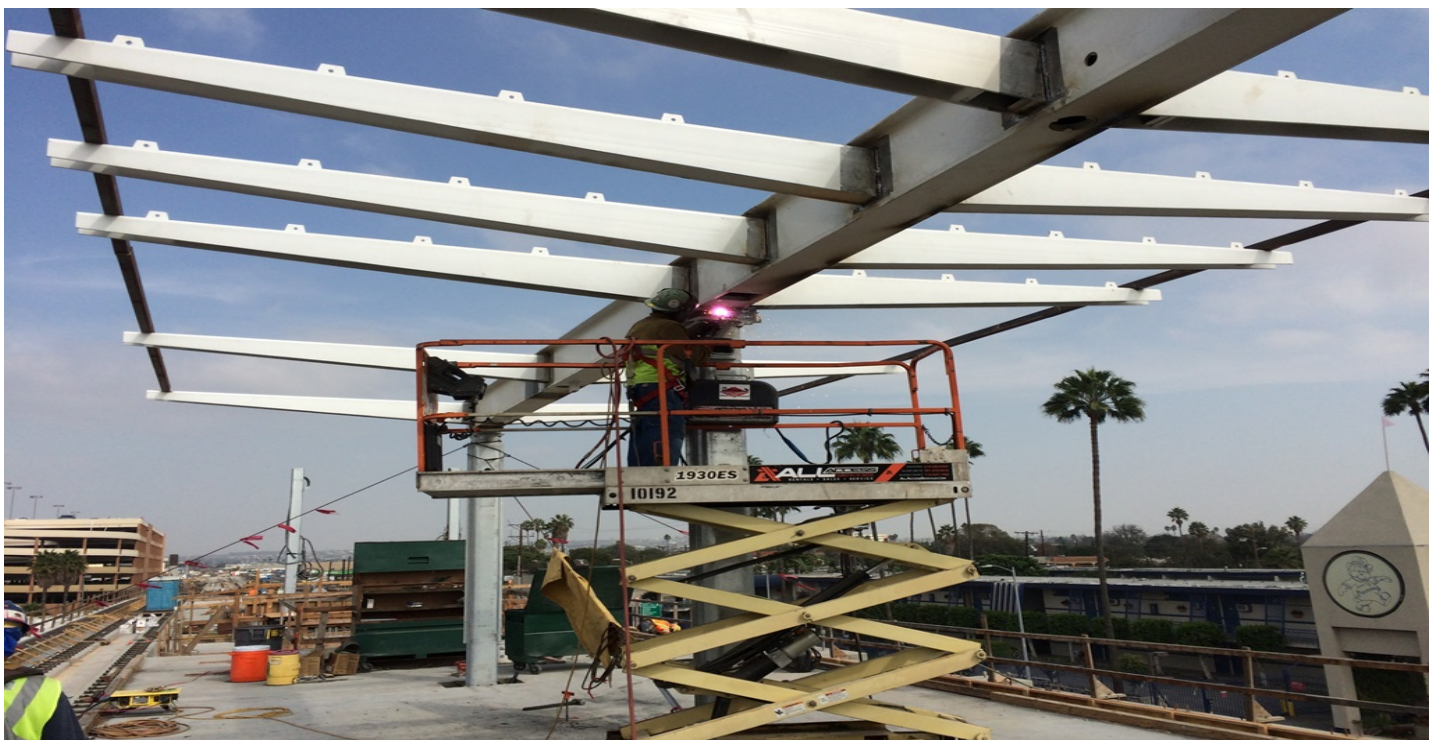
AVIATION/CENTURY BRIDGE -Full penetration weld between the canopy main beam and column in progress.
