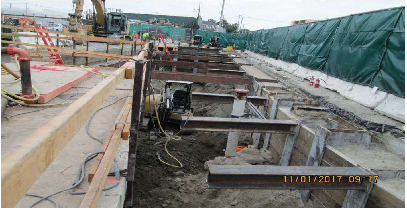
EXPOSITION/CRENSHAW STATION – Excavating at side structure “S”.
