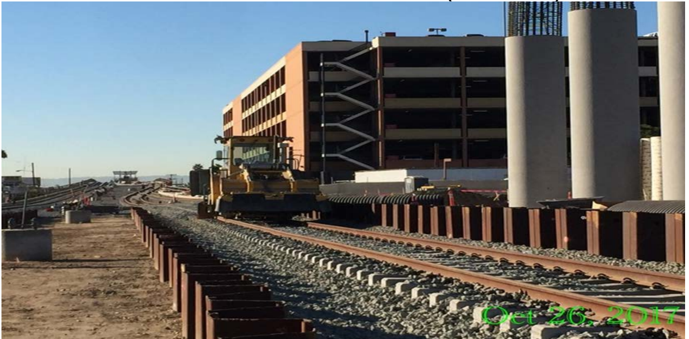
MSE 75L&R – Crew tamping, regulating and surfacing top ballast on track-3 SB from Vitae Street to Century Bridge.
