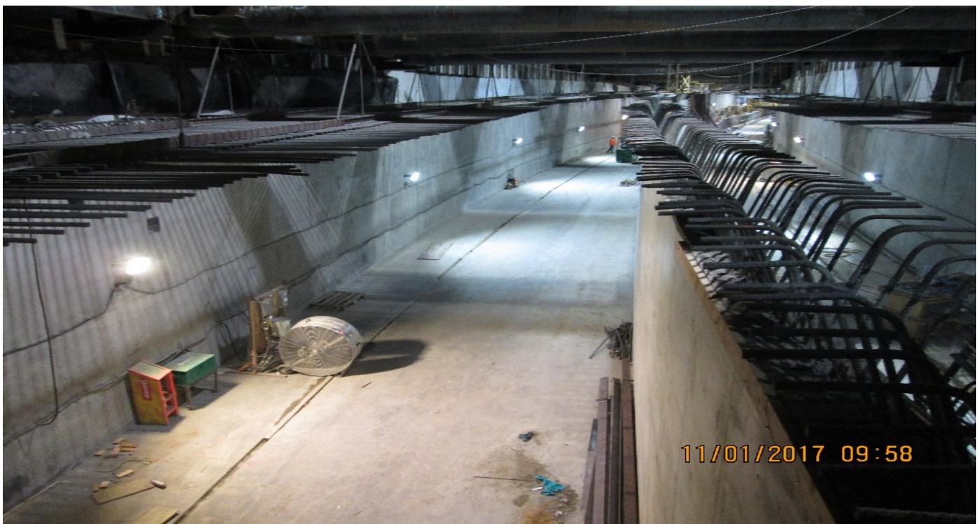
UG4 – East and center wall progress along the NB Guideway.
