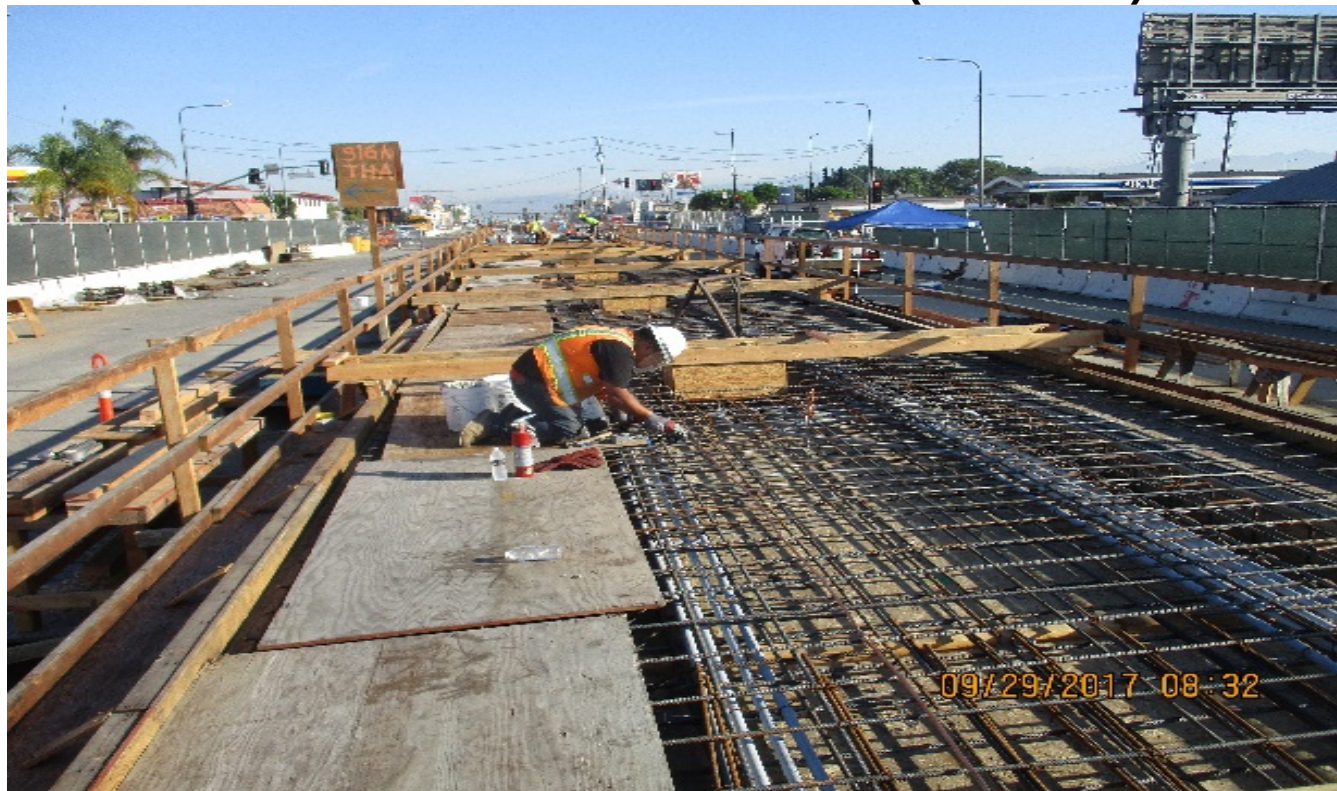
HYDE PARK STATION- Installation of electrical components in the platform deck.
