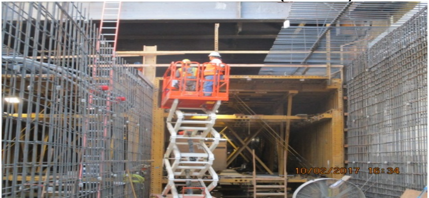
UG#3 - Installation of formwork for traveler section 47.
