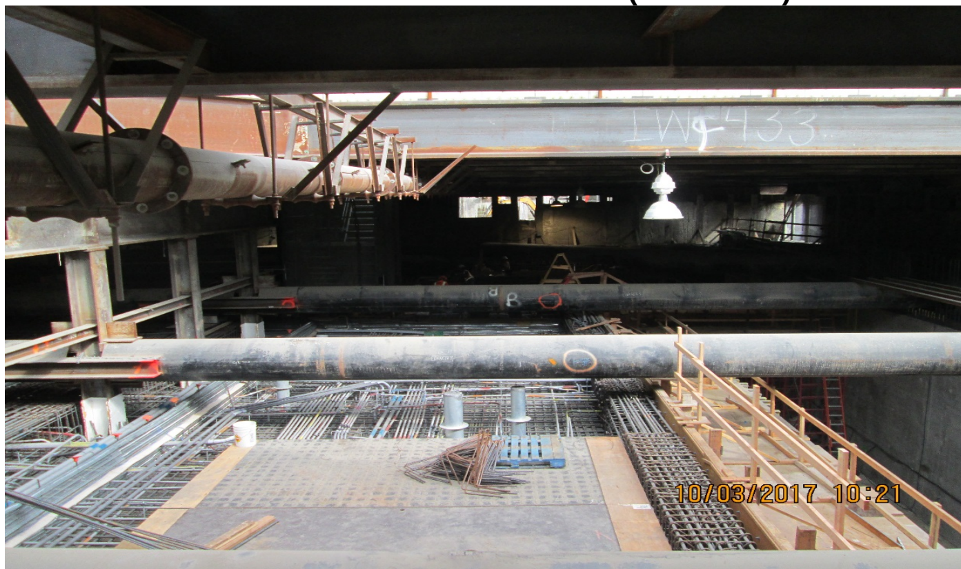
EXPOSITION/CRENSHAW STATION – Installing rebar for Roof Slab Phase 1.
