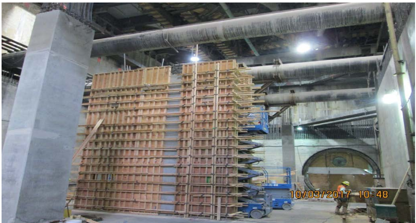
MARTIN LUTHER KING JR. STATION – Installing formwork for south emergency exit stair 1.
