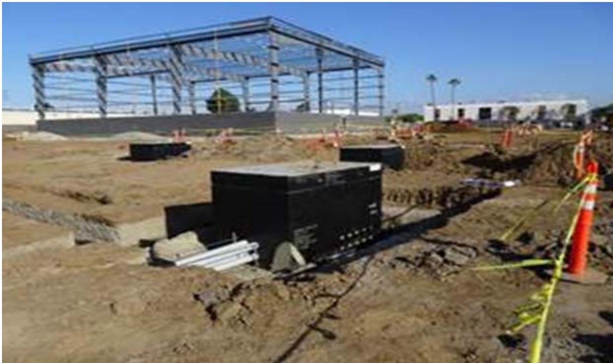
Southwestern Yard - Underground ductbank, vaults and material storage building.
