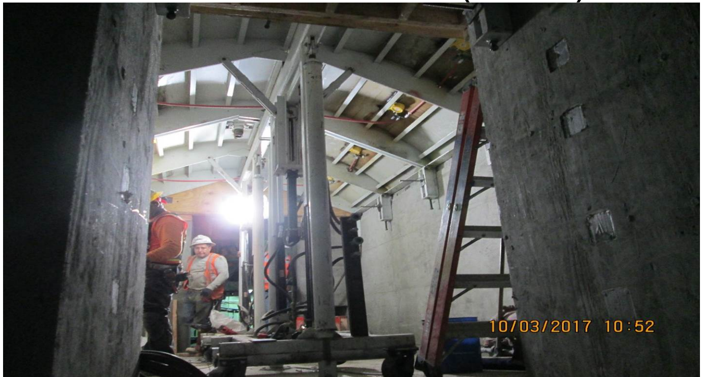
TUNNELING – Erecting arch section formwork at CP-5.
