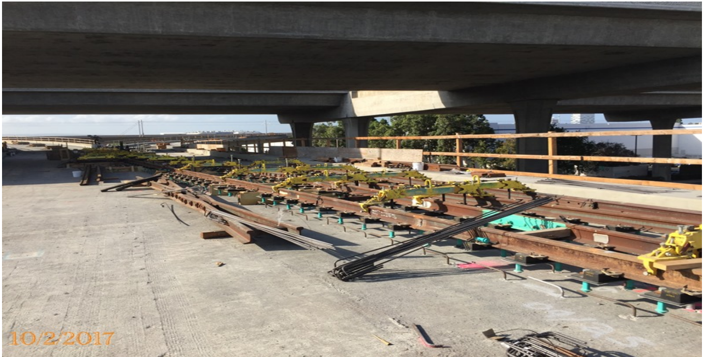
GREENLINE UNDERPASS – Bridge superstructure complete including approach slabs and joint seals. Special track work underway.
