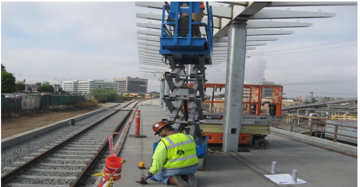
LA BREA AT GRADE STATION - Crews completed canopy outrigger welding and electrical and plumbing installations. Painting of structural steel and installation of canopy catwalks, gutters and glass panels to follow.
