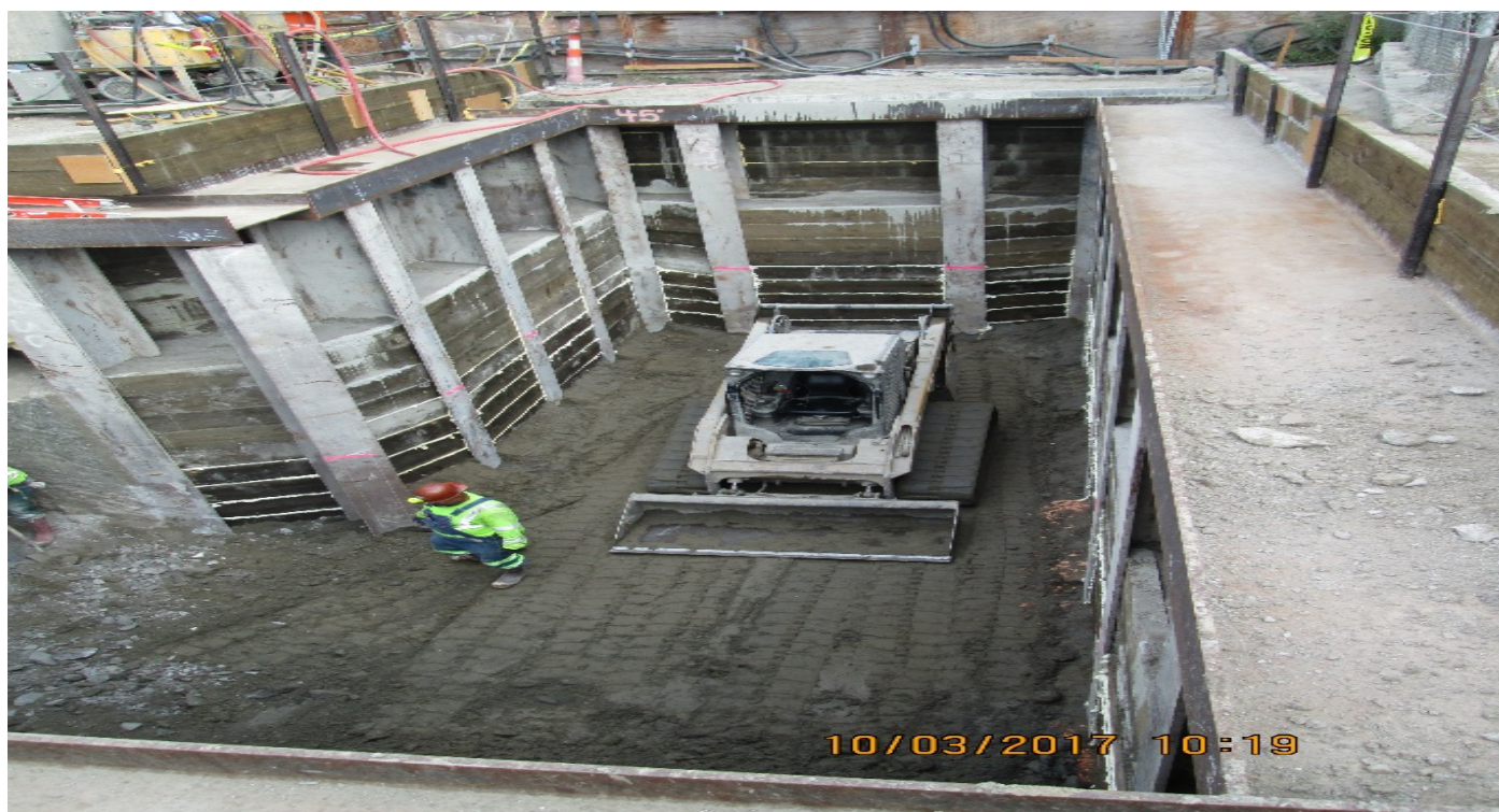
EXPOSITION/CRENSHAW STATION – Excavating at side structure “Q”.
