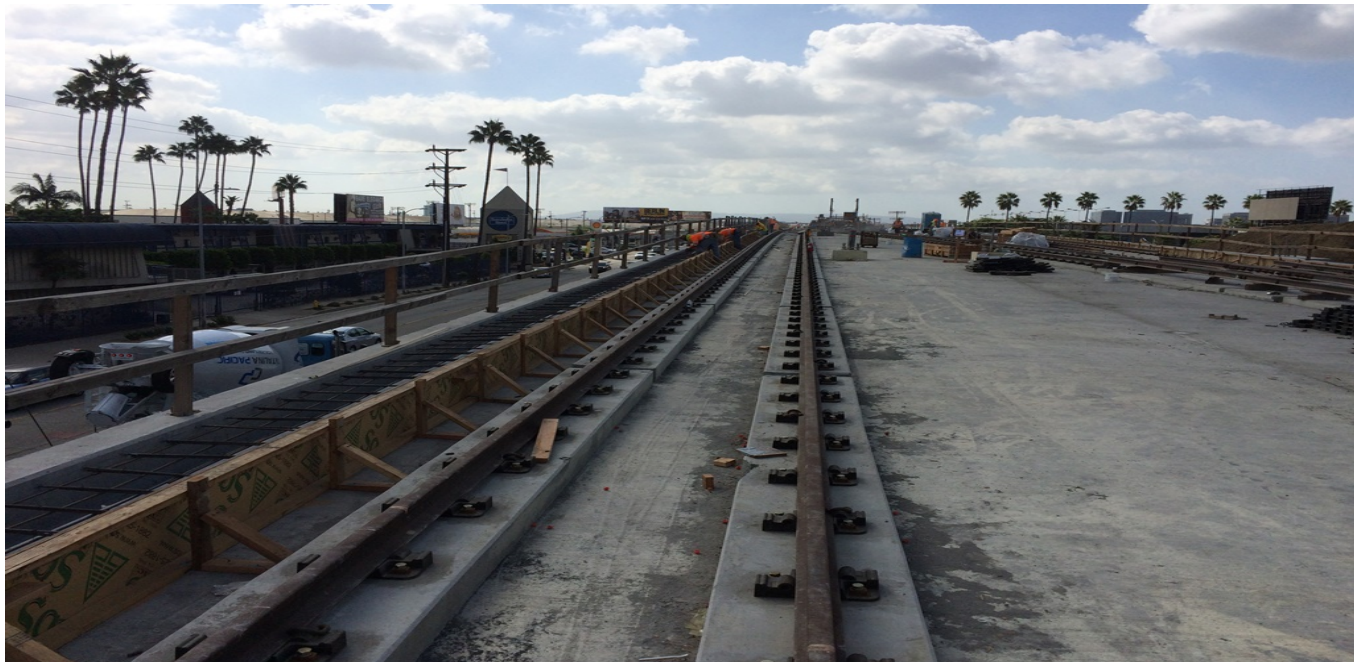
AVIATION/CENTURY BRIDGE – Northbound emergency walkway duct bank on the bridge deck.
