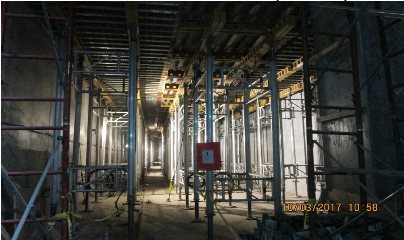
UG4 – Installing false work for roof sections R-28 thru R-25, south of Vernon portal.
