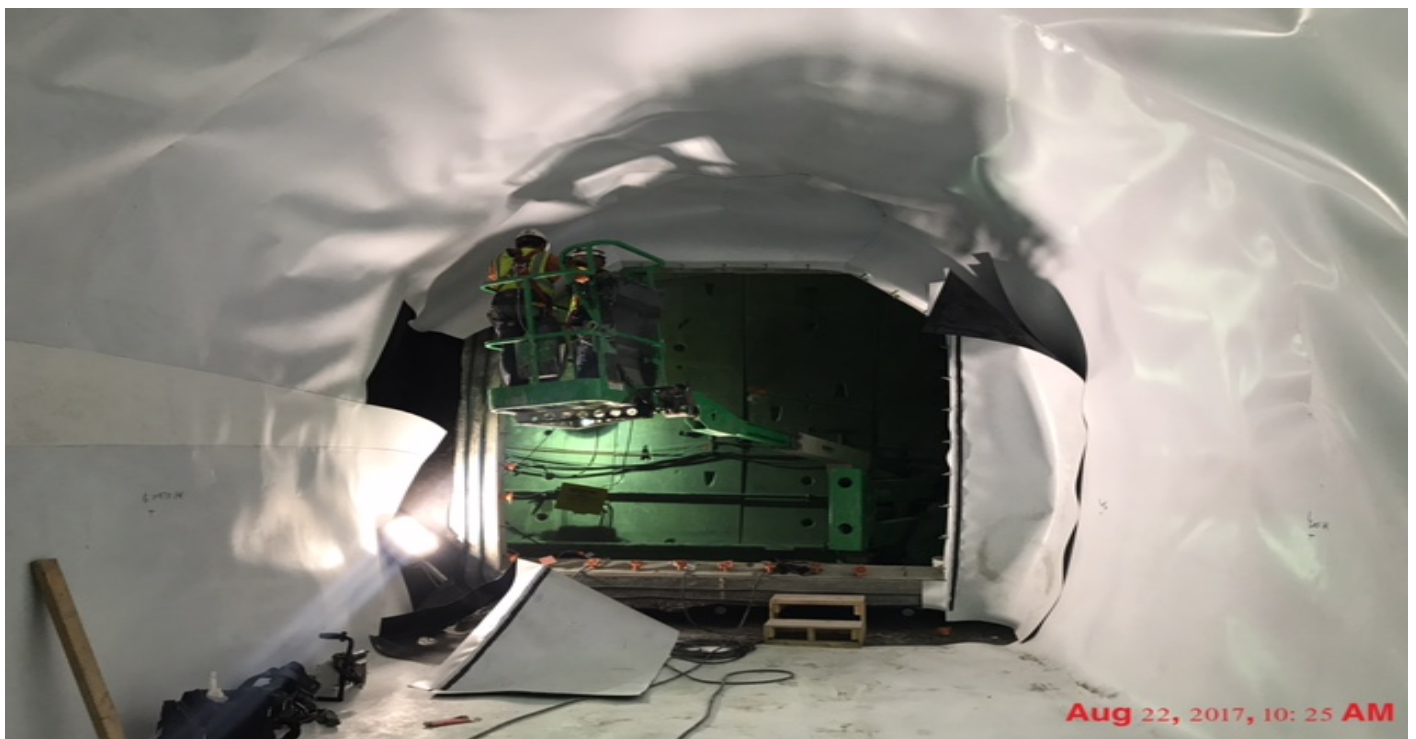
TUNNELING – Installation of waterproofing at CP-2.
