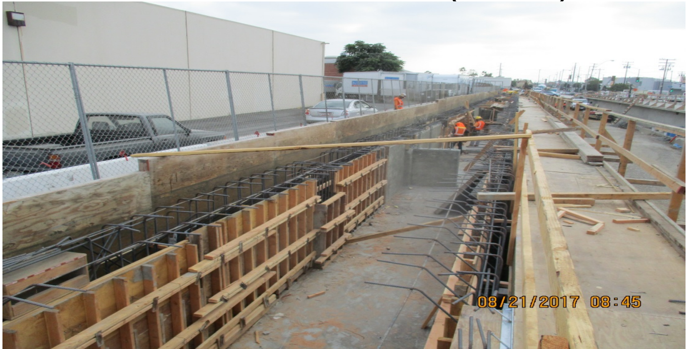
WESTCHESTER STATION – Exterior finish work continued along the NB platform stem walls.
