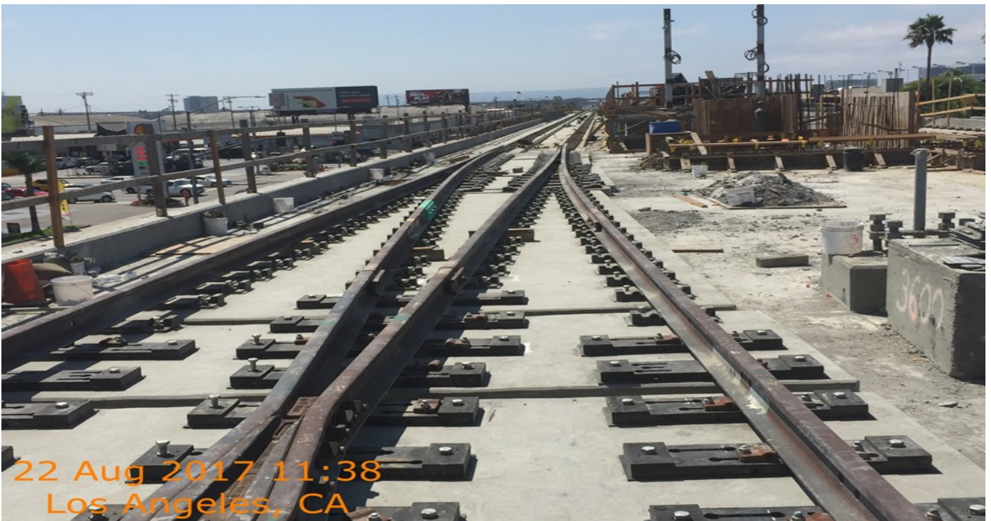
AVIATION/CENTURY BRIDGE – K1 switch for the #10 crossover facing down-station.
