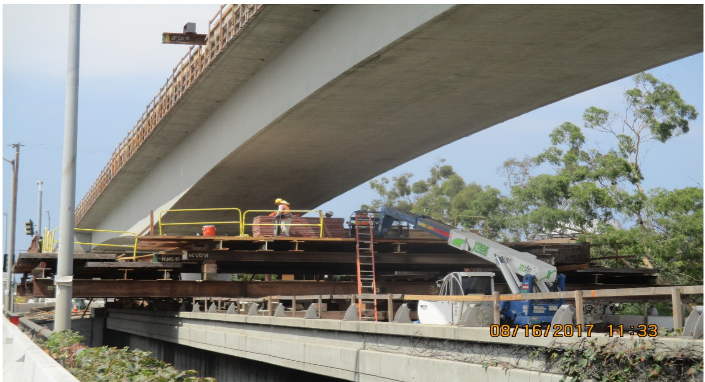
(AG-5) I-405 BRIDGE – Falsework removal complete.
