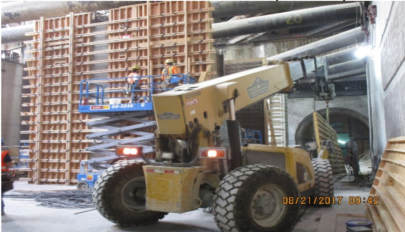
MARTIN LUTHER KING JR. STATION – Installation of formwork for north emergency stairs interior walls.
