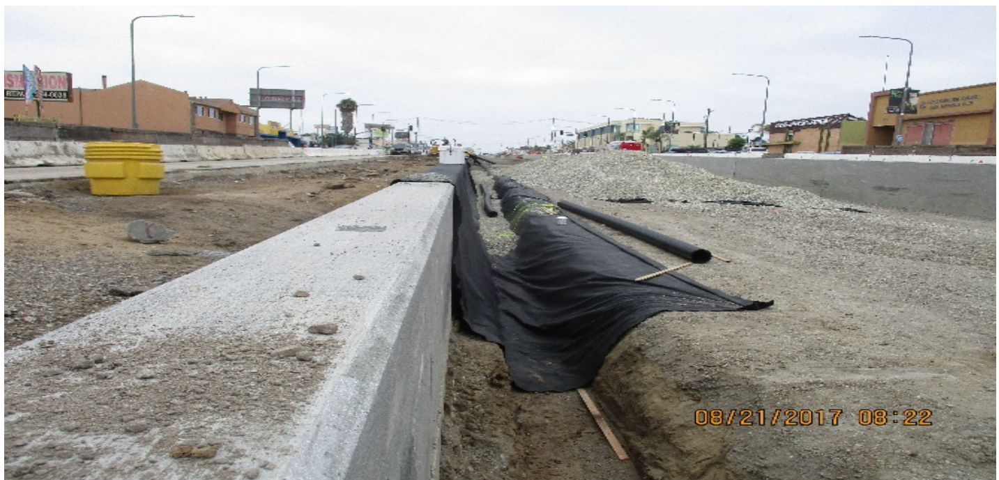
PARK MESA —Backfill activities along the northbound ballast walls between 50th and 52nd St.
