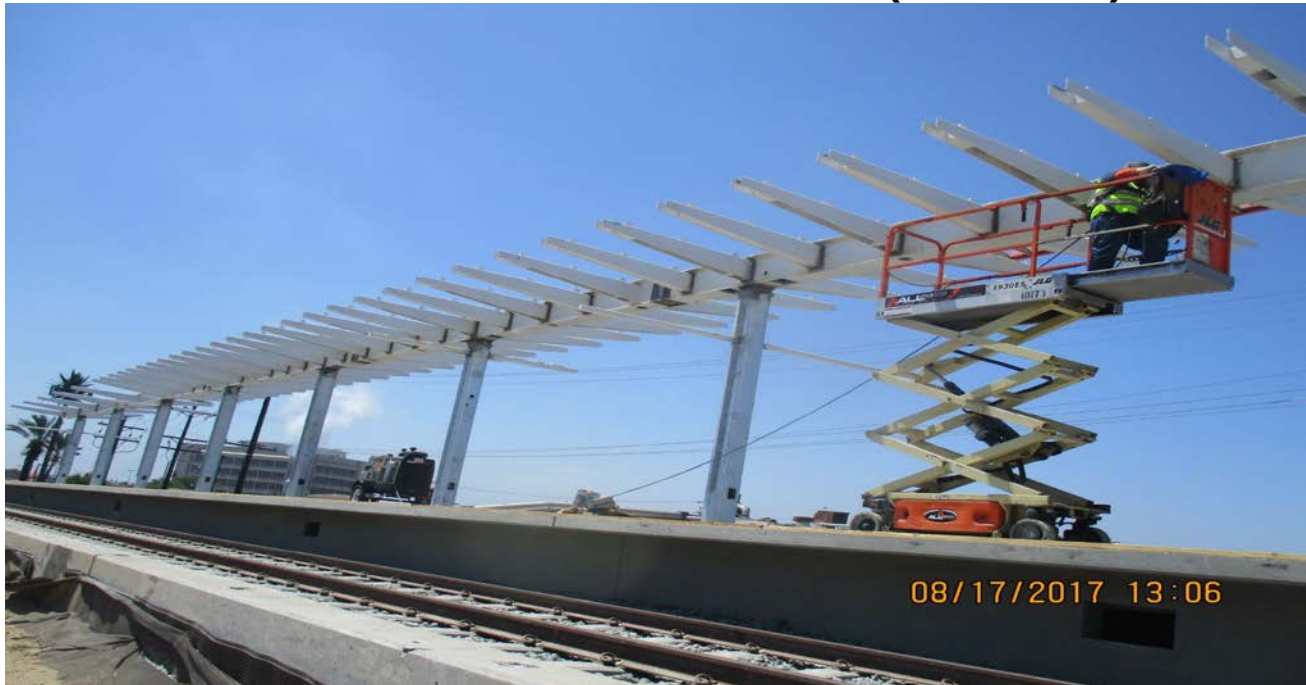
LA BREA AT GRADE STATION - Canopy frame erection complete. Crews worked on welding mounting brackets and electrical and plumbing installations.
