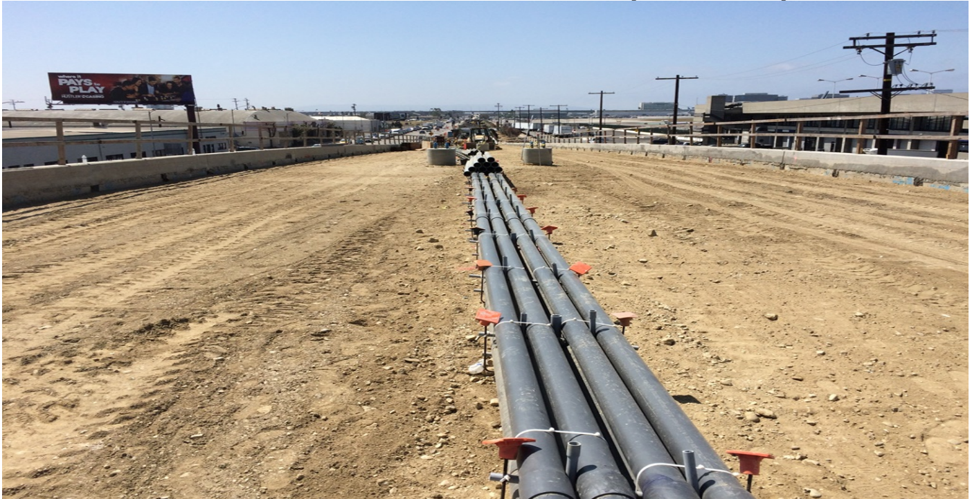
MSE 60L&R –Crews finished fine-grading in preparation for AC cap placement and Neil Electric laid conduit for the combined emergency walkway/ductbank.
