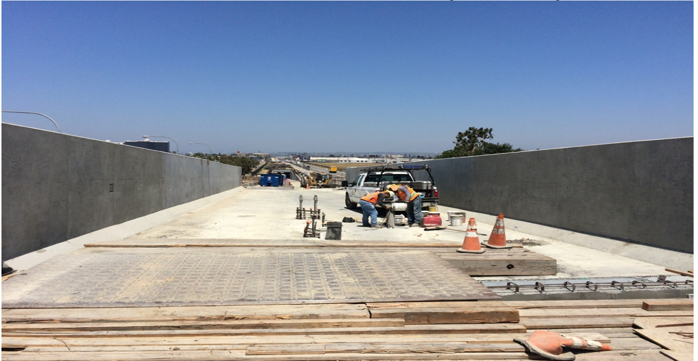
111 th Street – Bridge superstructure complete, DF track plinths to follow. Crews worked on girder wall finish work.
