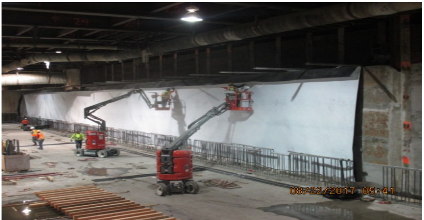
LEIMERT PARK STATION - Installing waterproofing along concourse level wall sections UW-1 thru UW-4.
