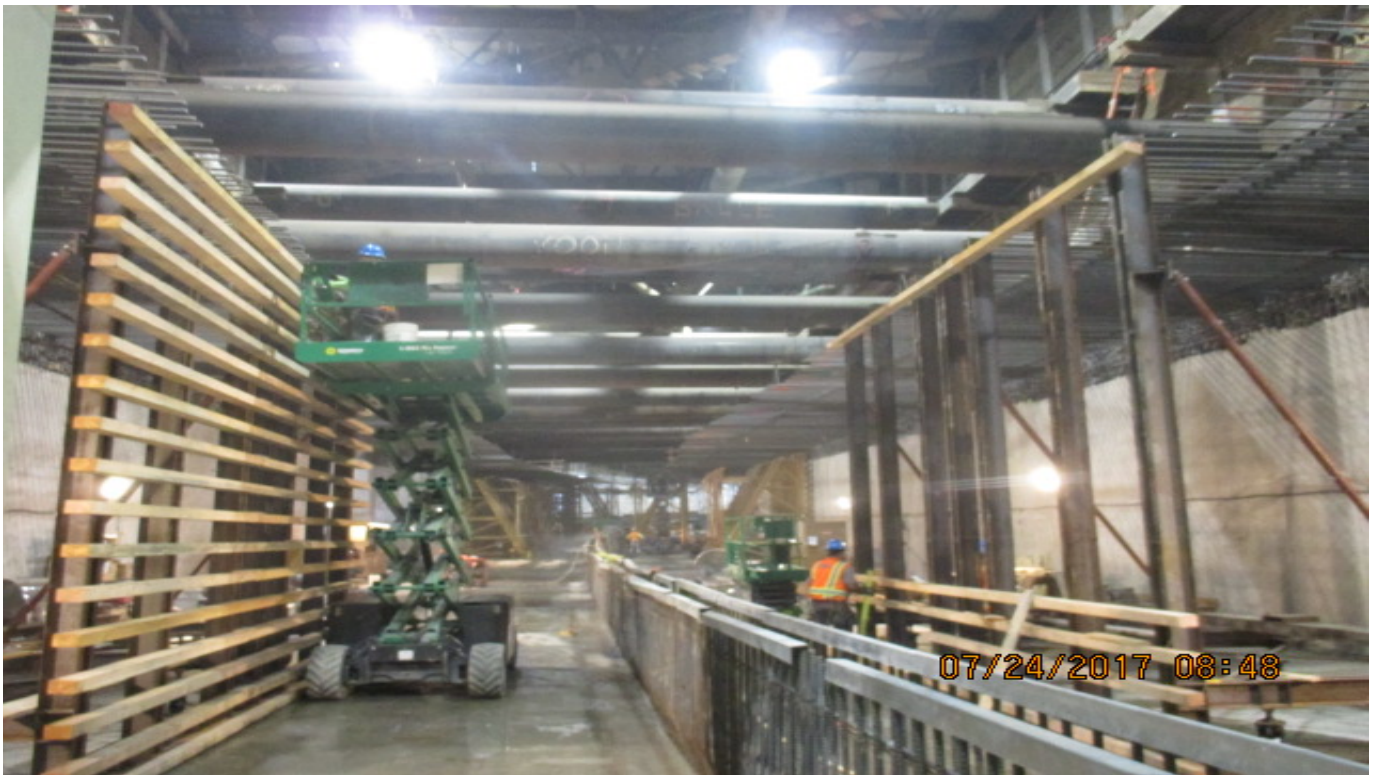
UG4 – Fabrication of Center Wall formwork.
