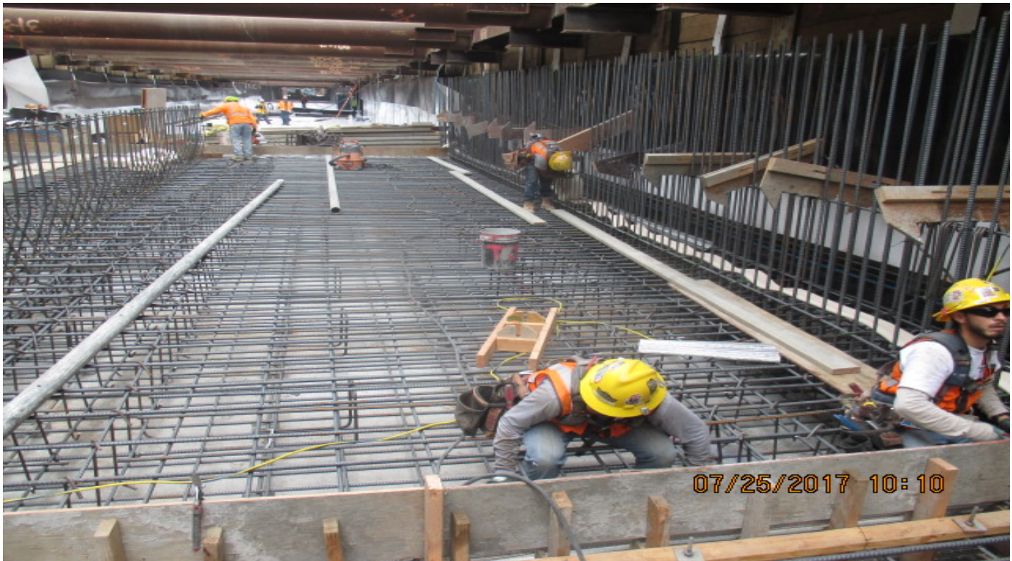
UG#3 - Preparing for invert placement at section P-44.
