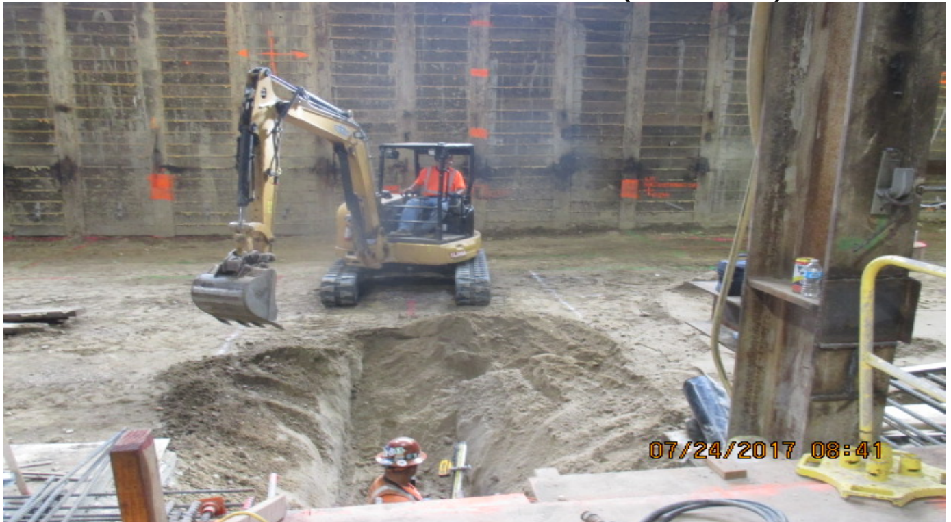
LEIMERT PARK STATION – Excavating at side structure for installation of utilities.
