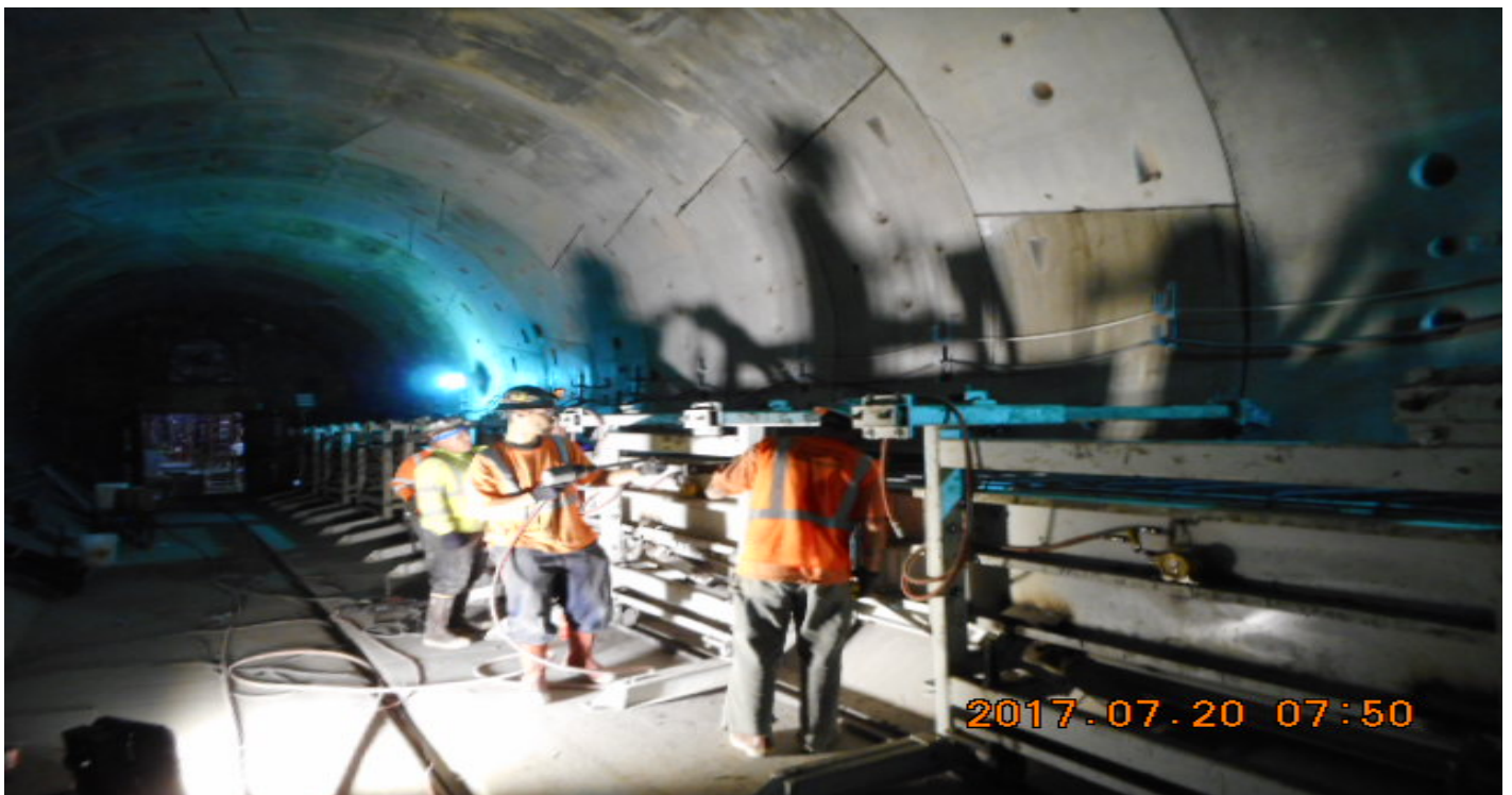
TUNNELING – Preparing for placement of SB Tunnel Walkway section 7a.
