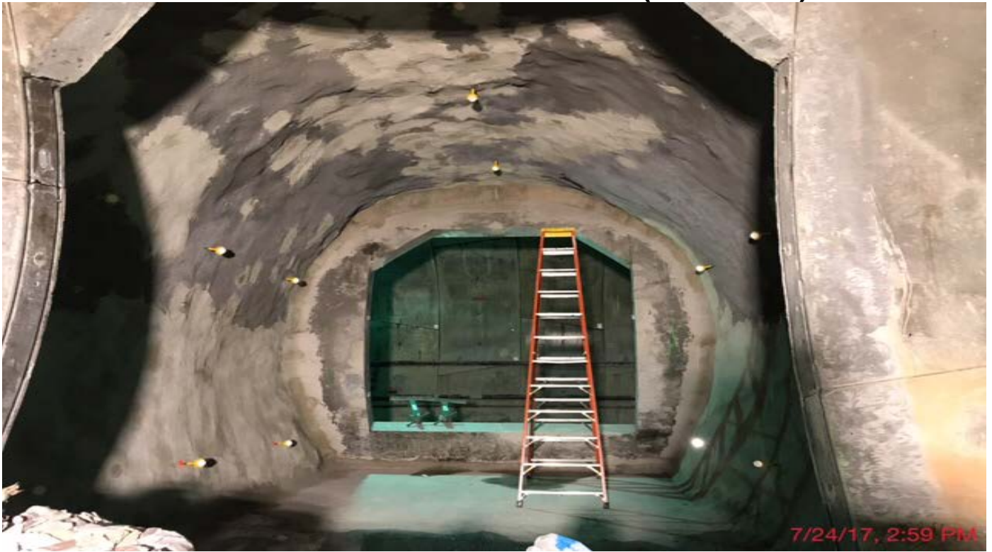
TUNNELING – Cross Passage #3 ready for waterproofing.
