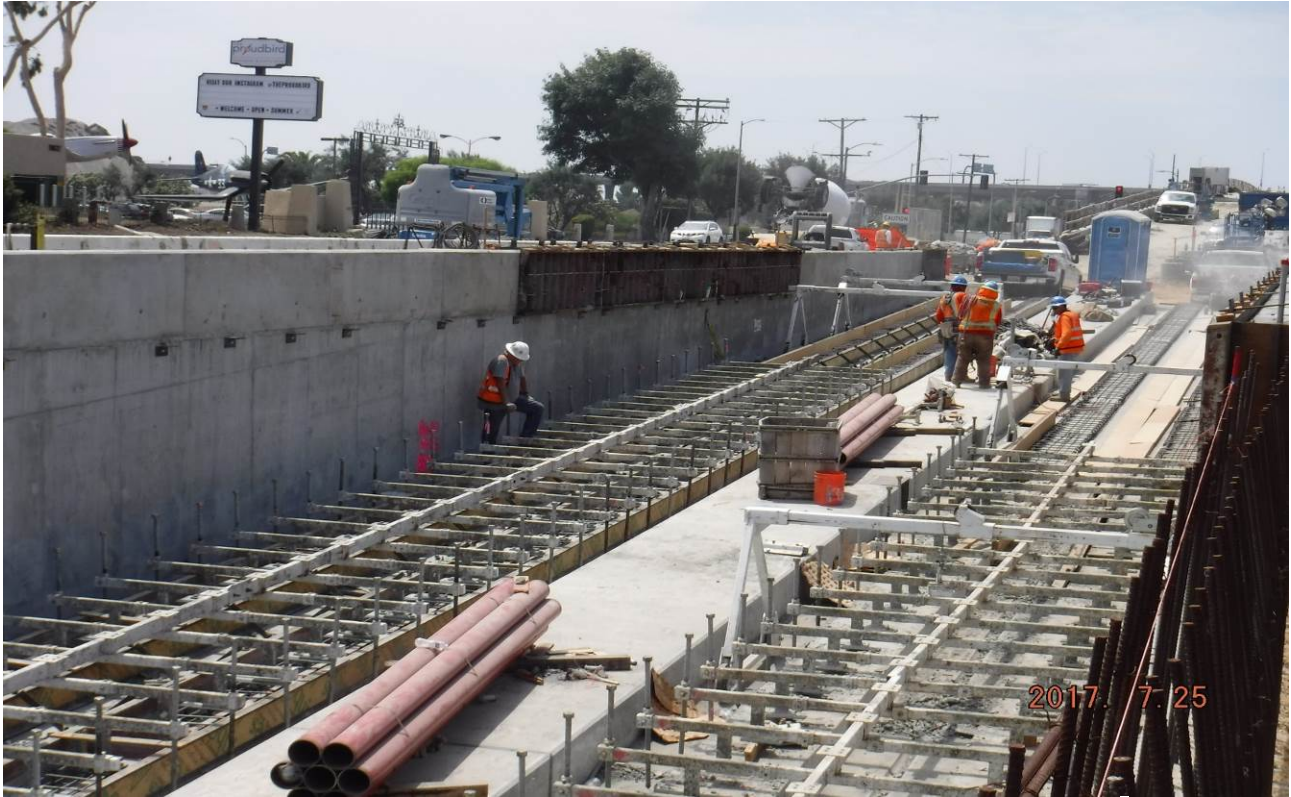
UG#1 - Bottom-up plinth construction nearing completion at UG1.
