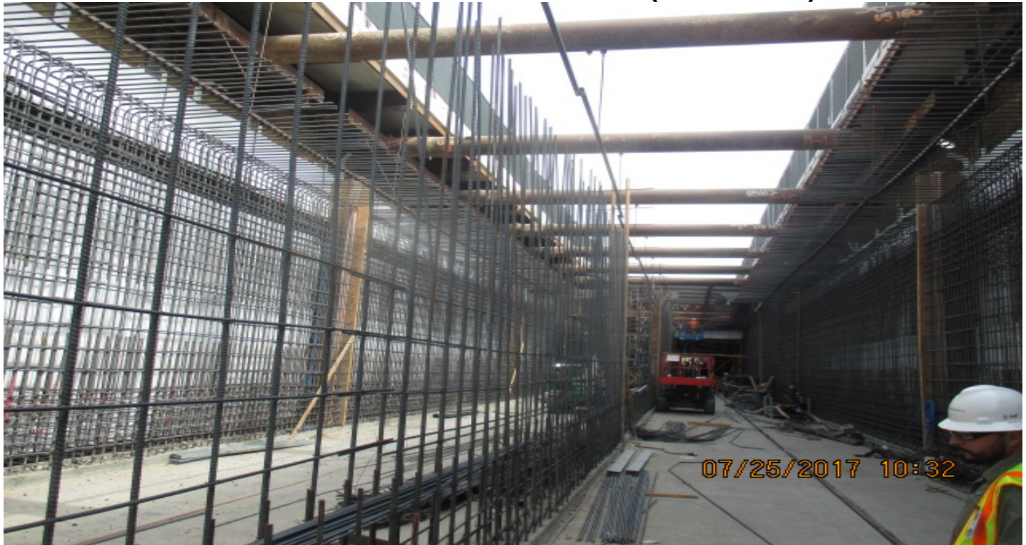
UG#3 - Installation of rebar for Center Wall (CW) sections 21 and 22.
