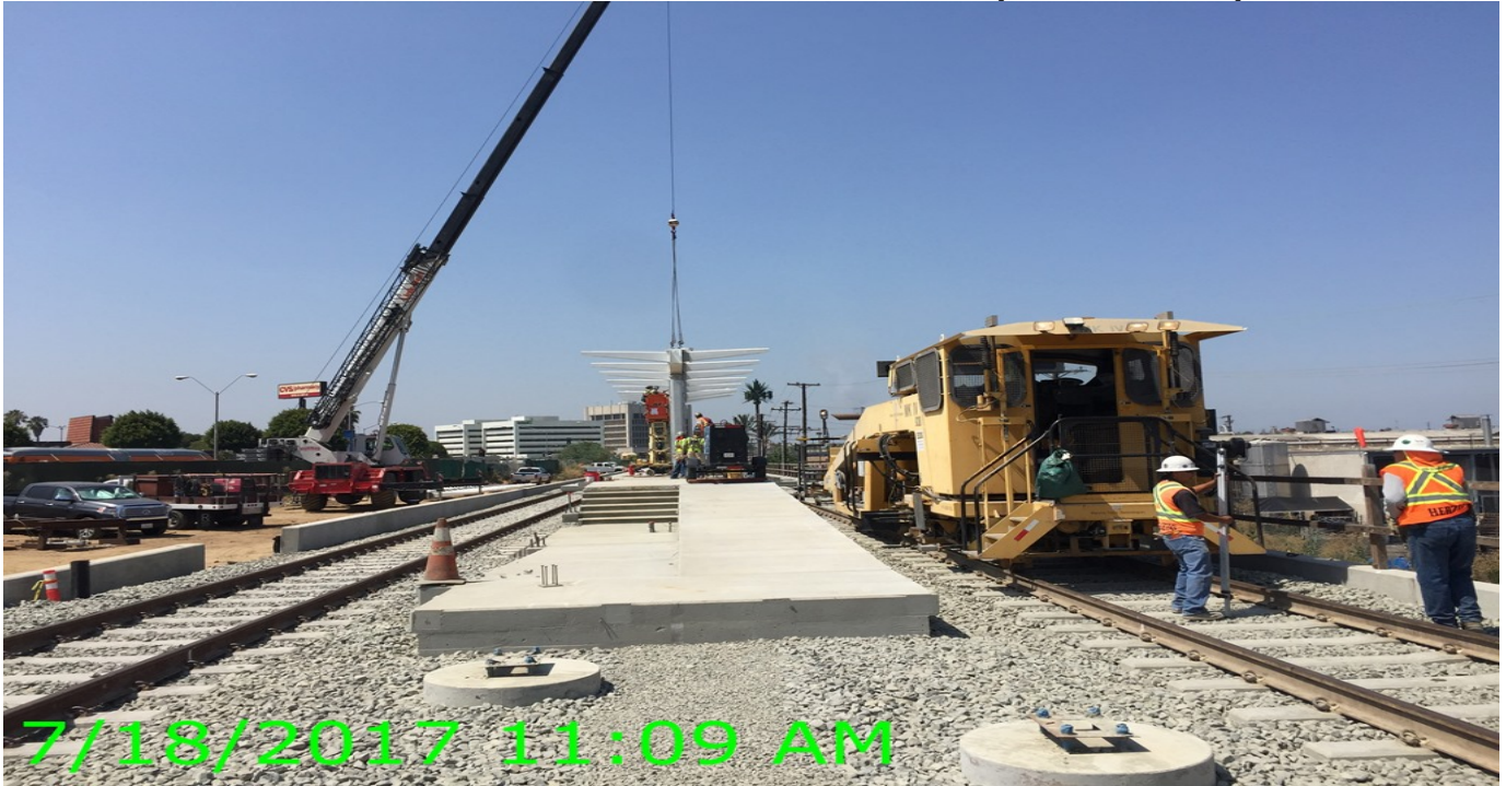
B1 GUIDEWAY – Between La Brea station and Centinela Ave.
