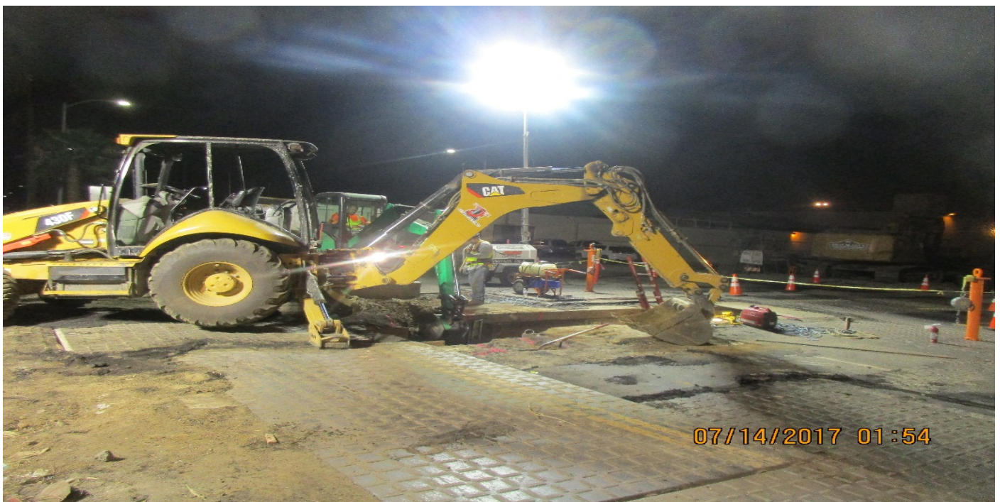
ARBOR VITAE GRADE CROSSING – Mainline ductbank excavation underway.
