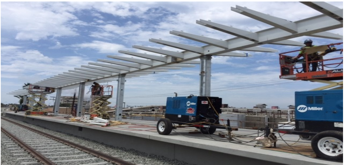
LA BREA AT GRADE STATION - Canopy frame erection underway.
