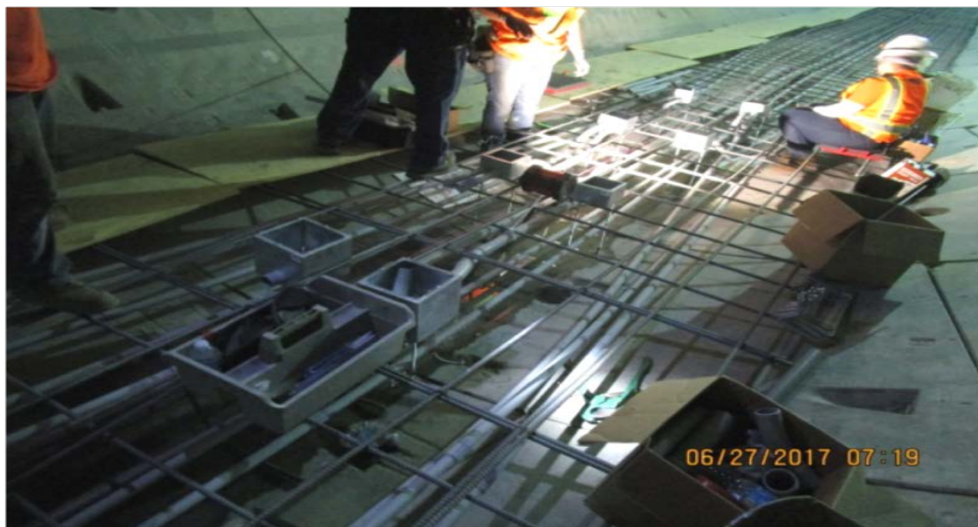
TUNNELING – Installation of electrical components/conduits for the NB tunnel invert between Expo and MLK.
