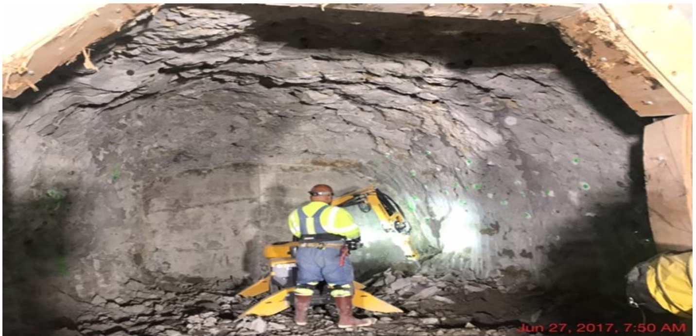
TUNNELING – Excavation of jet-grouted soils at CP-4.
