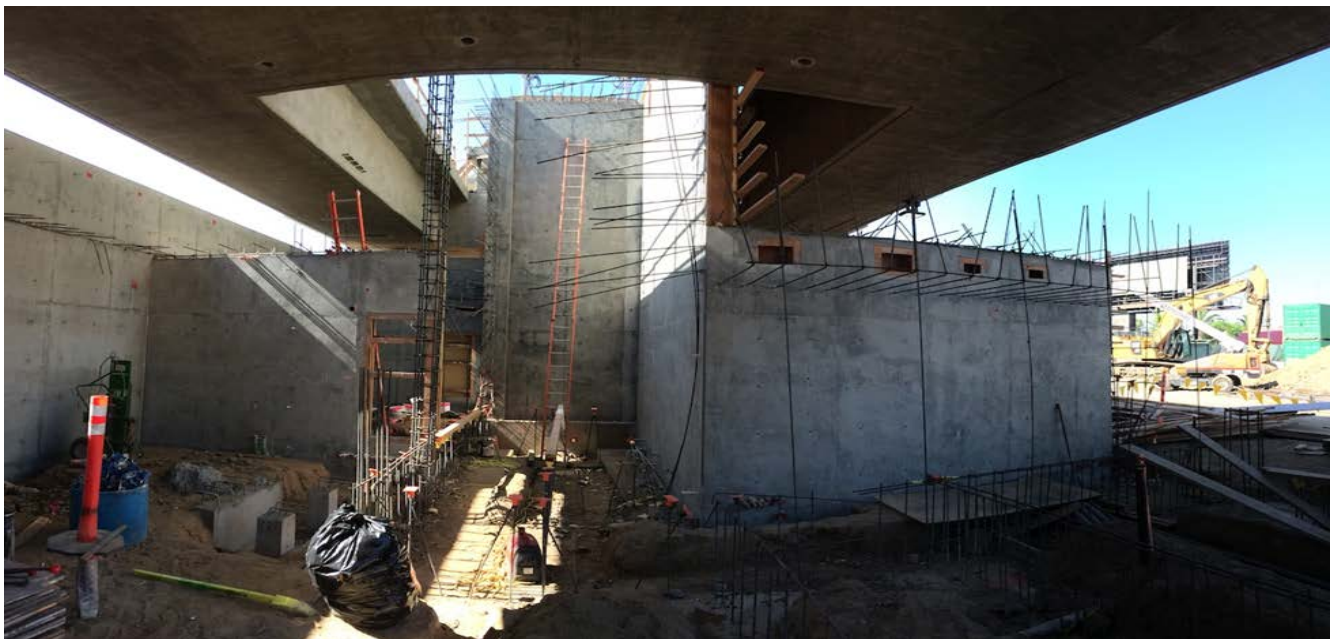
AVIATION/CENTURY BRIDGE – Construction of the plaza level service building and station elevator shaft underway.
