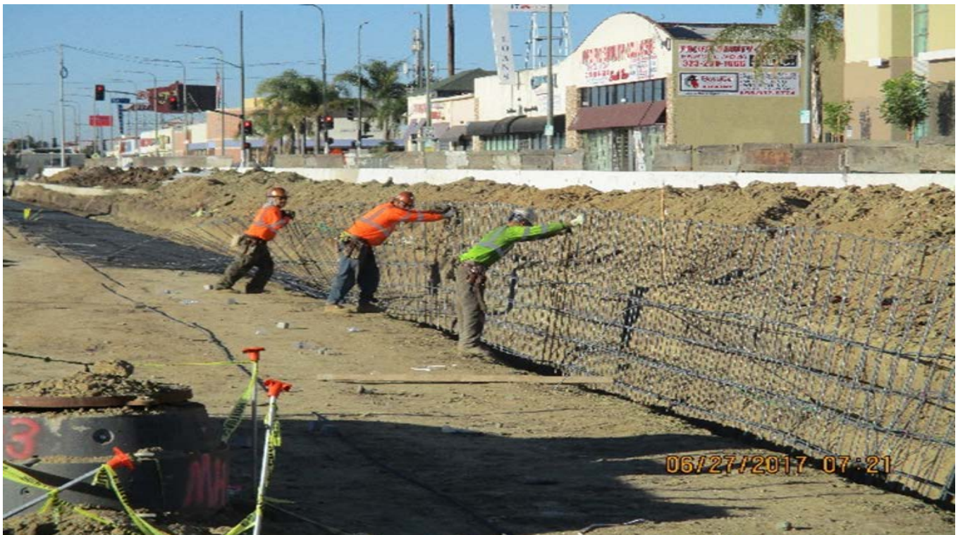
PARK MESA – Installation of ballast wall along west wall between 52nd St. and 54th St.
