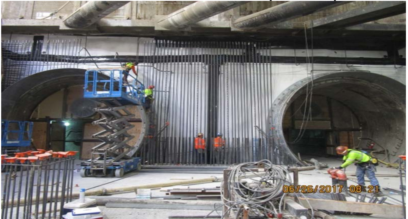
MARTIN LUTHER KING JR. STATION – Installation of rebar along south lower walls and installation of NB/SB Omega rings at south hammerhead.
