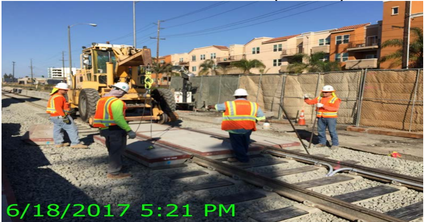
OAK ST. GRADE CROSSING - Crews finished the Oak Street grade crossing.
