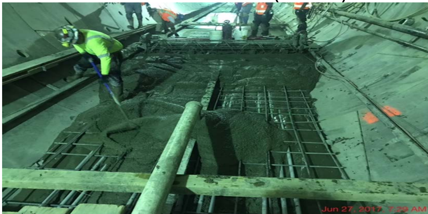
TUNNELING – Placement of NB Tunnel Invert section 10.
