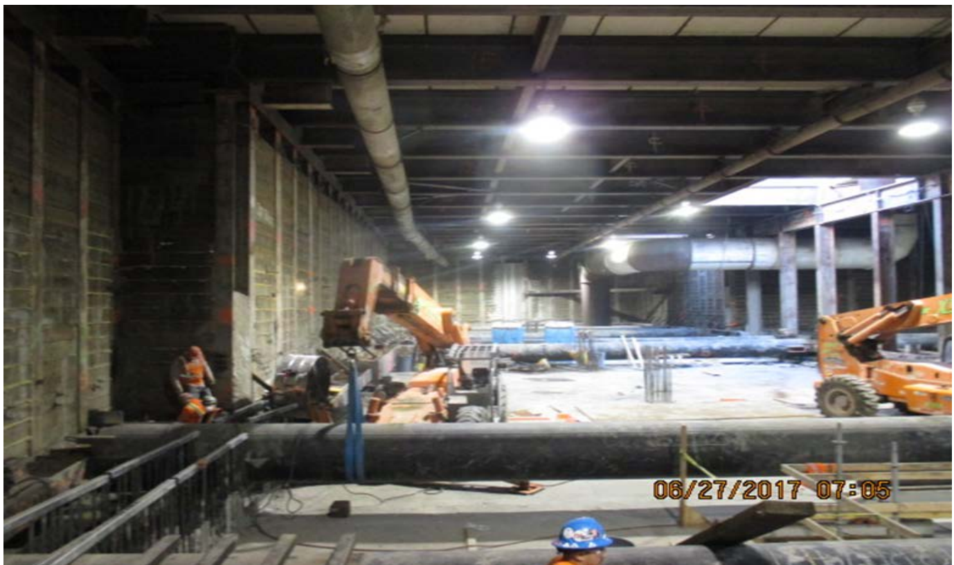
LEIMERT PARK STATION – Removing Tier-2 struts.
