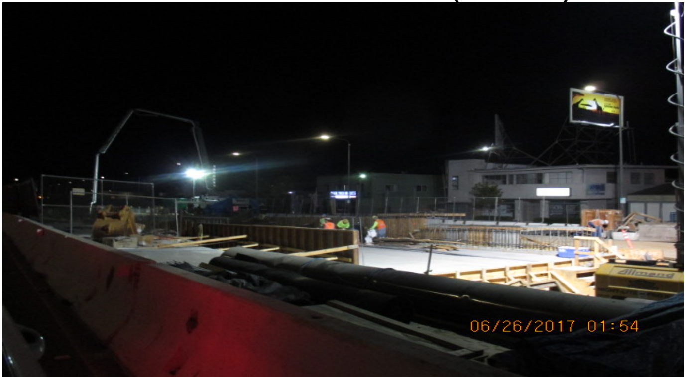
UG4 – Placement of invert sections I-2 and I-4; UG4 invert is now complete.
