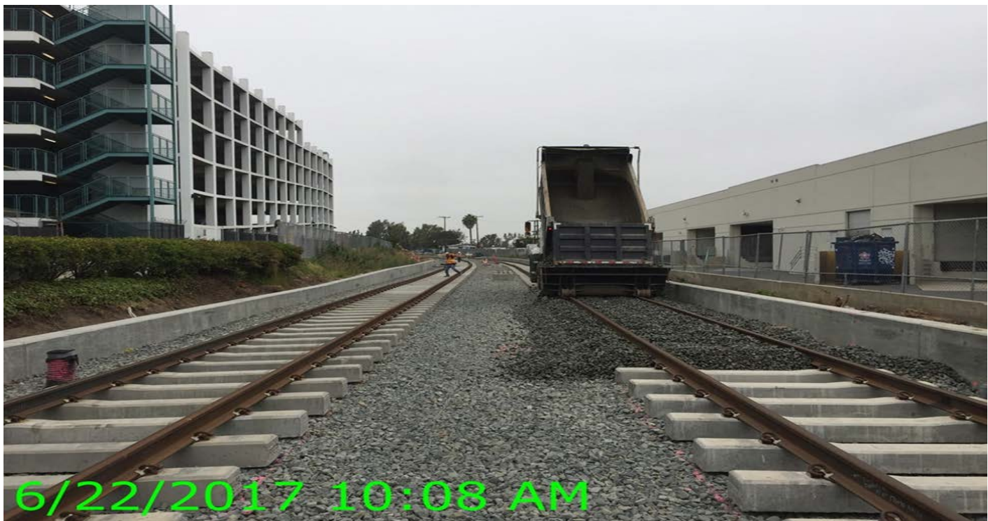
Ballasted track between Cedar and Eucalyptus.
