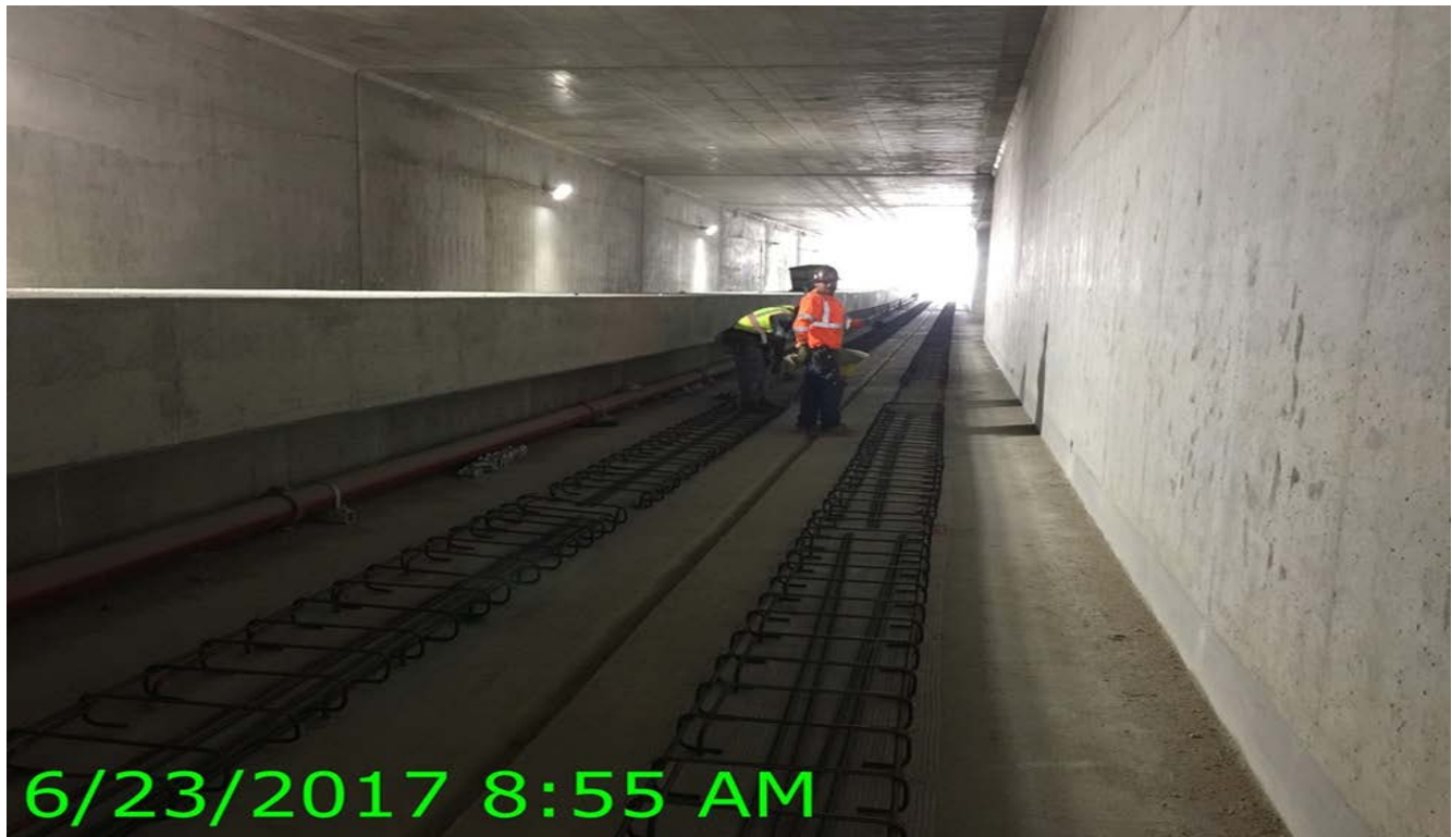
UG#1 – UG1 plinth construction underway.
