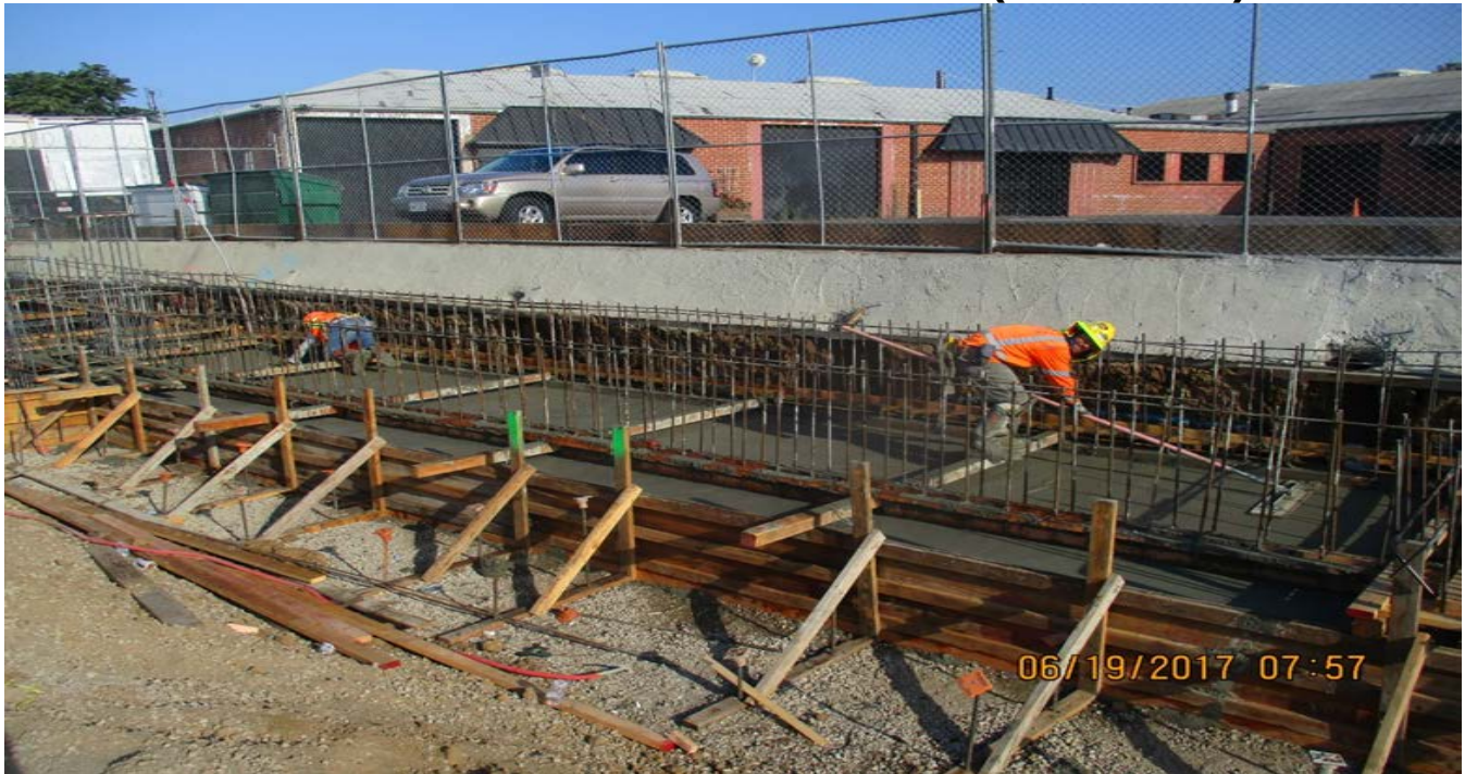
WESTCHESTER STATION – Crews continued with finish work for the north bound station platform. Crews placed concrete for the south bound platform footing.
