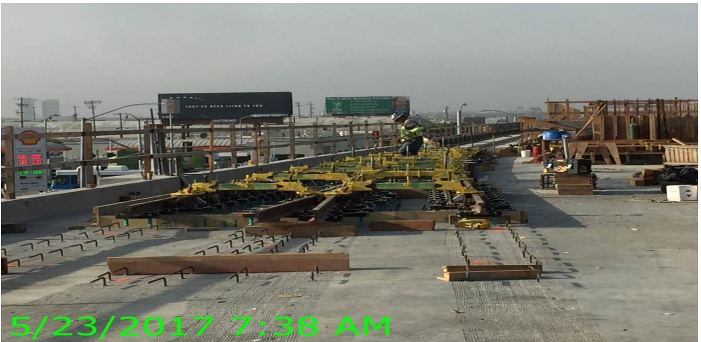
AVIATION/CENTURY BRIDGE – Top down construction of the 10K1 crossover utilizing the Iron Horse system underway at Aviation Century.
