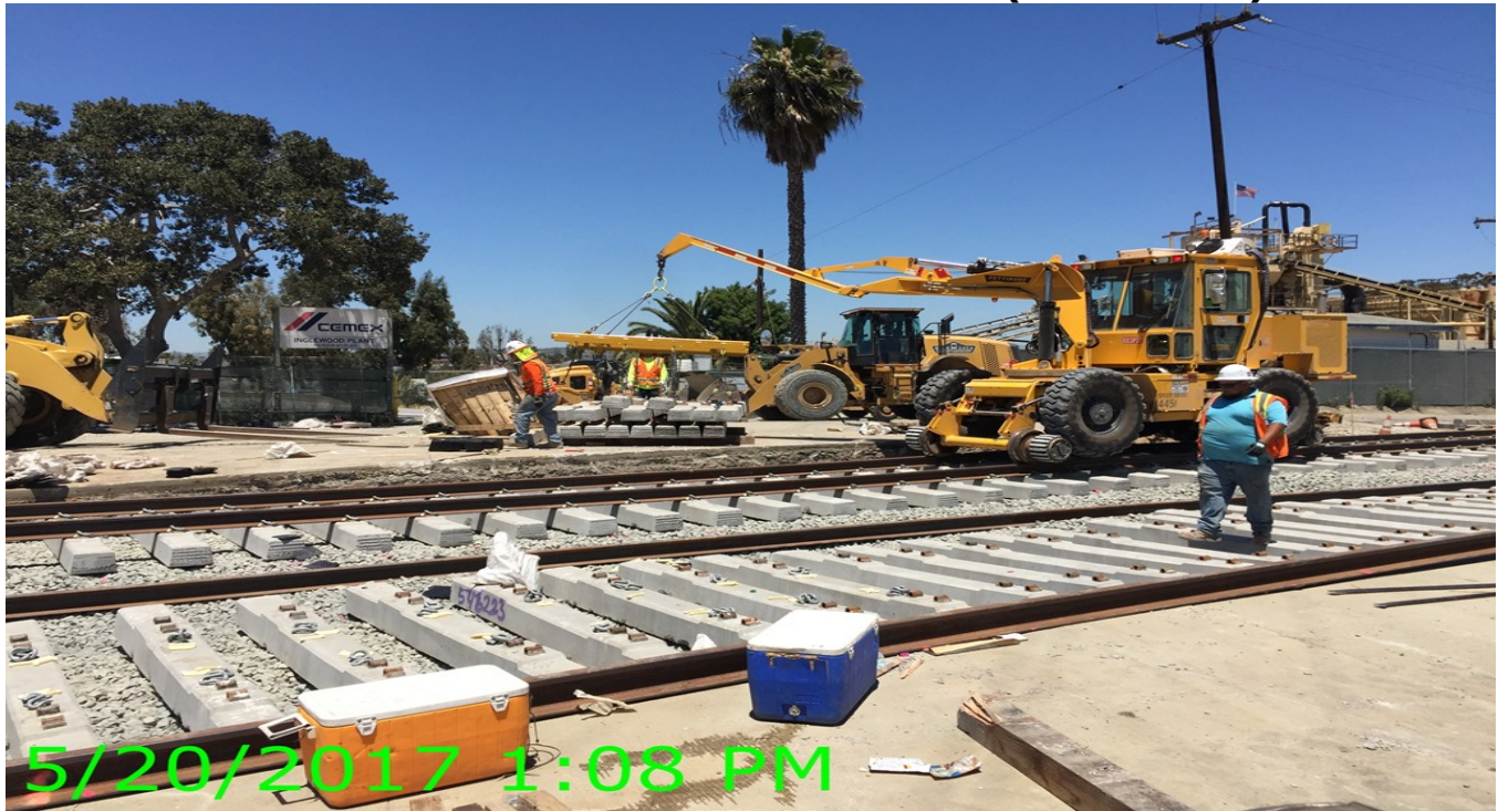
CEDAR GRADE CROSSING - Setting ties.
