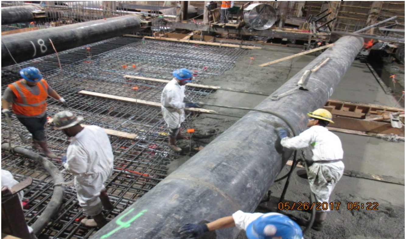
LEIMERT PARK STATION – Placement of concourse deck section C-2.
