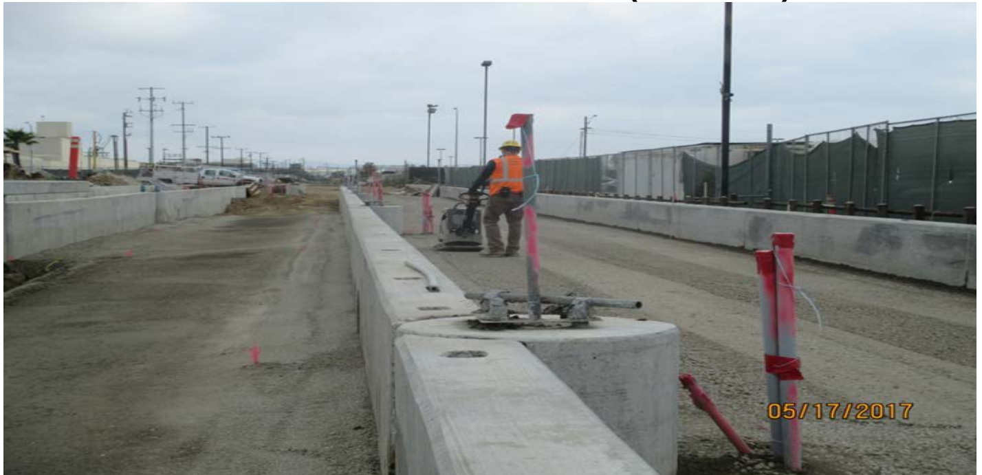
96 th STATION ACCOMODATIONS – Sub Ballast placement and compaction underway.
