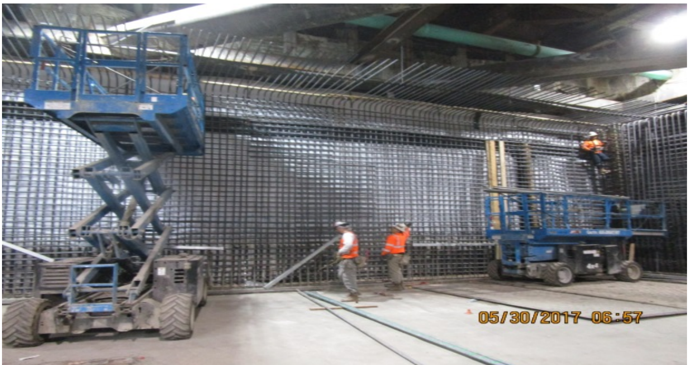
EXPOSITION/CRENSHAW STATION – Installation of rebar for concourse level wall sections G-22 and G-23.
