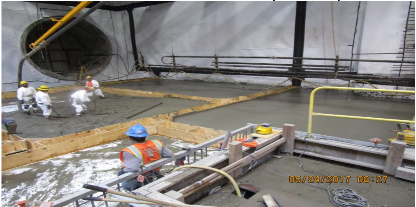
MARTIN LUTHER KING JR. STATION Placement of protection slab at north hammerhead.
