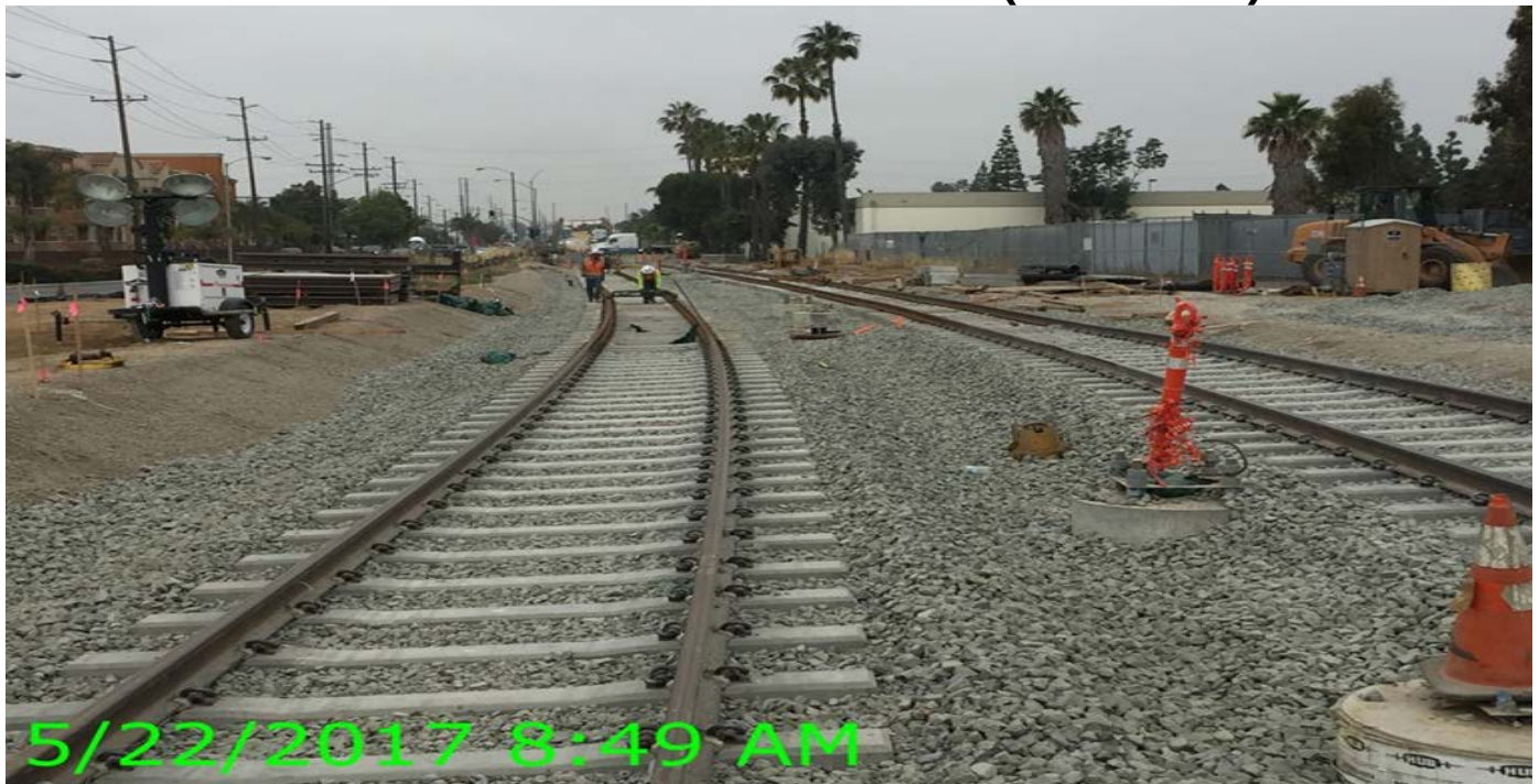
Ballasted track work between Oak and Cedar.
