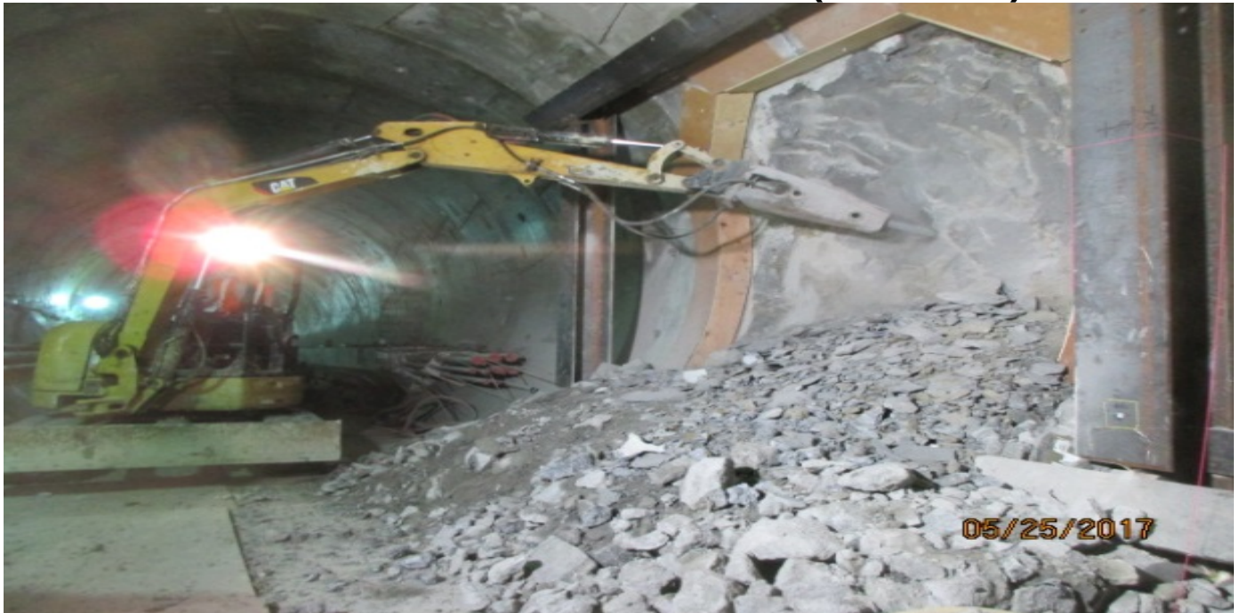
TUNNELING – Excavating into Cross Passage 5.
