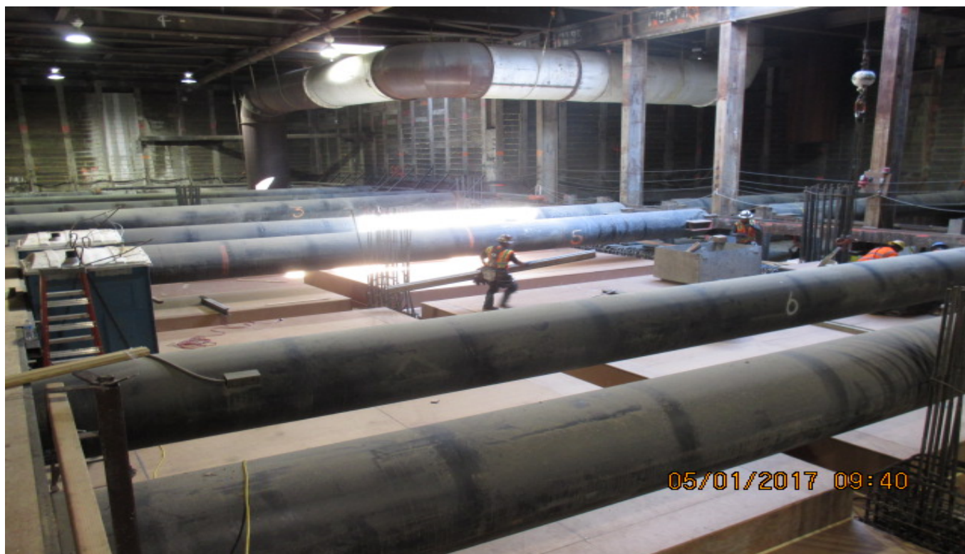
LEIMERT PARK STATION – Installation of formwork and rebar for concourse level slab.
