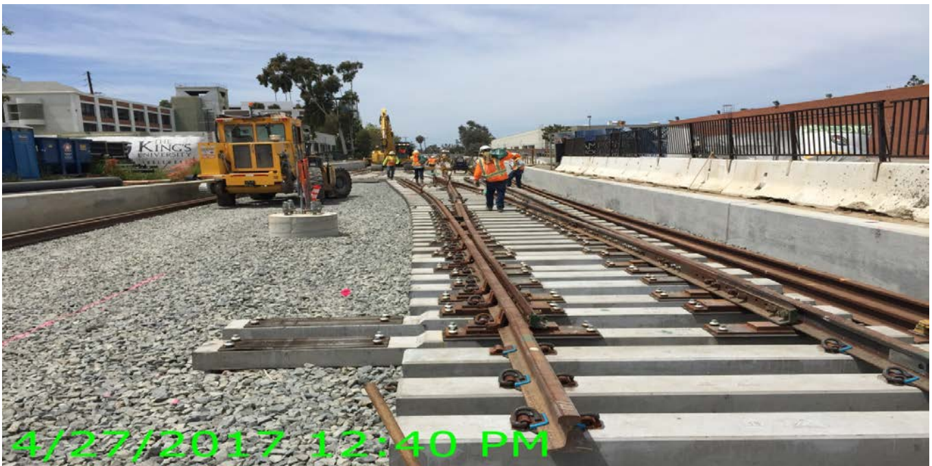
Special ballasted trackwork installation.
