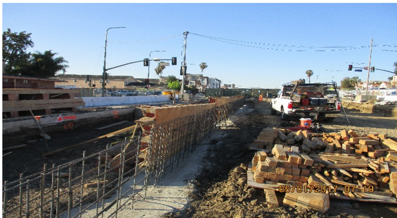
PARK MESA – Installation of formwork for ballast wall south of 50th St.
