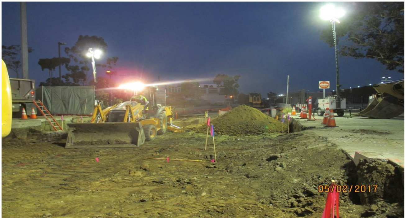
EUCALYPTUS GRADE CROSSING - AC paving of the approach and departure to match the existing elevation of Centinela Ave.
