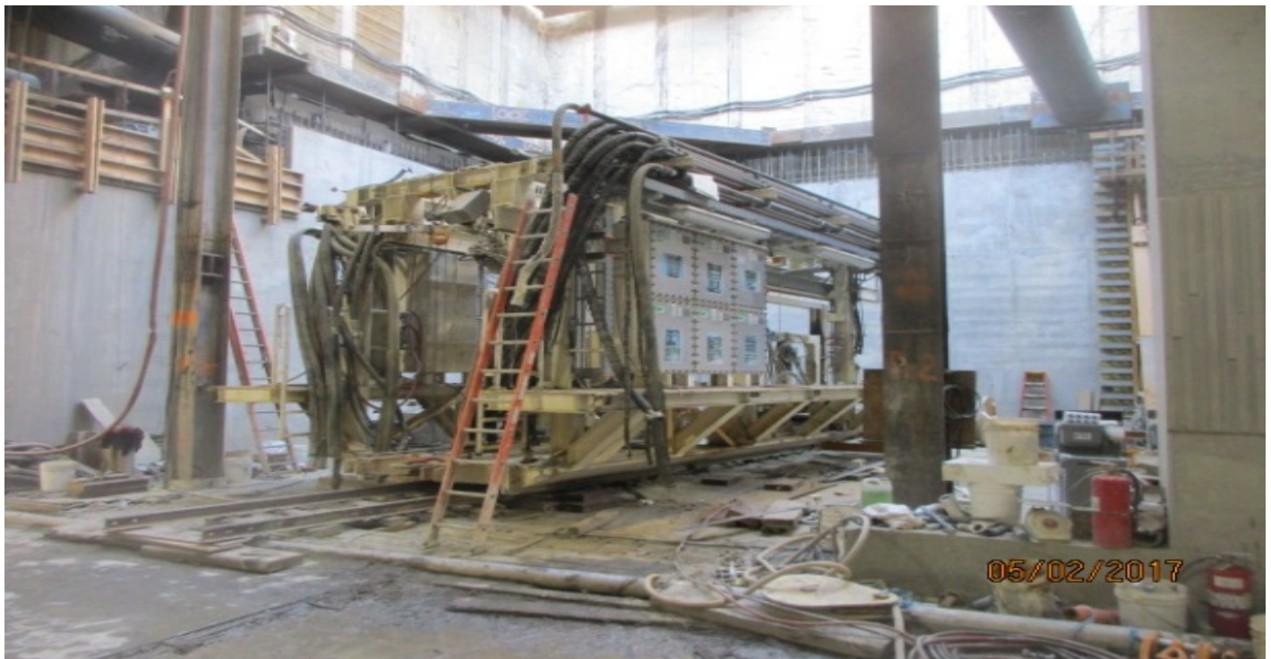
TUNNELING – Disassembling TBM trailing gear car #2 and preparing to hoist out of MLK Station.
