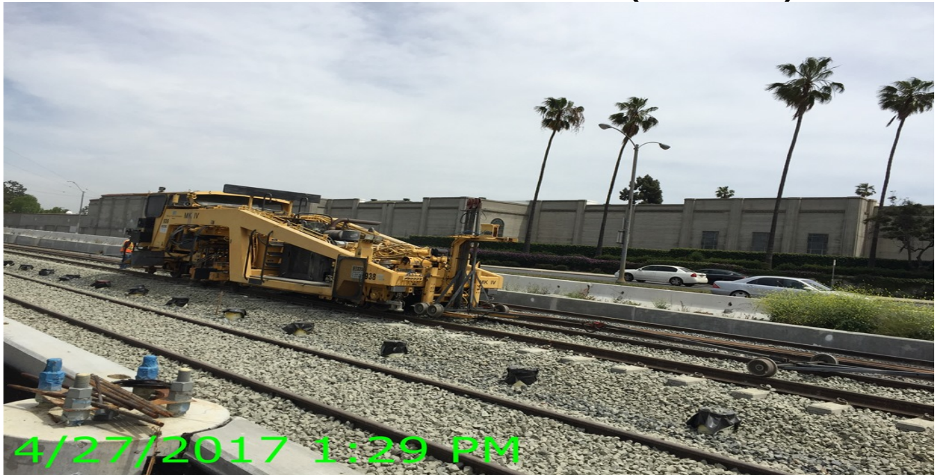
Ballast tamping ongoing.
