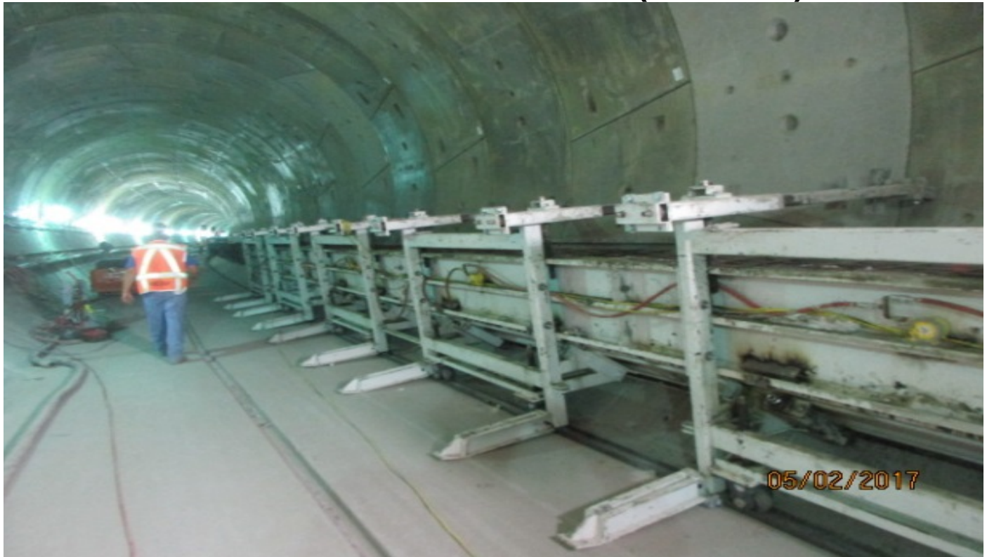
TUNNELING – Installation of SB Tunnel Walkway formwork.
