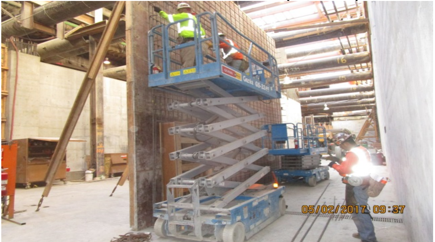
MARTIN LUTHER KING JR. STATION – Installation of formwork for interior wall section LW-28.
