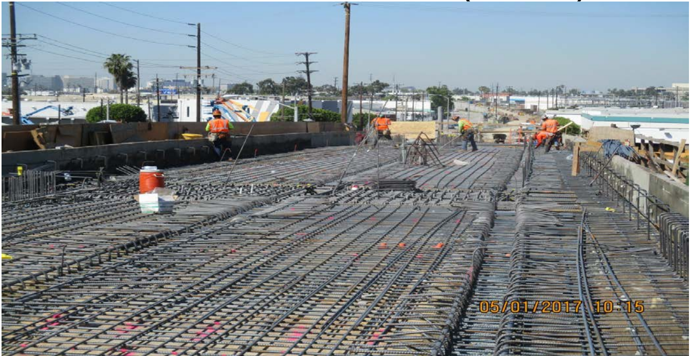
(AG-5) I-405 BRIDGE- Crews finished lost deck construction. Subcontractor IRP continued installing deck, overhang and parapet curb reinforcement. Deck pour tentatively scheduled for May 13th. (Span 1).
