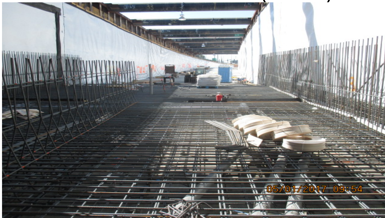
UG4 – Installation of rebar for invert section I-16.
