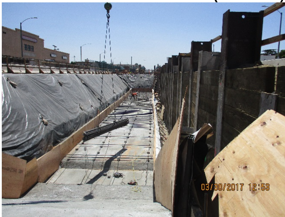
Hyde Park Station – Rebar installation for TC&C room invert slab.
