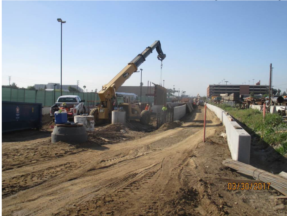
Contractor constructing the final remaining ballast walls for 96 th Street station accommodations effort.
