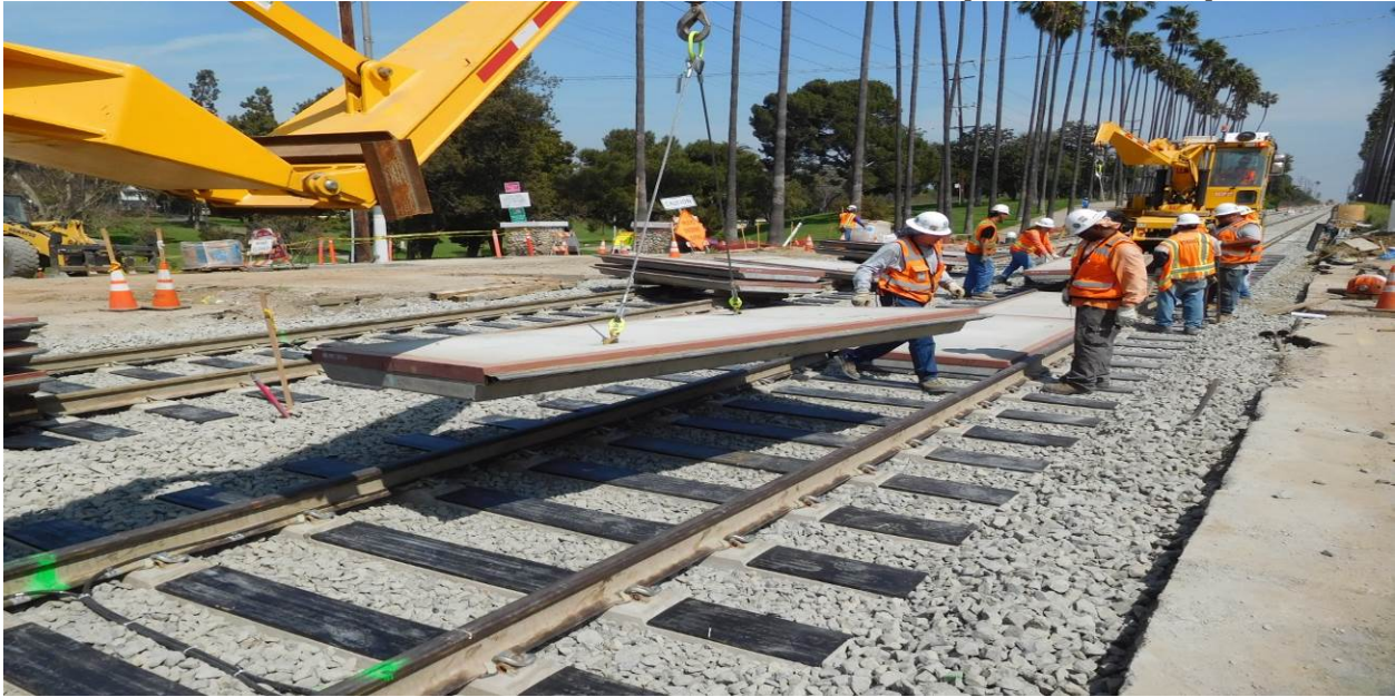
Centinela Avenue grade crossing - Crossing panel installation.
