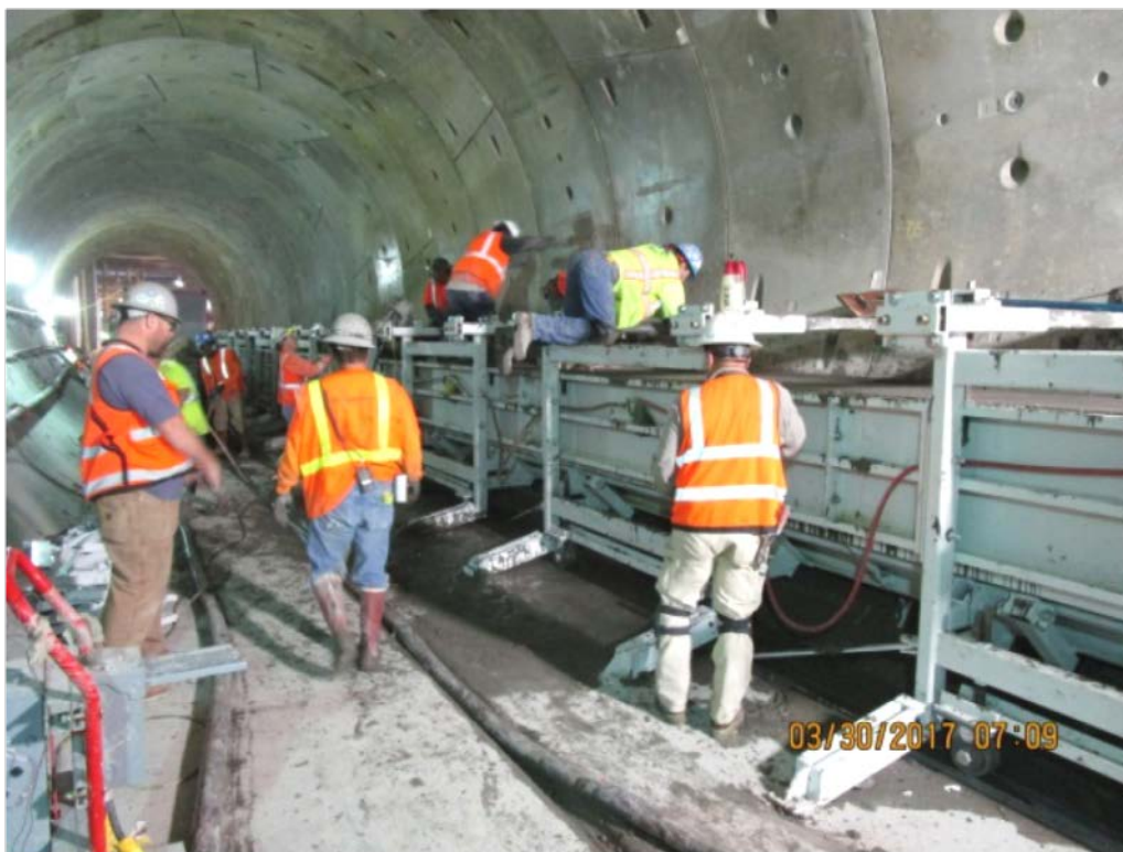
First Walkway placement in tunnel just south of MLK station – SB tunnel.
