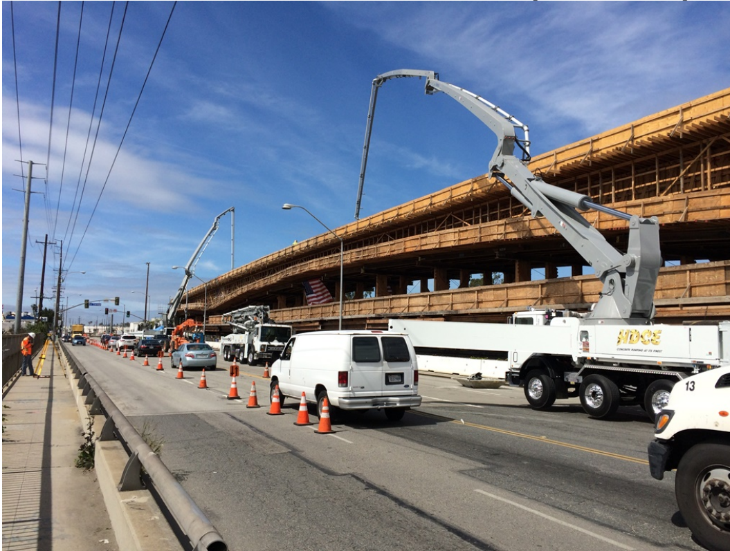
Contractor placing concrete for I-405 bridge span.
