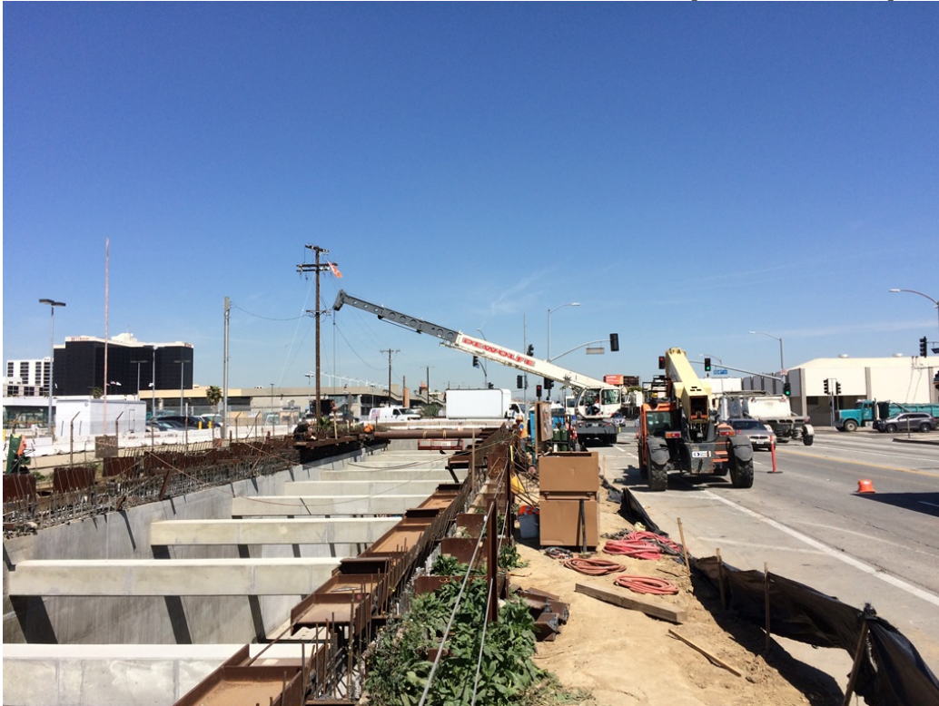
Tier 1 SOE strut removals nearly complete for tunnel in front of LAX runways.
