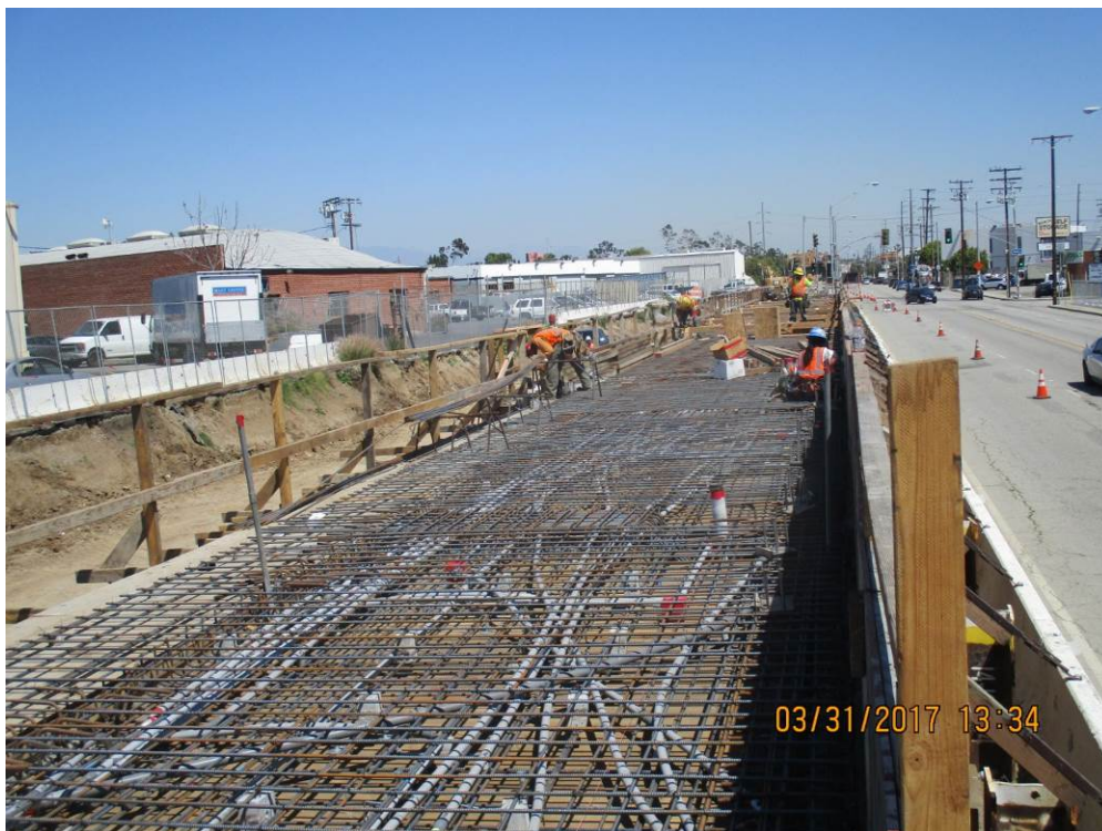
Deck reinforcement and conduit embed installations ongoing for Hindry Station NB platform (photo facing up-station).
