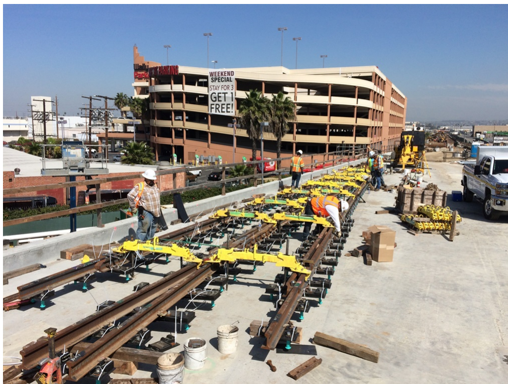
Iron horse assembly in preparation for top-down DF construction of the 10k and 10k1 crossovers.
