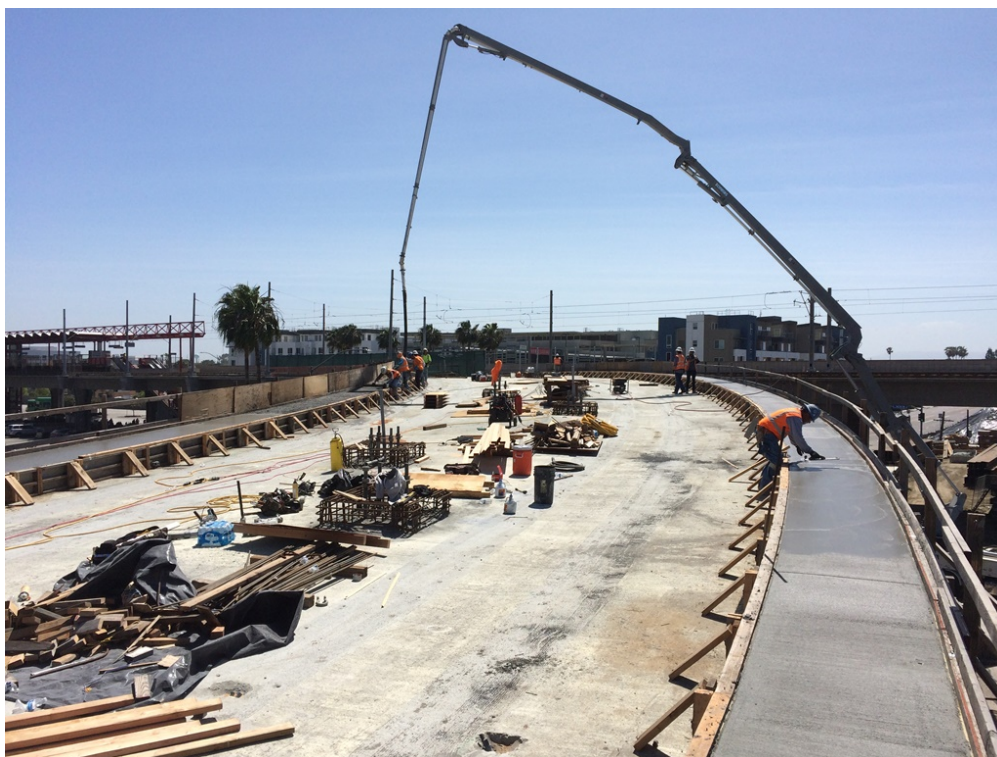
Contractor continues concrete placement for the multi-purpose emergency walkway/ductbank/parapet curbs for Green Line tie-in structure.
