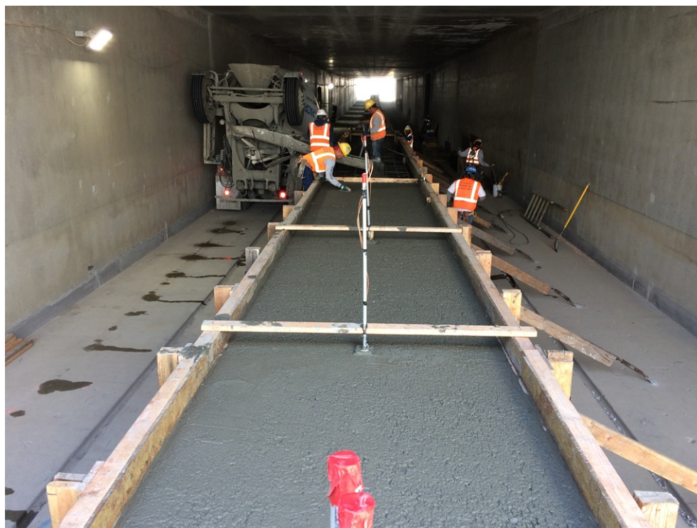
Contractor continues raised emergency walkway construction for tunnel in front of LAX runway.
