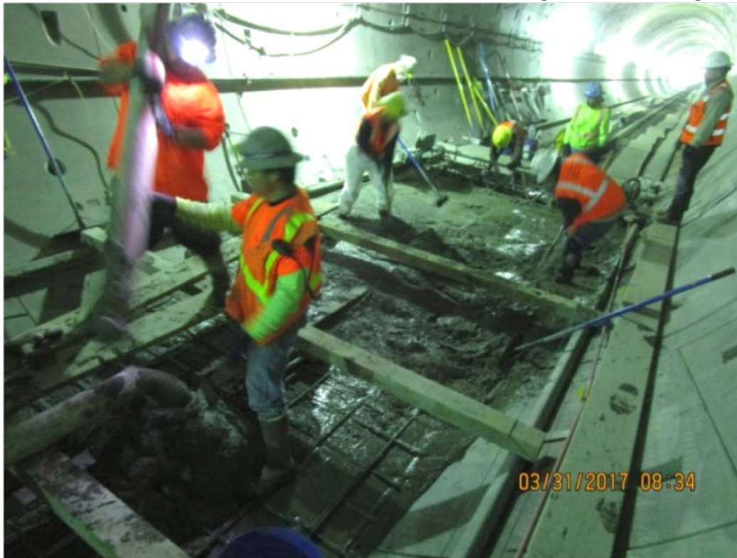
Placement of SB Tunnel invert.
