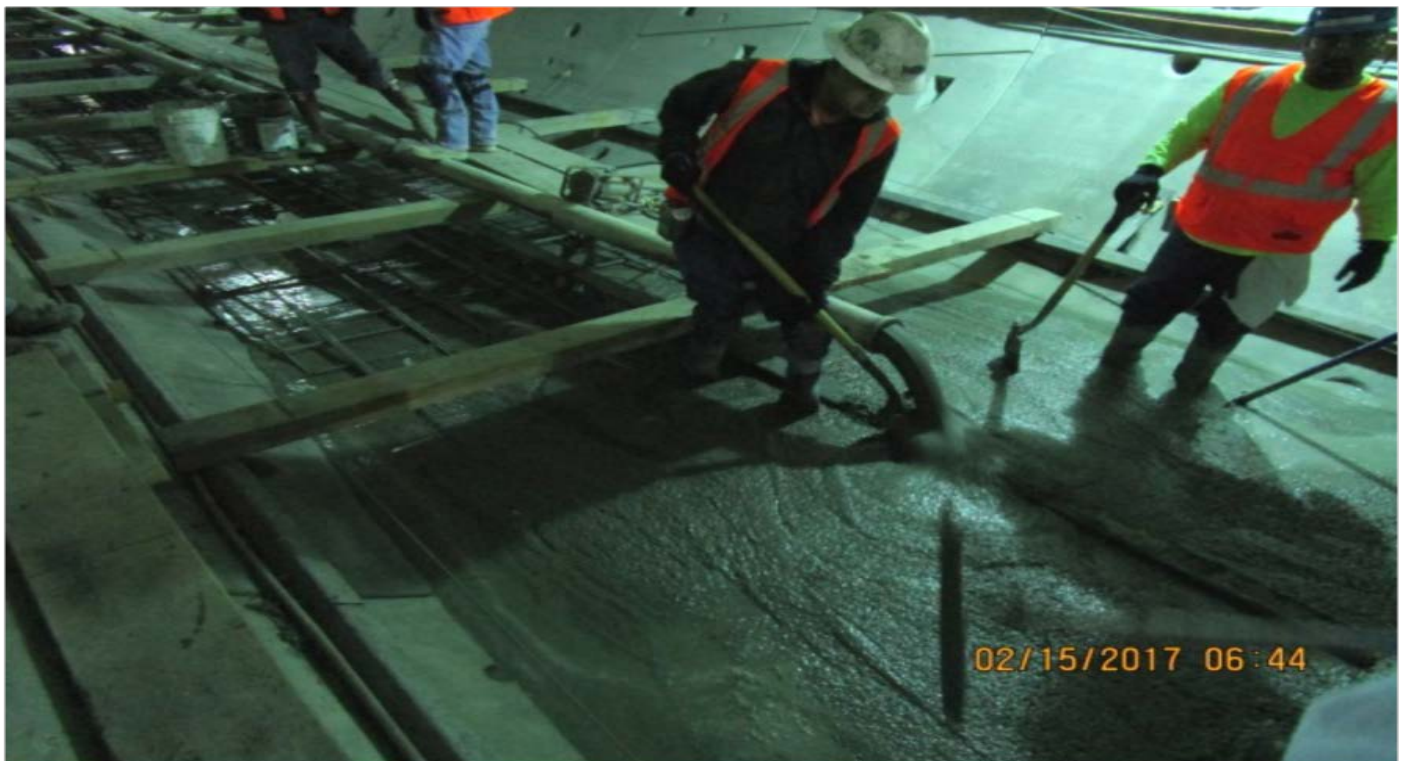
TUNNELING – Placement of SB Tunnel Invert section 11.
