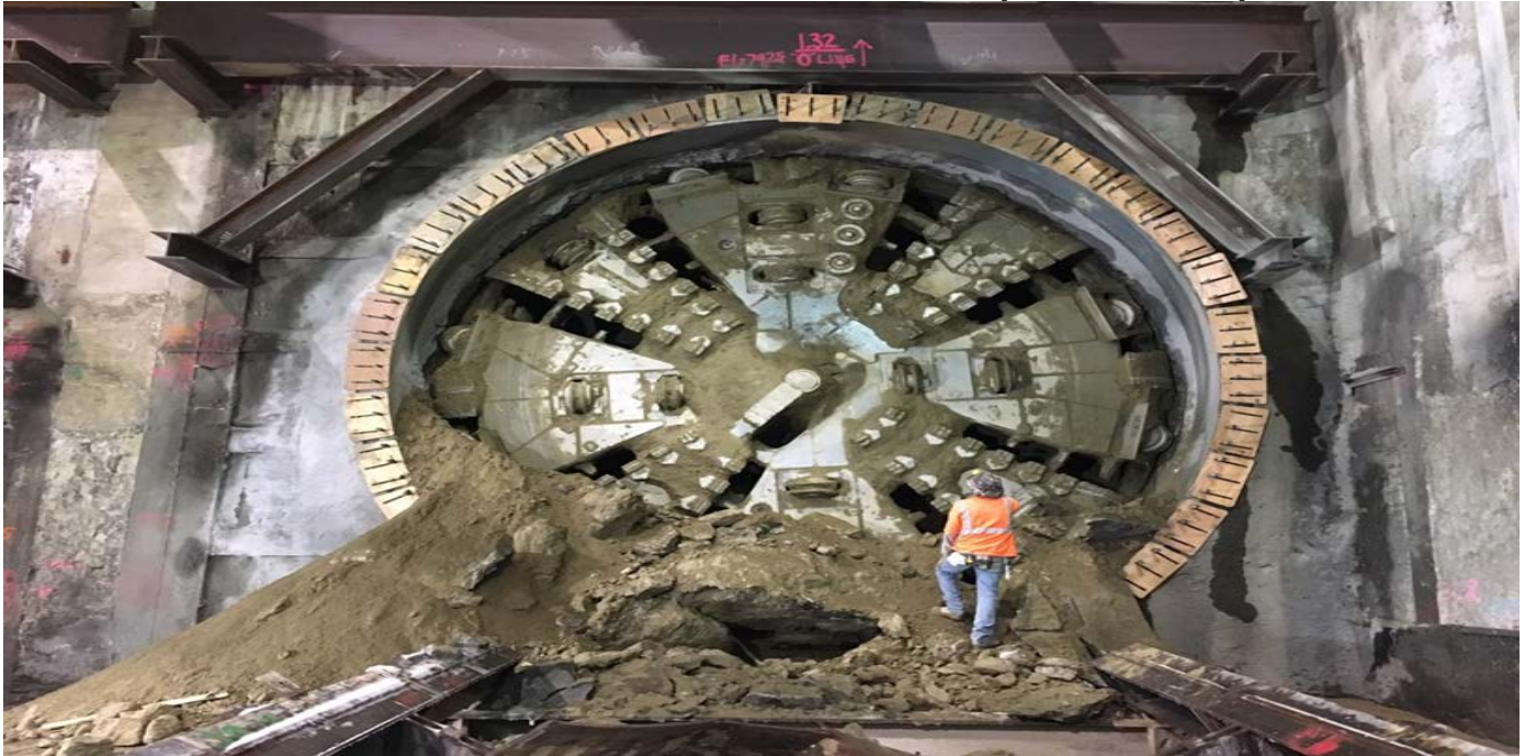
TUNNELING –TBM holed into MLK Station at 6:40 PM on Tuesday, 2/14/17.
