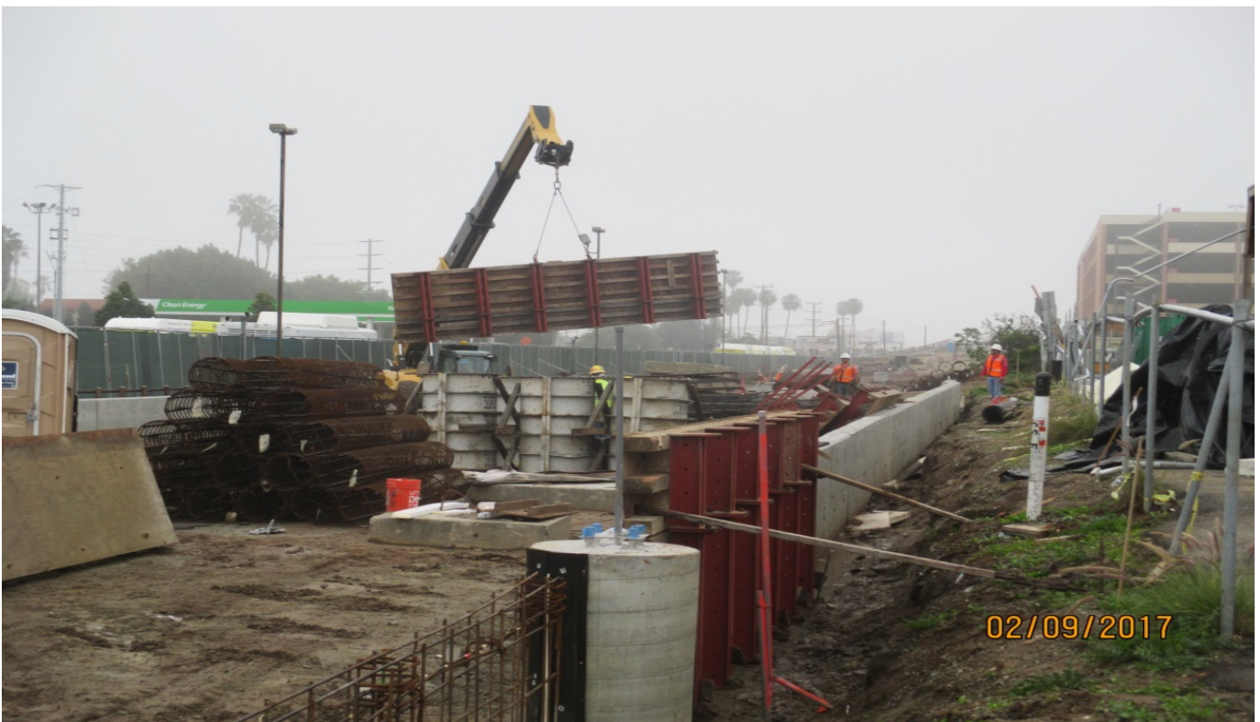
96 th STATION Accommodations – Crews continued constructing ballast retainer walls.
