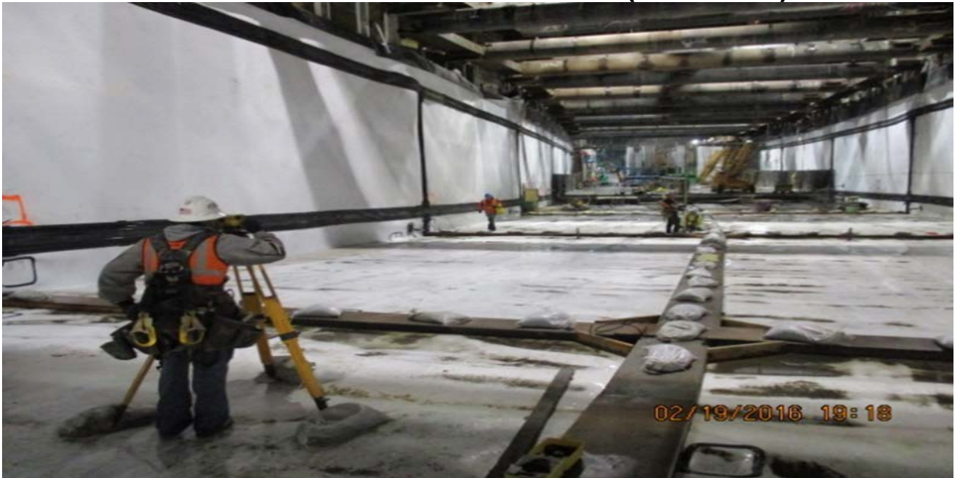
UG#4 – Waterproofing near Leimert Park Station.
