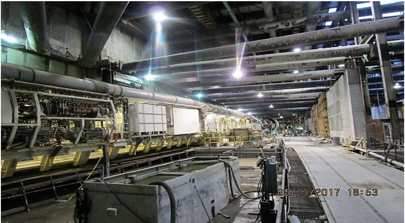
TUNNELING –TBM trailing gear being pulled thru MLK Jr. Station.
