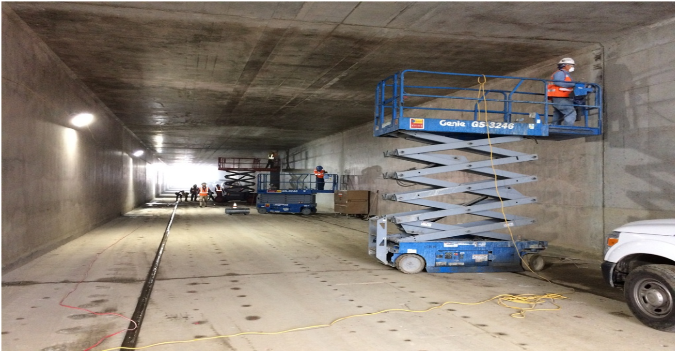
UG1 - Concrete finish work underway along the cut & cover tunnel segments.
