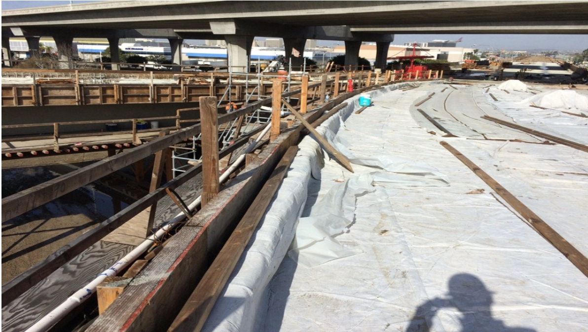
GREENLINE UNDERPASS – Frame 1: Deck concrete cure.
