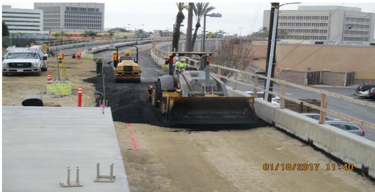
(AG-6) LA BREA BRIDGE –. Crews worked on placing the Asphalt cap.
