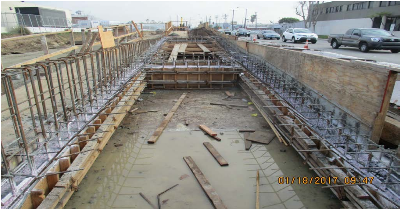
WESTCHESTER STATION – Concrete placement for the northbound platform's stem walls, shear walls and engaged columns.
