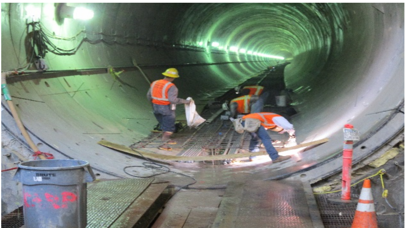
TUNNELING – Preparing SB Tunnel for invert.
