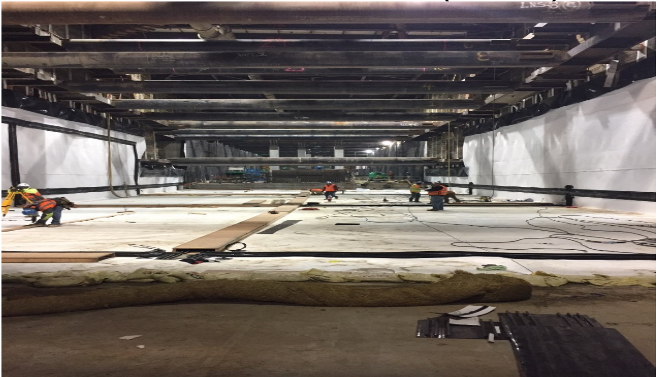
UG#4 – Installation of waterproofing and formwork for protection slab at north portal.
