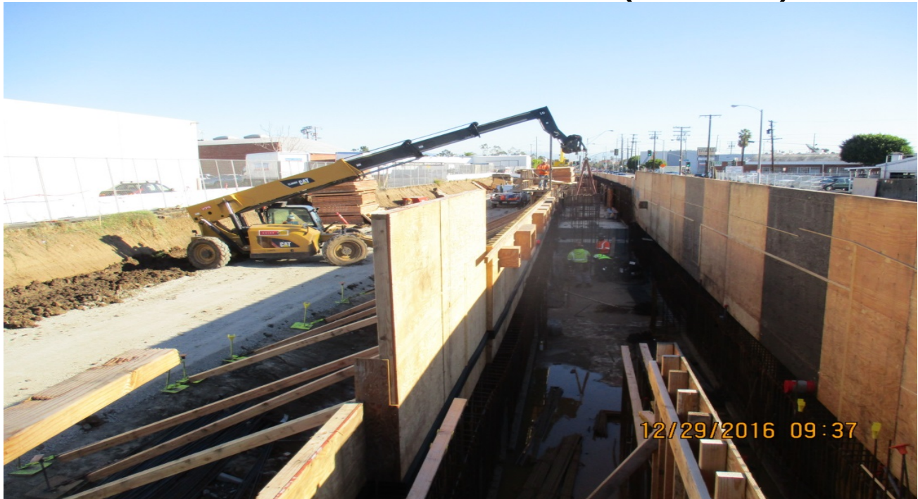
WESTCHESTER STATION – Rebar and formwork for Hindry station north bound platform stem walls.
