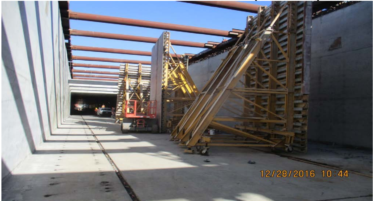
UG#1 – Crew continues with sequential construction at Underground Guide way progressing from South to North. Open cut at strutted U-wall.
