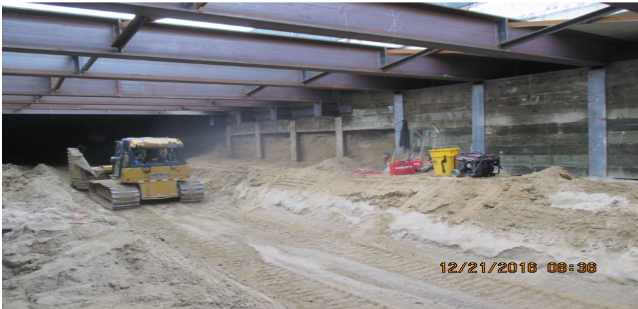
UG#3 – Lagging and excavation activities at 63rd St. UG#3 - Trenching activities for OCS conduits at north portal.
