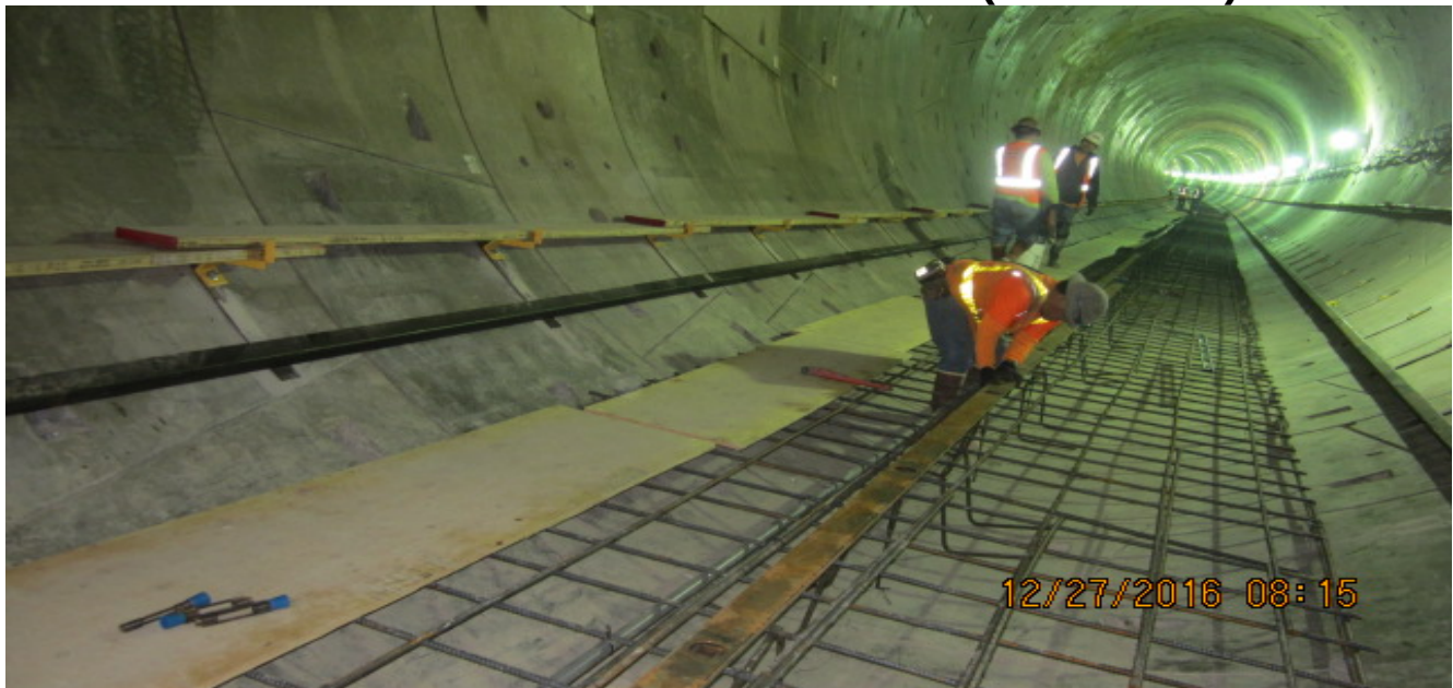
TUNNELING – Installation of gutter drain formwork at SB tunnel to accommodate tunnel invert work.
