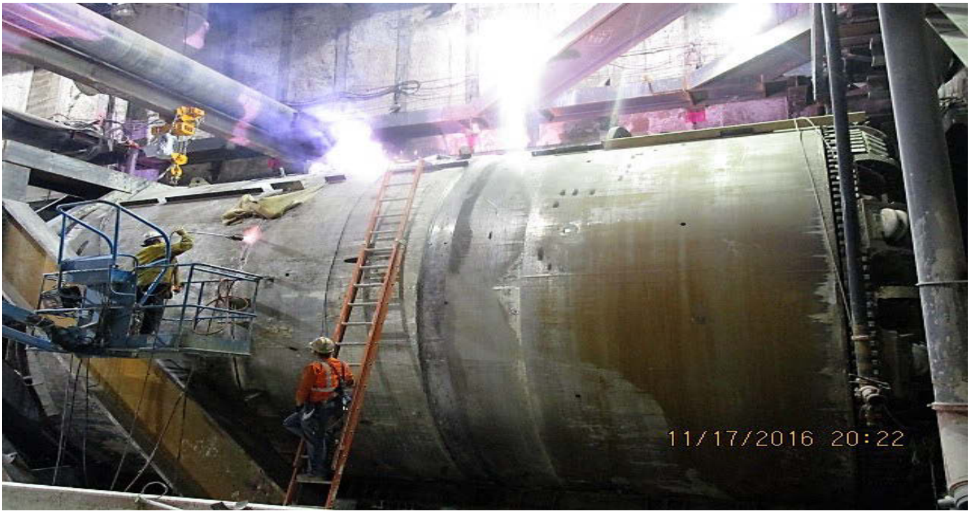
TUNNELING – Welding of the TBM mid-shield/tail shield joint at NB tunnel portal.
