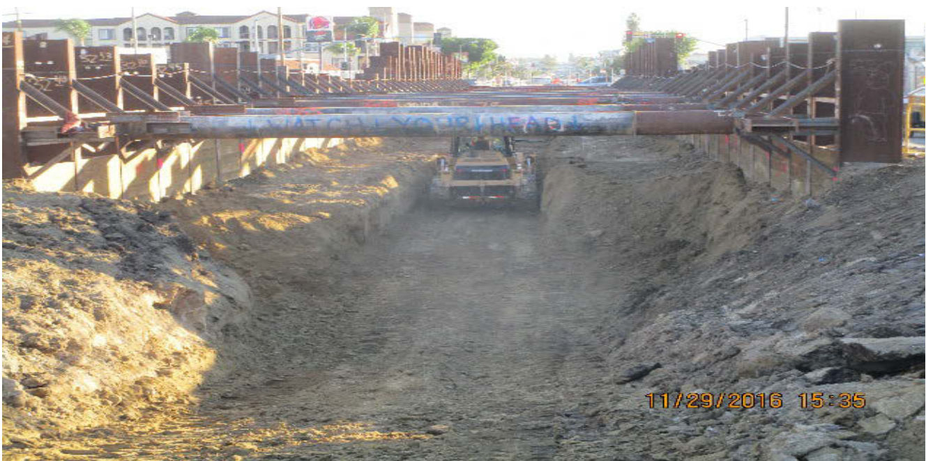
UG#3- Excavating beneath struts at north portal.
