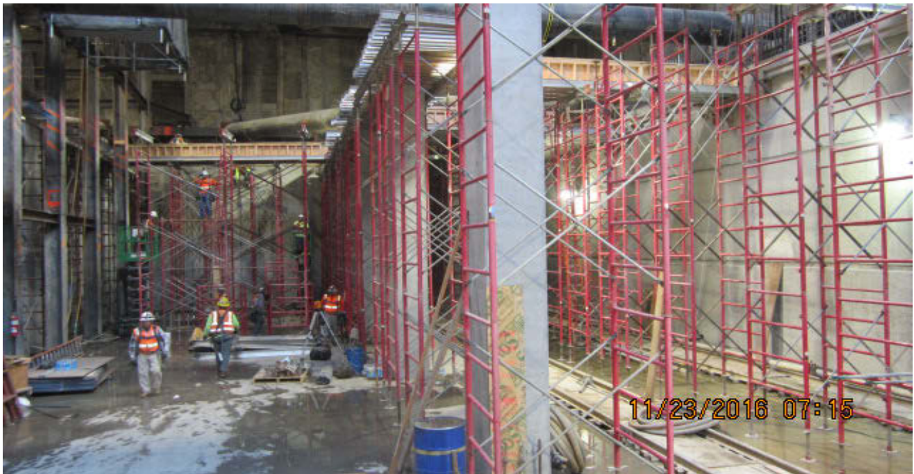
EXPOSITION/CRENSHAW STATION – Installation of shoring components for concourse slab falsework.
