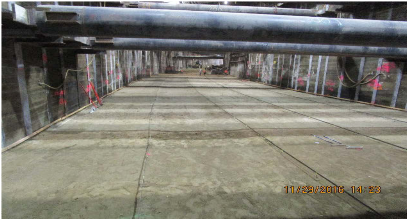
UG#4 – Preparing grade for mud slab placement at north end of UG4.
