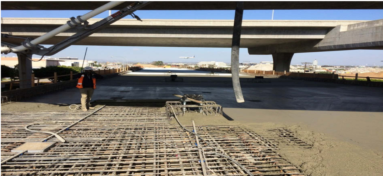
GREENLINE UNDERPASS – Frame 2: Deck concrete placement.
