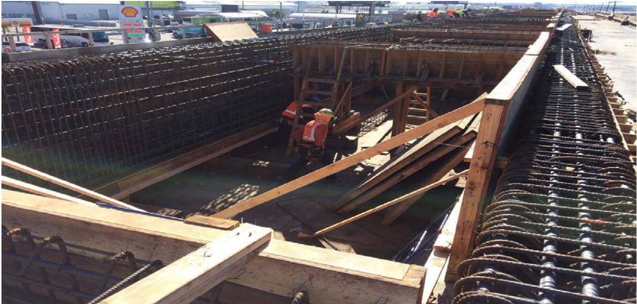
AVIATION/CENTURY BRIDGE – Formwork and rebar installations ongoing for the girders and beams of the aerial station platform.
