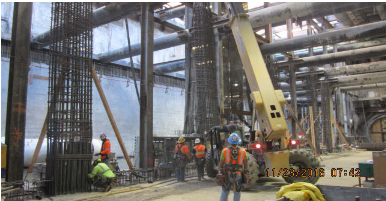
MARTIN LUTHER KING JR. STATION – Installation of rebar for invert columns.
